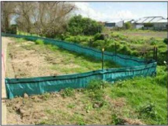
EXAMPLE OF SEDIMENT FENCING WITH RETURNS
