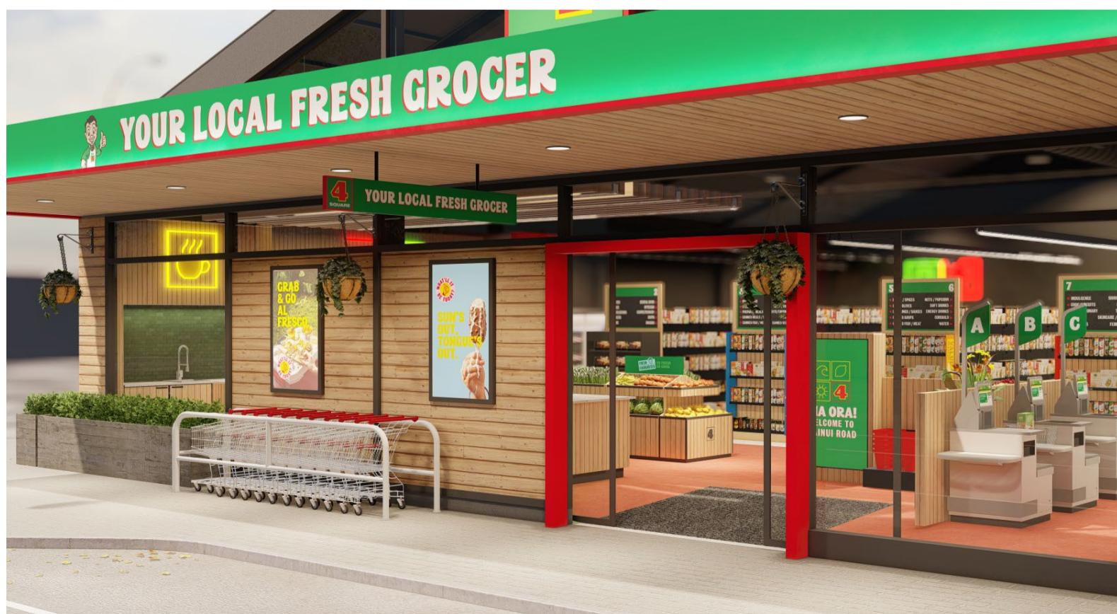
Typical Building Four & Fascia Tagline Signs Implementation
