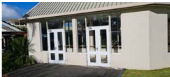
3 EXISTING LINK BUILDING PHOTO NOT TO SCALE
