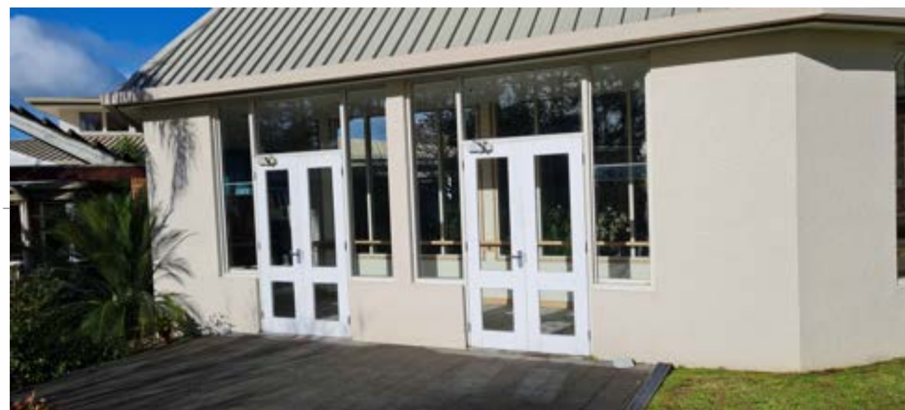
EXISTING LINK BUILDING PHOTO
