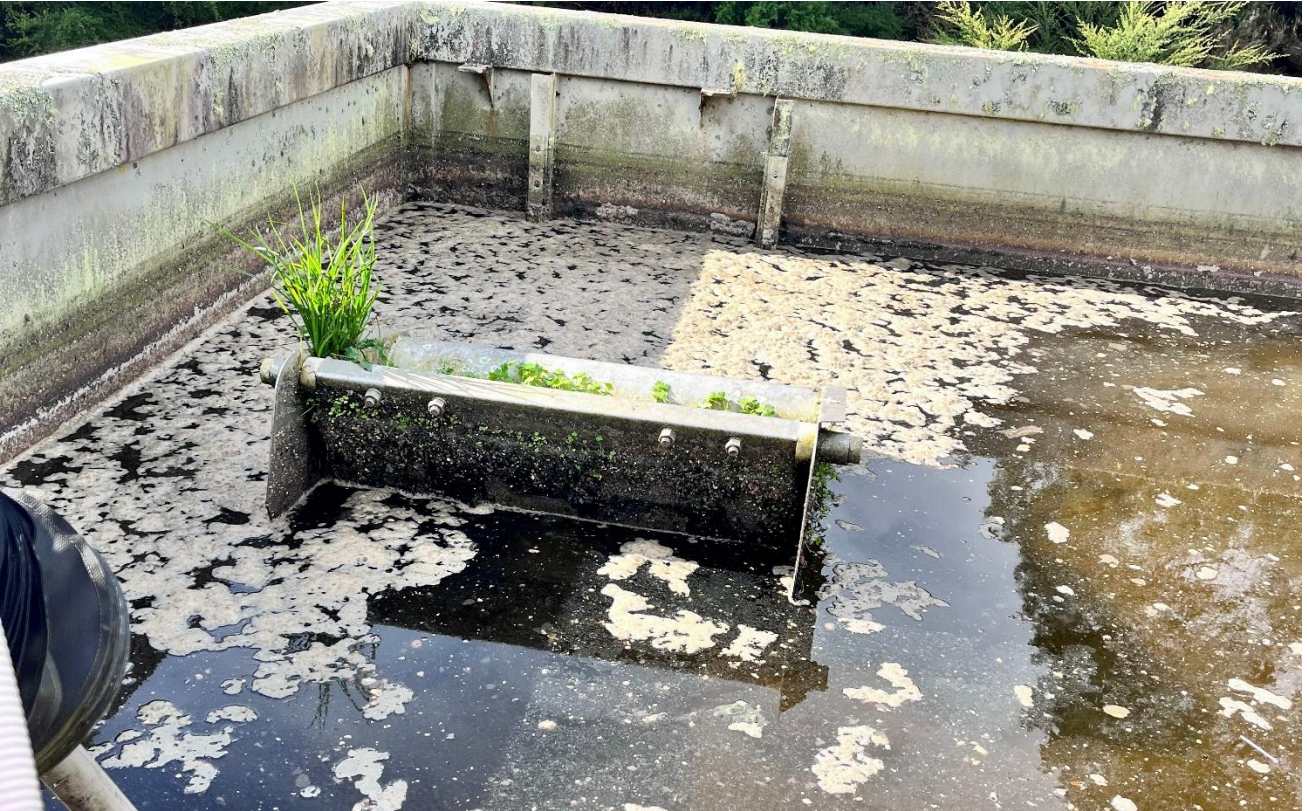
Figure 9 : Decanter SBR Reactor 1
