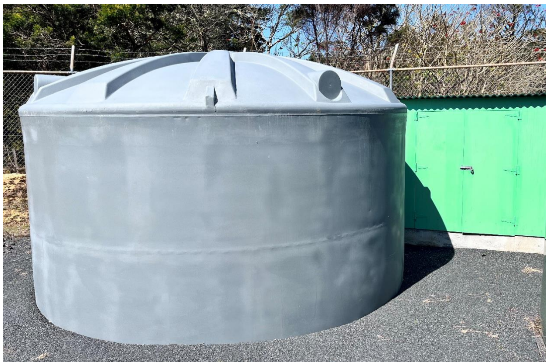
Figure 17 : Backwash water supply tank (left) and Backwash supply pump house (right)
