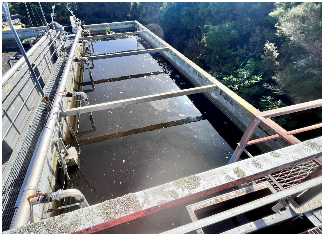
Figure 6 : SBR Reactor 1
