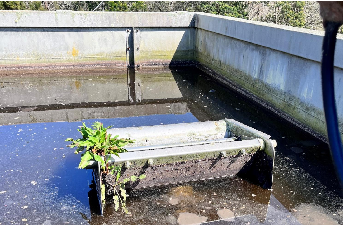
Figure 10 : Decanter SBR Reactor 2
