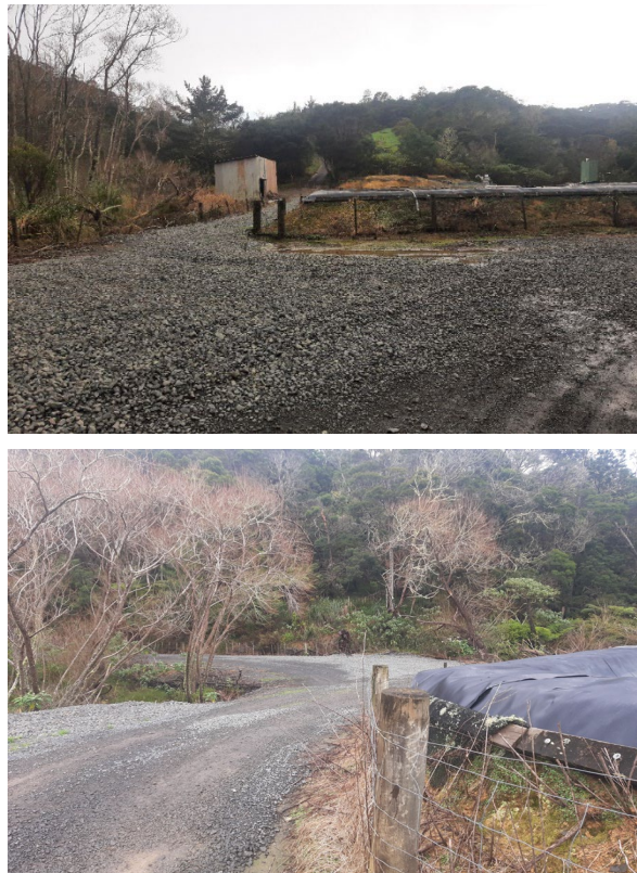
Figure 4: Photos of constructed pond bunds at KR-WWTP (photos taken 6th Sept 2023)
