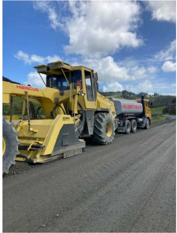
Figure 6: Peria Road Seal Extension Section 5 Stabilising
