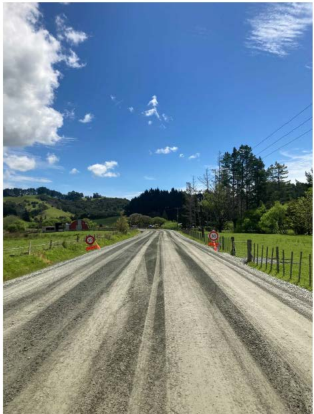
Figure 8: Peria Rd Seal Extension Section 5 Seal Prep
