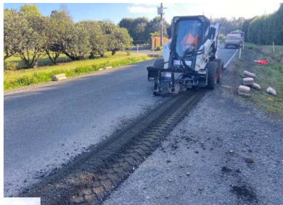
Stanners Rd – Bobcat Pre hoeing before Stabilising
