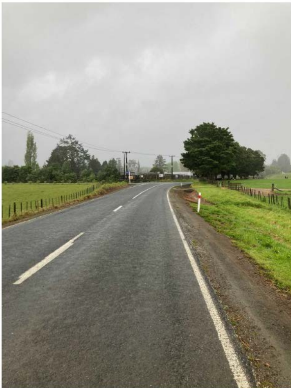
Figure 11: Oruru Rd Pre-reseal Watertabling
