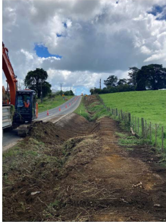
Figure 17: Oruru Rd Rehab 1 Enabling works
