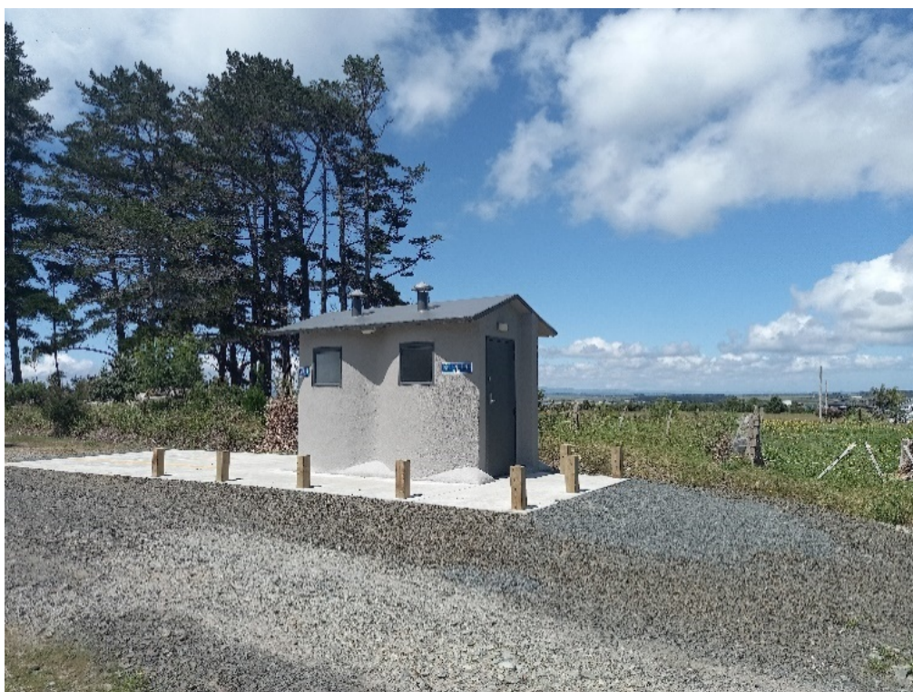
Whatuwhiwhi - new toilet block
