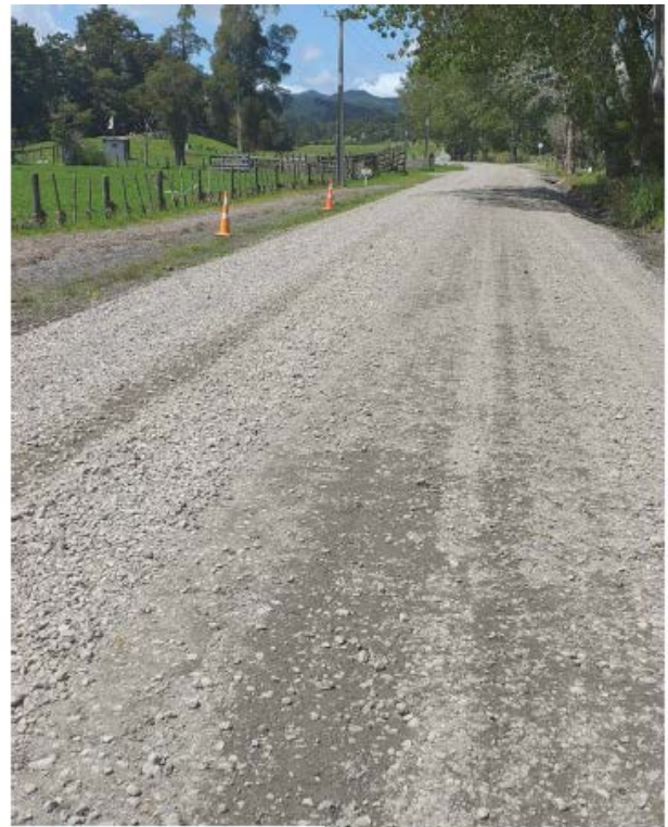
Before/After - Horeke Rd – Heavy rain event Respread followed by rip and remake.
