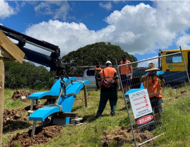
Procrete installing the bird seats
