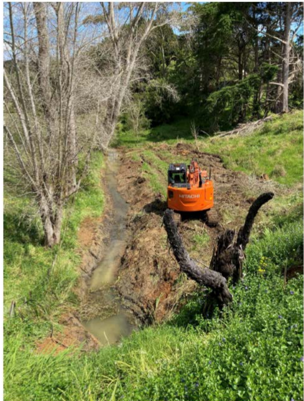
Figure 16: Oruru Rd Rehab 1 Enabling works
