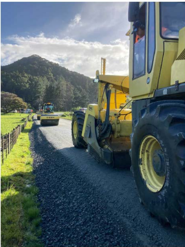
Figure 7: Peria Rd Seal Extension Section 5 Stabilising
