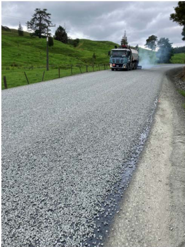
Figure 15: Pawarenga Rd Rehab Sealing
