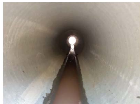
Bolero Road - Culvert Replacement
