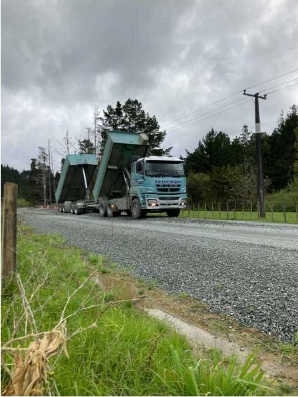
Figure 5: Peria Rd Seal Extension Section 5 Overlay
