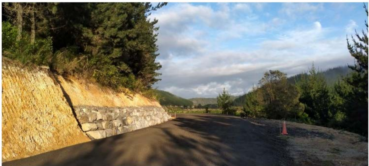
Ngapipito Rd – Above – New Seal, Below – Rock lined batter
