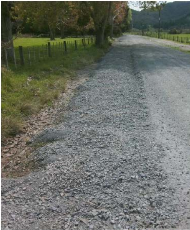
Before/After - Horeke Rd – Heavy rain event Respread followed by rip and remake.
