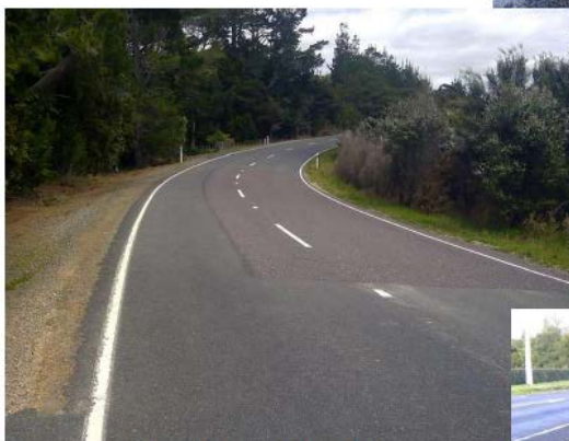
Aucks Rd – After picture – Stabilised pre seal patch
