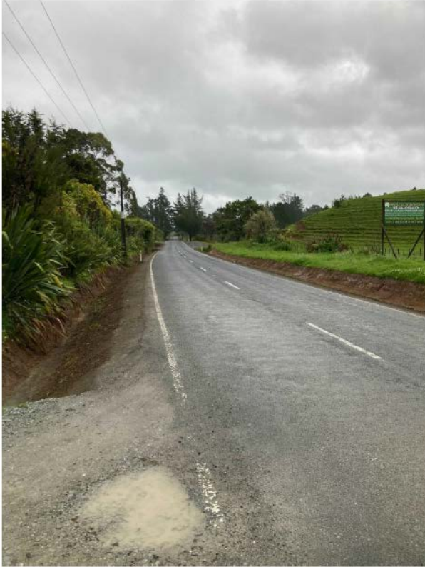
Figure 13: Oruru Rd Pre-reseal Watertabling
