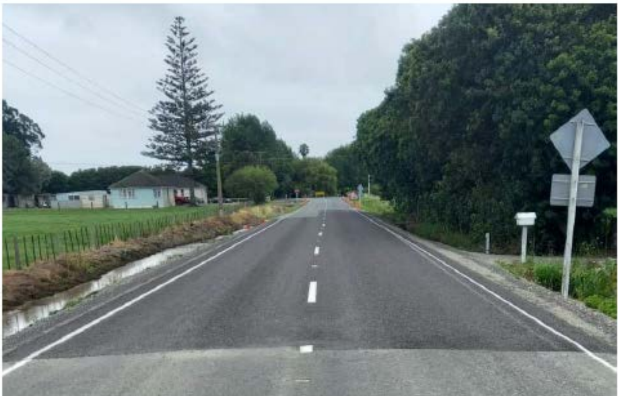
Unahi Rd – Awanui – Sealed Patch
