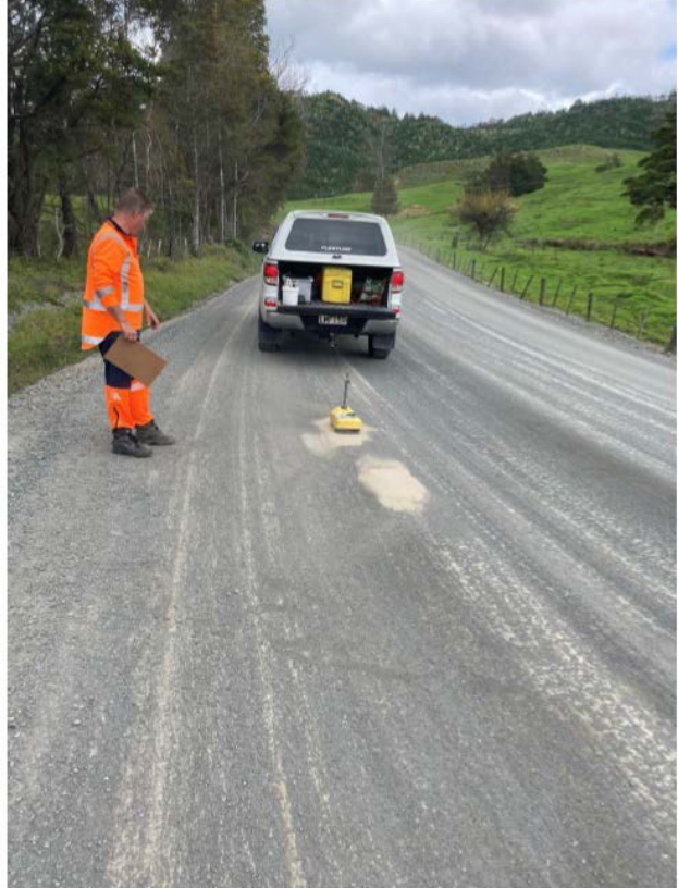
Figure 14: Pawarenga Rd Rehab Testing
