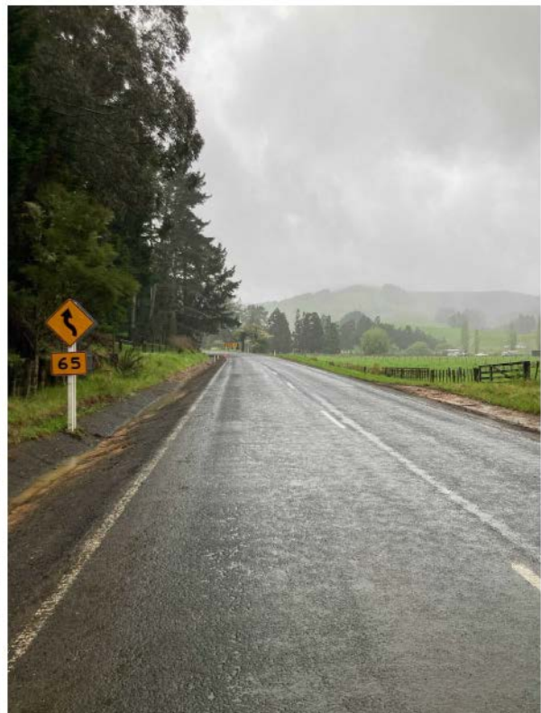
Figure 12: Oruru Rd Pre-reseal Watertabling
