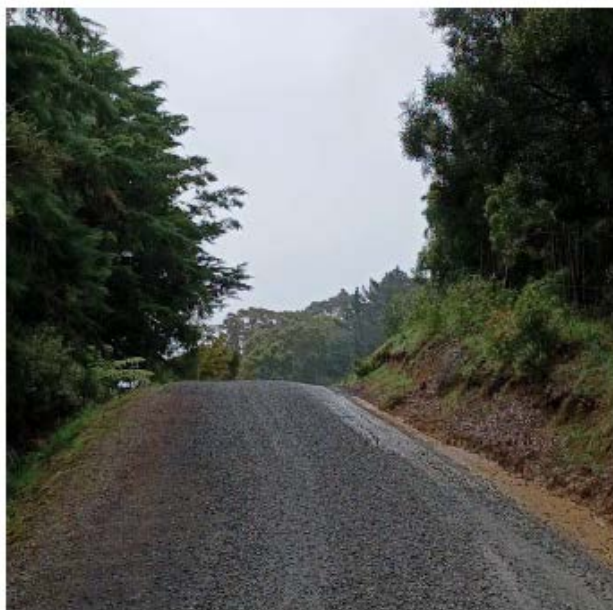
Ohuri Rd – Maintenance Metalling
