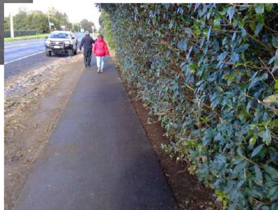
Kerikeri Inlet Rd – Footpath vegetation trimming
