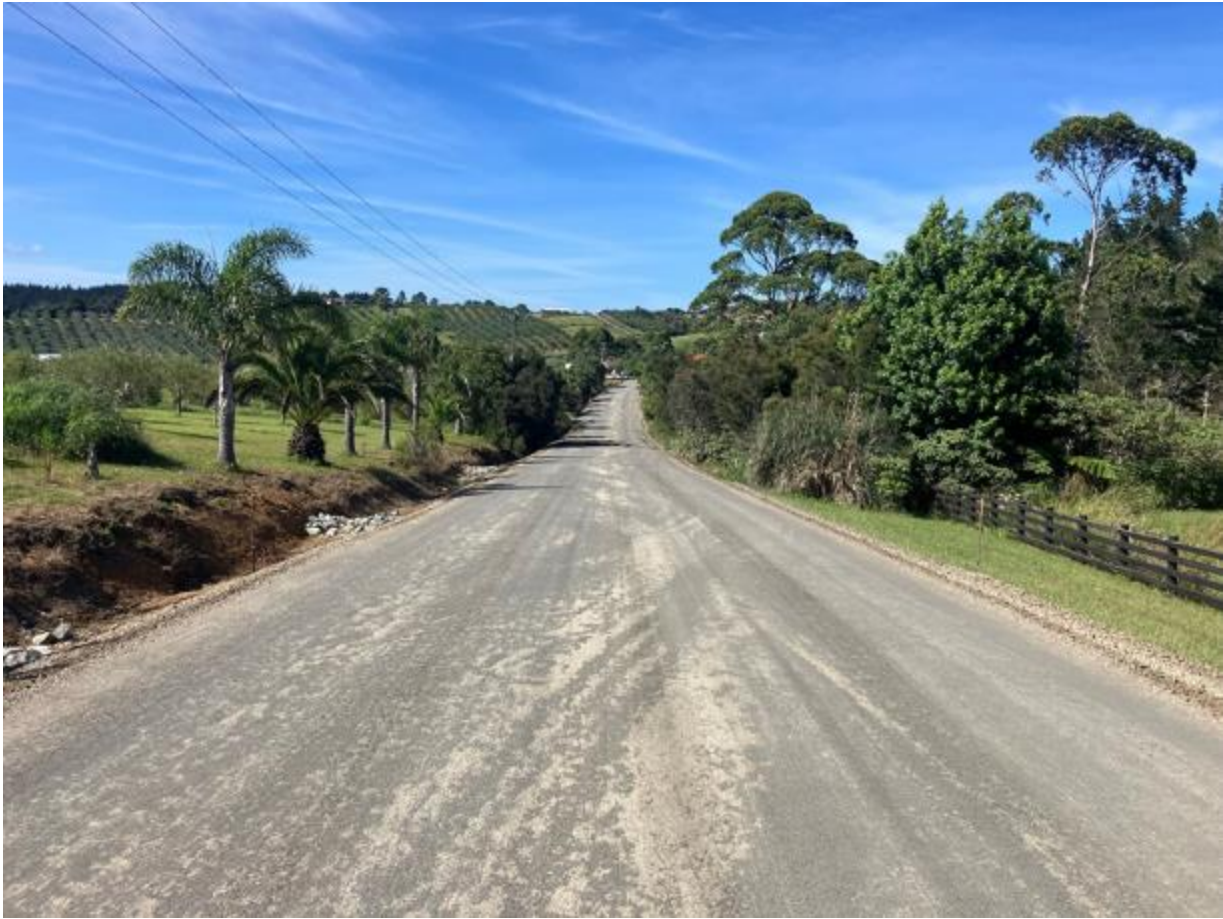
Midgeley Road Pavement Rehab ready for seal
