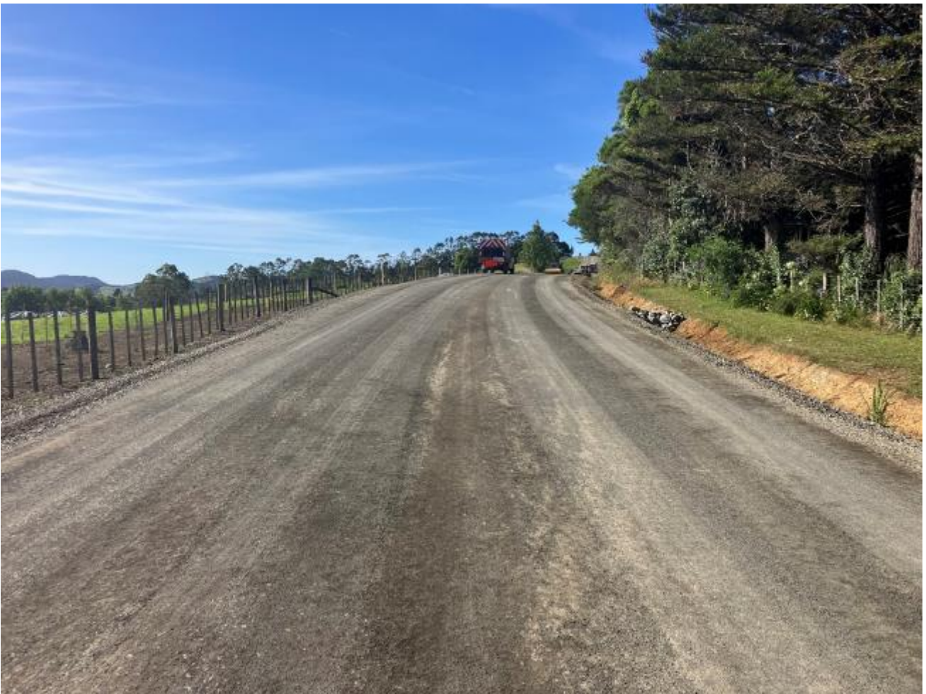
Midgeley Road Pavement Rehabilitation ready for seal
