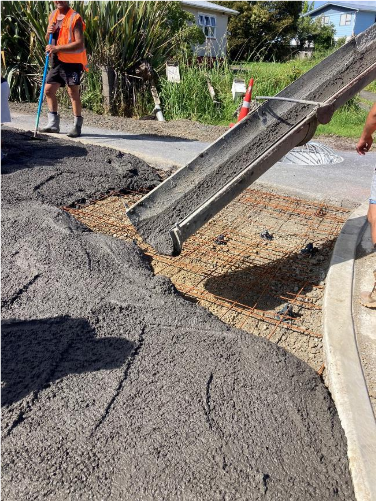
Sommerville Ave Pavement Rehab Driveway Construction
