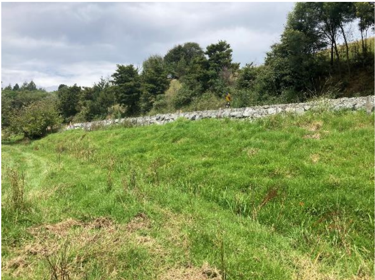
Fairburn Road Storm Damage Repair
