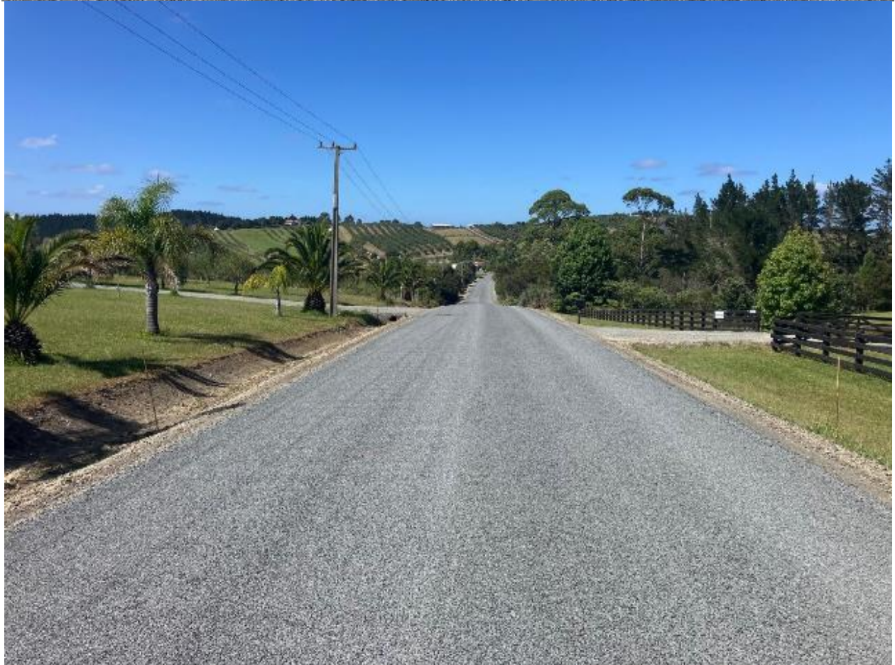
Midgeley Rd Pavement Rehab New Seal
