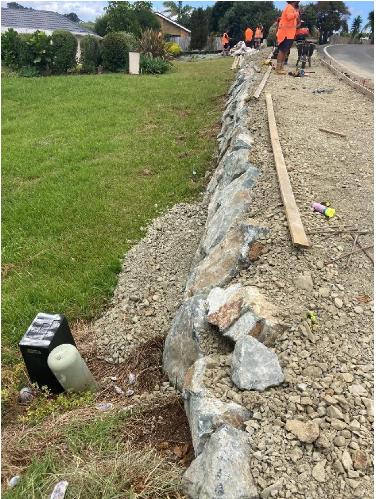
Cable Bay Block Rd New Footpath Prep
