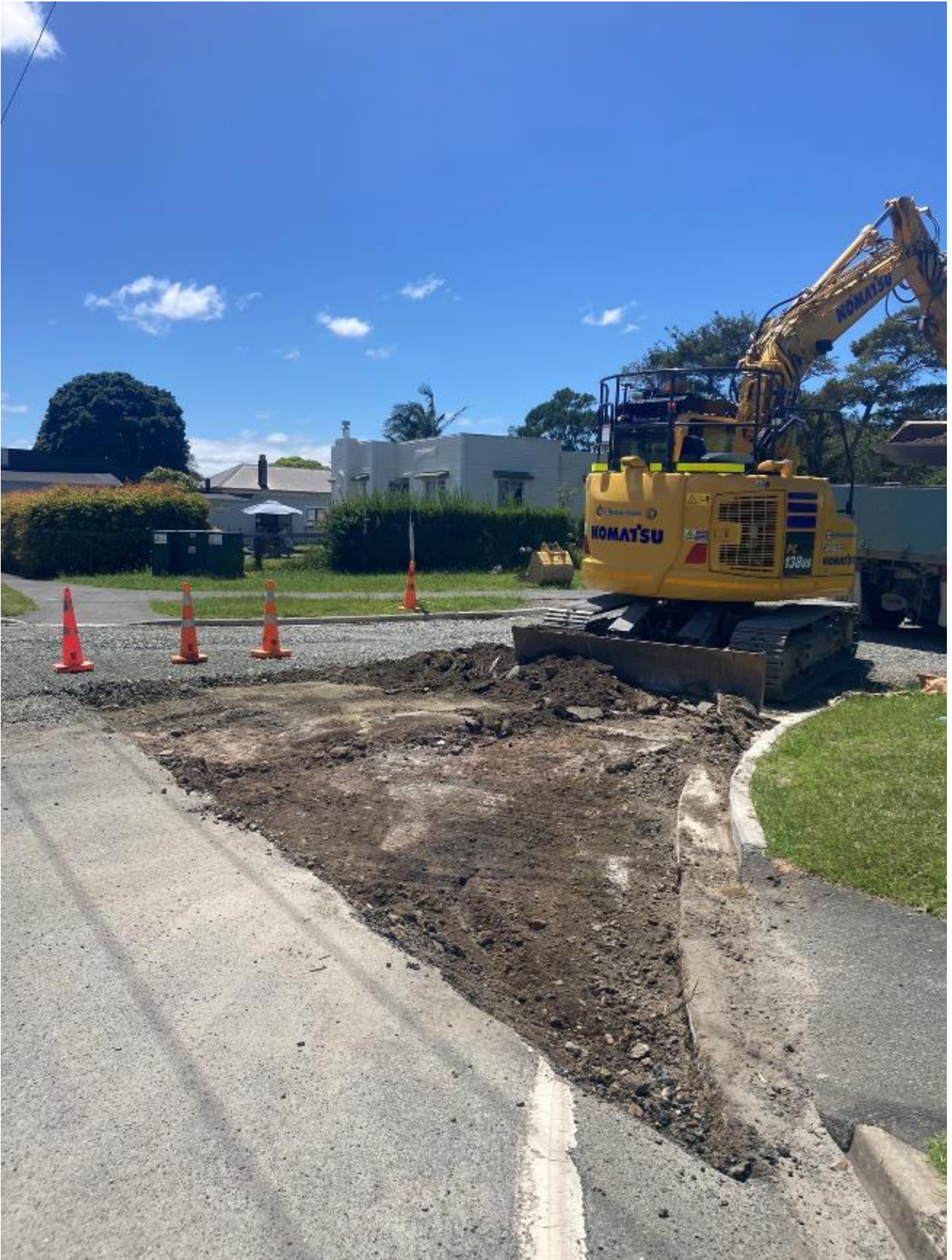
Sommerville Ave Pavement Rehab Undercut
