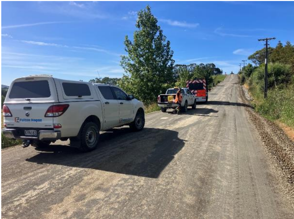
Midgeley Road Pavement Rehab NDM Testing Prior to Seal
