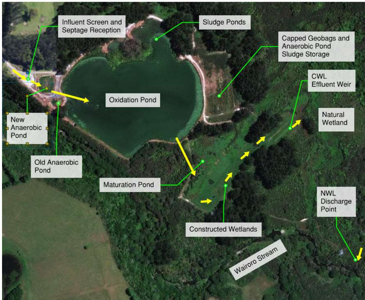
Figure 3: Kaikohe WWTP Overview (Image sourced from ArcGIS® software by Esri).
