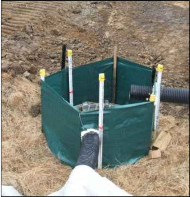
SILT FENCE AROUND CATCHPIT - DETAIL
