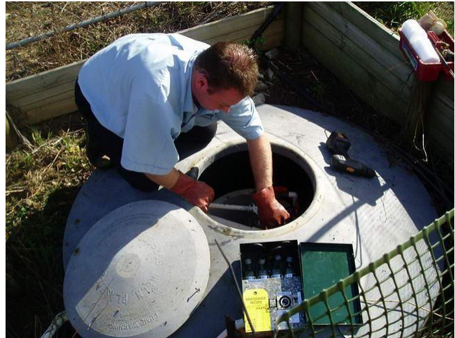
Servicing an advanced wastewater treatment unit
