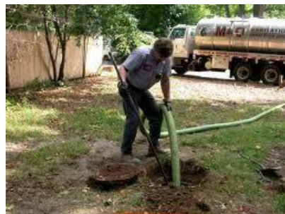
Septic tank pumpout
