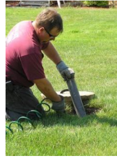
Lifting and hosing down effluent outlet filter
