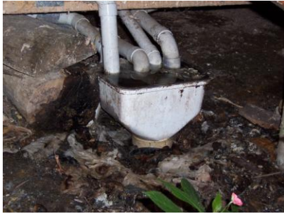
Backup to gully trap from clogged tank
