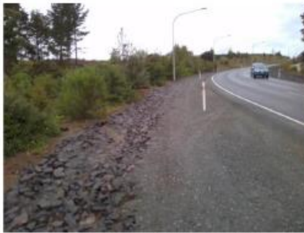
Puna Rere Dr Water-table Restoration
