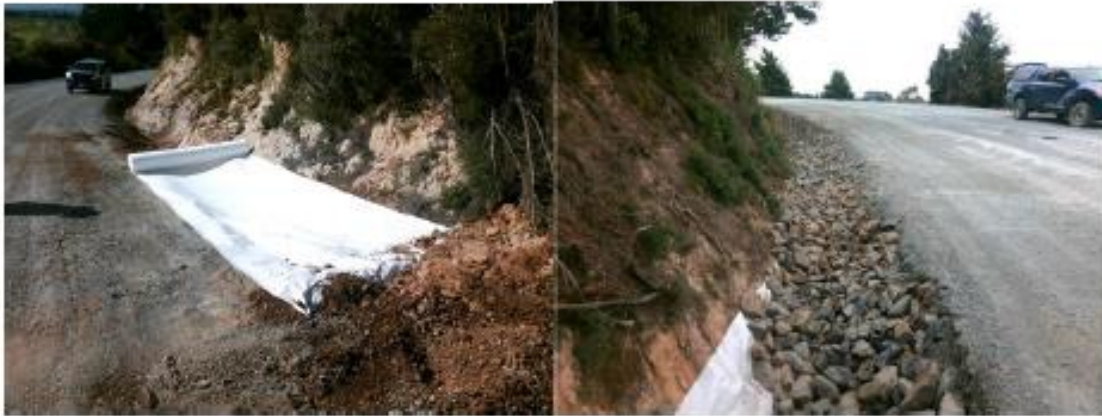
Mine Rd Stage 1 Water table reconstruction
