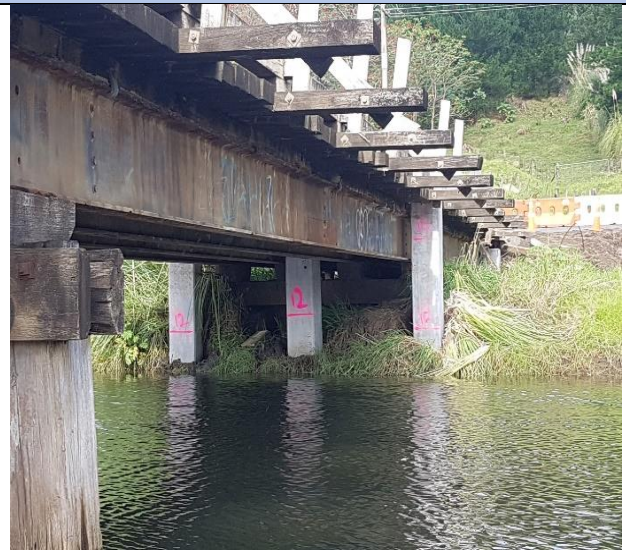
West Coast Road/ New piles in ground
