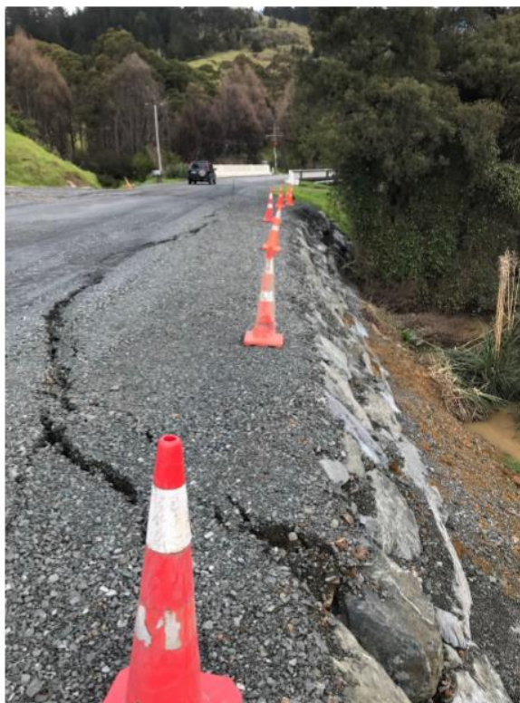
Figure 2: Section Five Underslip
