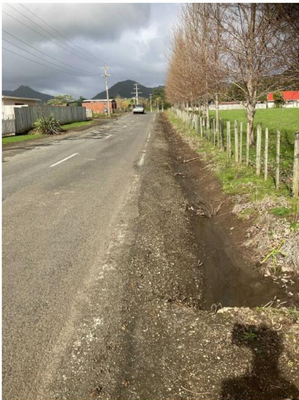
Figure 8: Roma Rd Pre Reseal Watertabling
