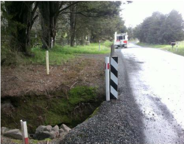
Waimatenui-Mataraua Rd – Bridge end marker replaced
