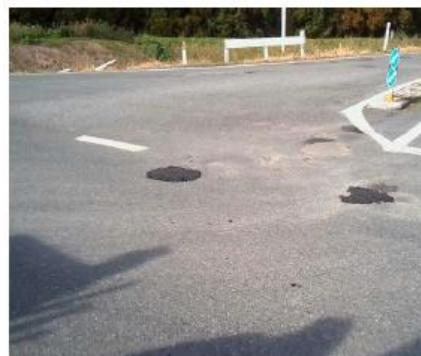
Waiare Rd – Pothole Repairs
