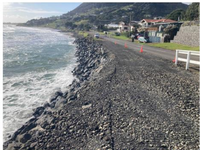
Figure 5: Foreshore Rd Seawall Repair / Footpath Prep
