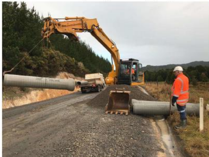
Ngapipito Rd – Culvert Installation along with a bit of on-the-job dumpy level training by Tony
