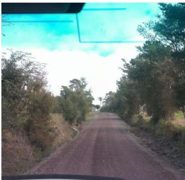
Pakaru Rd – Maintenance Metalling
