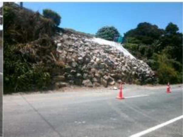
Whangarei Heads Rd Stormwater control
