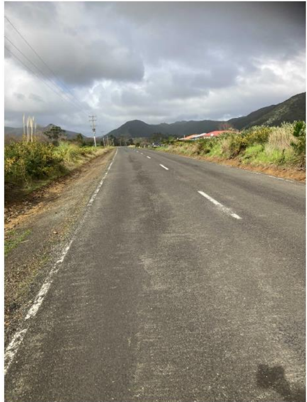
Figure 7: Roma Rd Pre Reseal Watertabling
