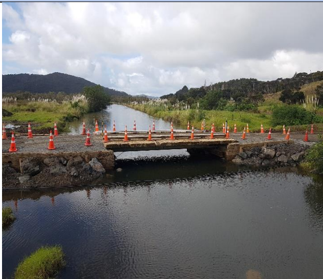
West Coast Road/Temporary bridge
