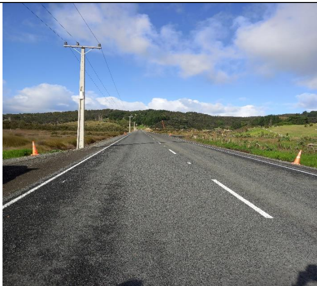
Panguru Road/Section C – Pavement raising & resurfacing completed
