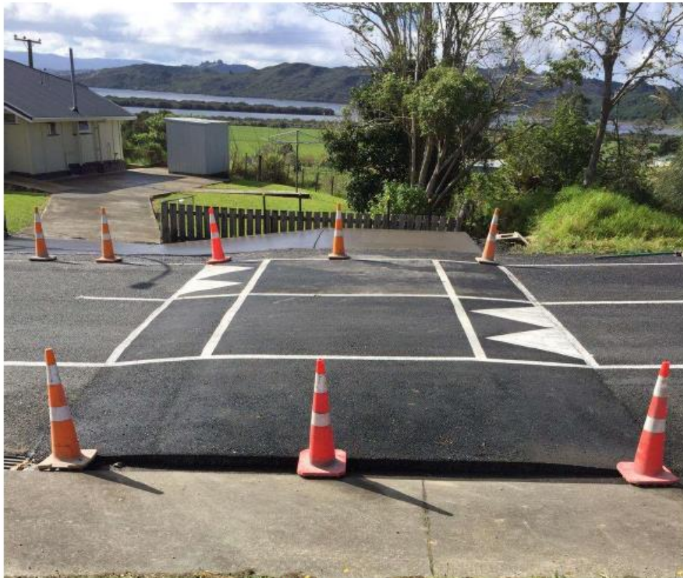
Parnell St, Rawene – Speed Table installation
