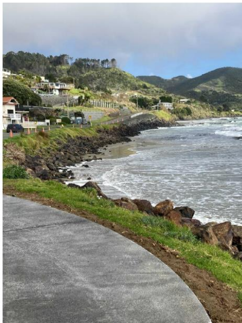
Figure 4: Foreshore Rd Seawall Repair / Footpath Build
