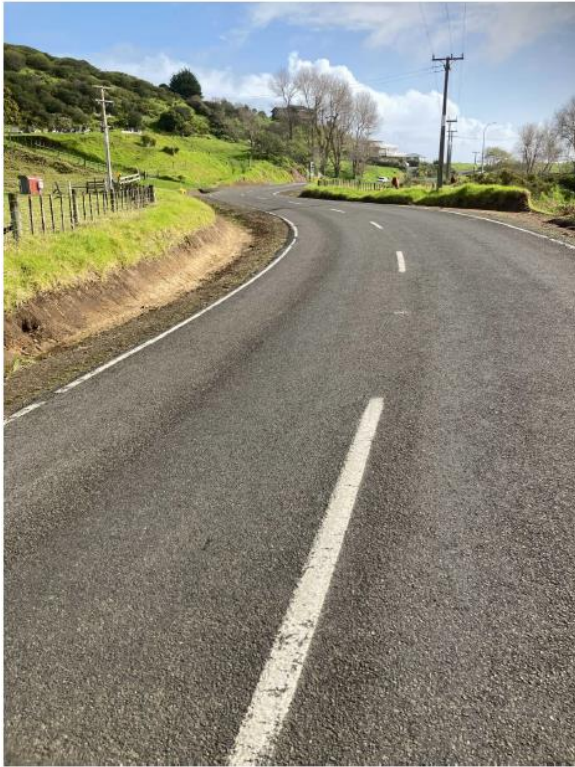
Figure 6: Roma Rd Pre Reseal Watertabling
