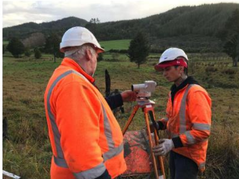
Ngapipito Rd – Culvert Installation along with a bit of on-the-job dumpy level training by Tony
