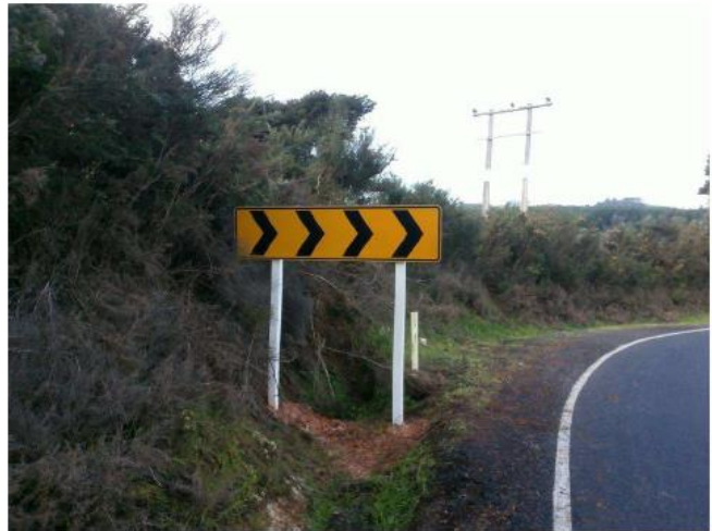
Kerikeri Inlet Rd – New PW66 installed on new posts following vandalism
