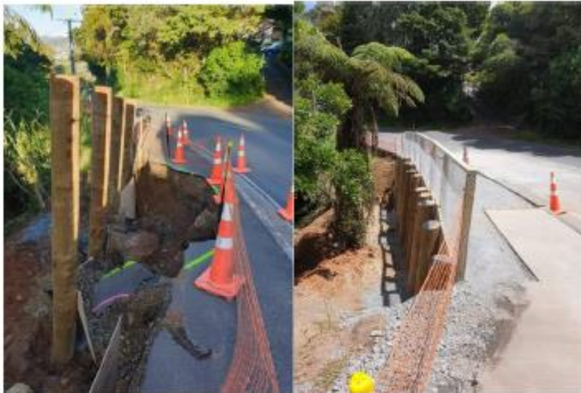
Memorial Dr Footpath Retaining wall
