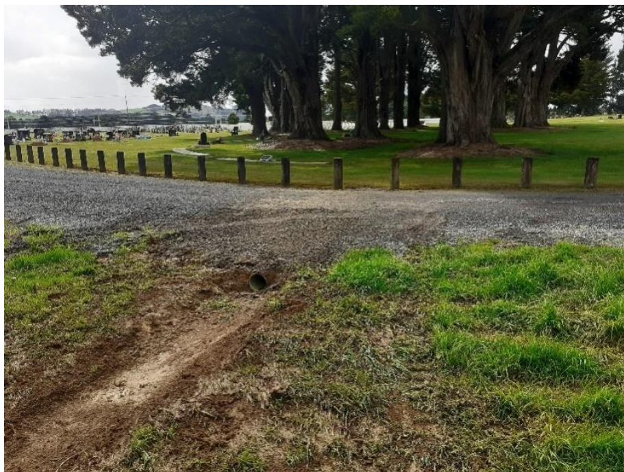
Stormwater improvements, Kaikohe cemetery
