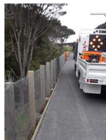
SH11 (Haruru) – Fencing damage repairs
