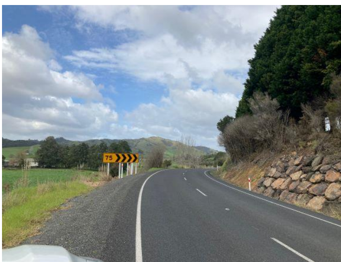
Fairburns and Oruru Road - Kaitaia Safety improvements
