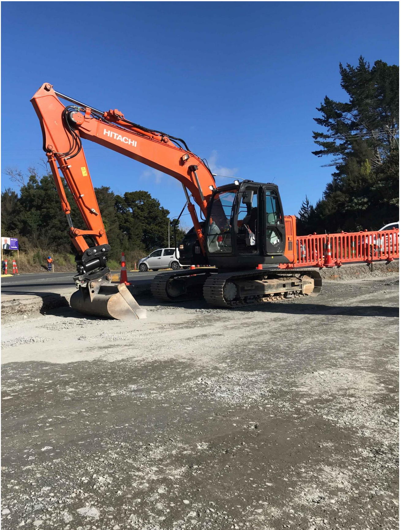
200903_1: Excavation of the temporary intersection corner/shoulder to build the temporary road.
