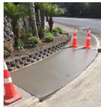
Blue Marlin Dr – Pram Crossing Replacement
