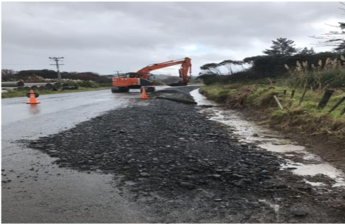
West Coast Road, Panguru Flood Mitigation/ Road Widening and Drainage work
