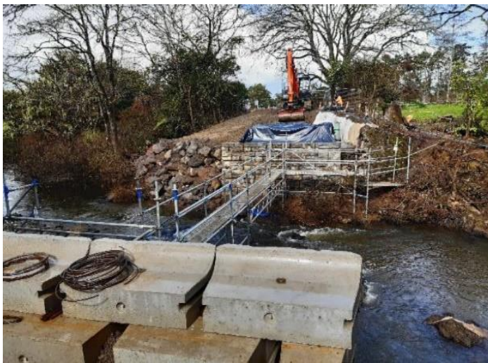
On-going works of Otatau Bridge replacement
