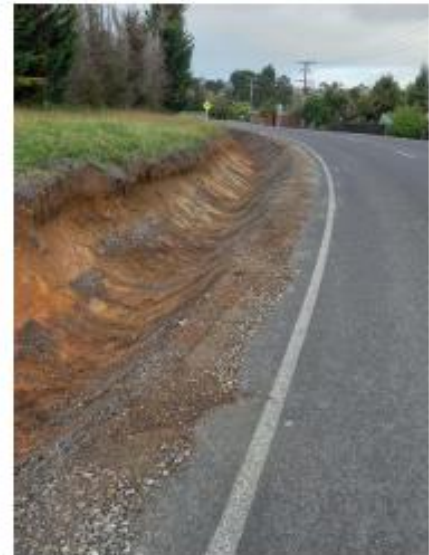
Waimate North – Watertable Repairs completed
