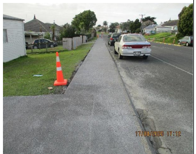
Pukepoto Road Footpath Renewal
