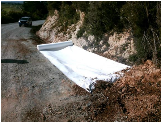
Mine Rd Stage 1 Water table reconstruction
