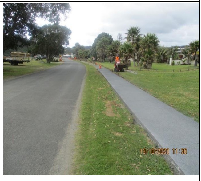
Foreshore/Footpath construction – Concreting
