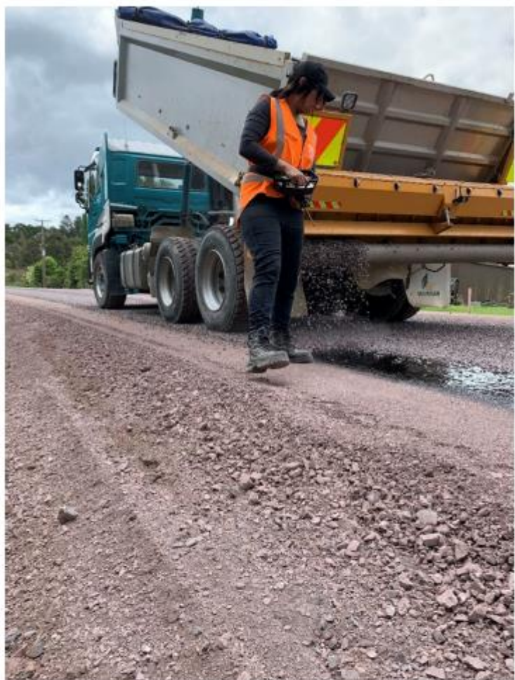
Puketi Rd – Jodie using the brand new roller spreader with 8 gate remote.
