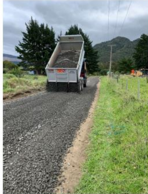
Waima School Rd dust seal – stabilising and chipseal to follow in early Nov
