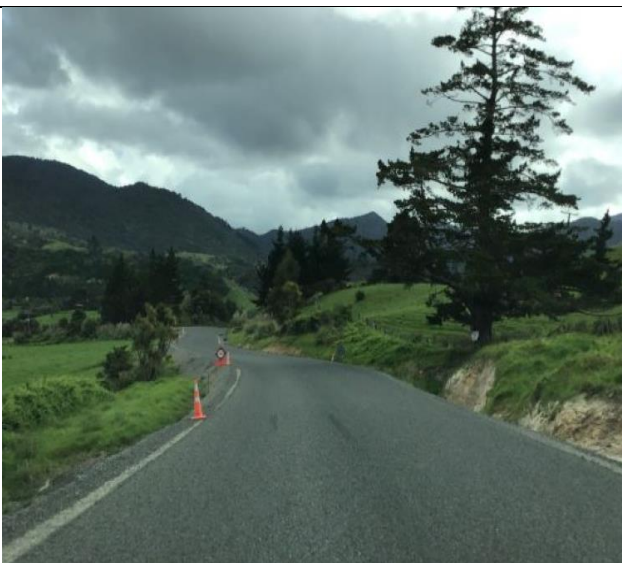
Broadwood Rehabilitation/Sealing completed
