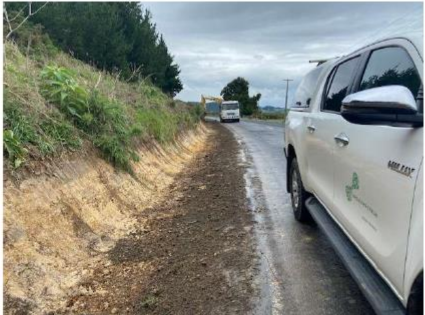
Horeke Rd – Water tabling.
