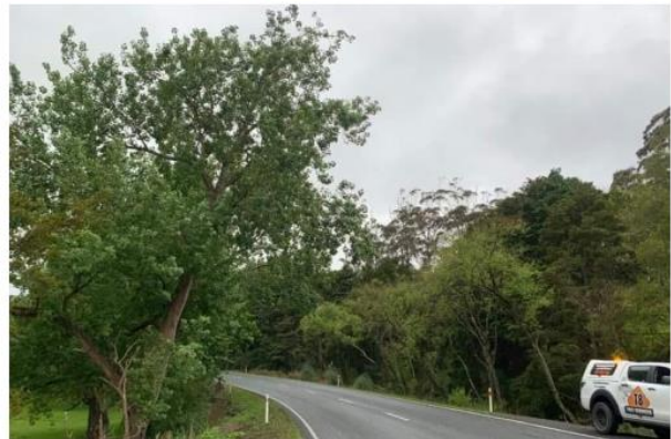
Site 9. RP 15399 – 15404: Removal of heavily leaning Poplar tree to ground level (no photo)
