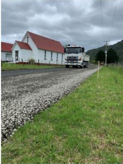
Waima School Rd dust seal – stabilising and chipseal to follow in early Nov
