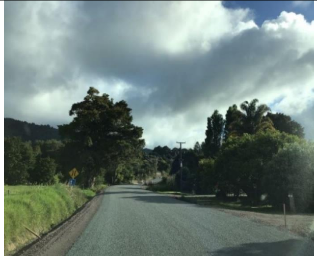
Puketi Seal Extension/Sealing works completed
