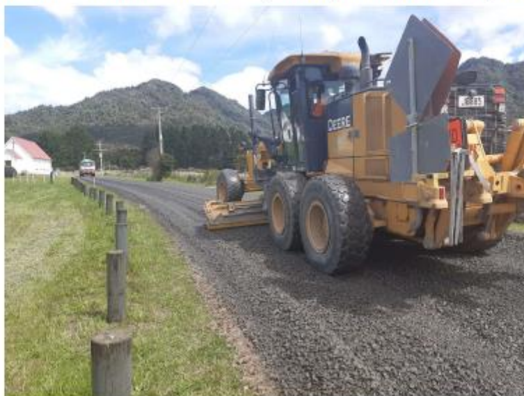
Waima School Rd dust seal – stabilising and chipseal to follow in early Nov
