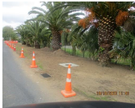
Taipa Drainage preparation
