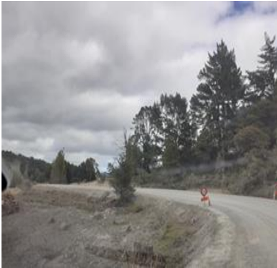
Peria Rd. Cleared Pines on the inside of corner
