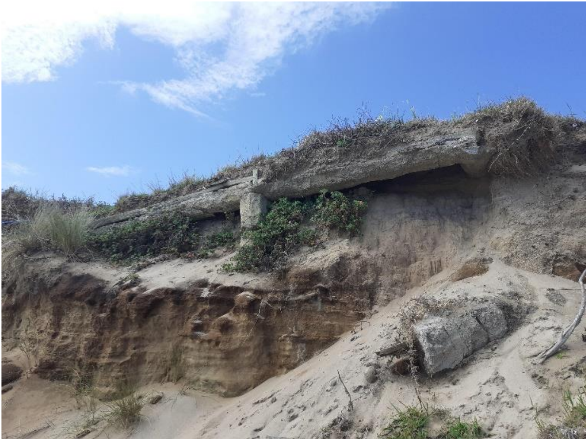
Old concrete foundations to be removed from Lucy Baxter reserve
