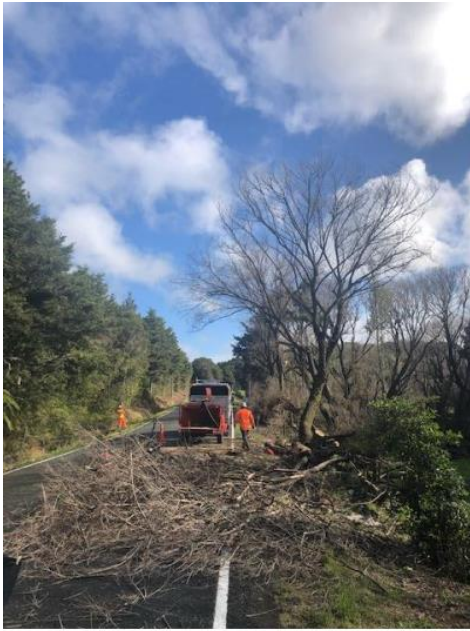
Site 8. RP 15251 – 15256: Removal of leaning Poplar trees to ground level and clear fallen debris from culvert.
