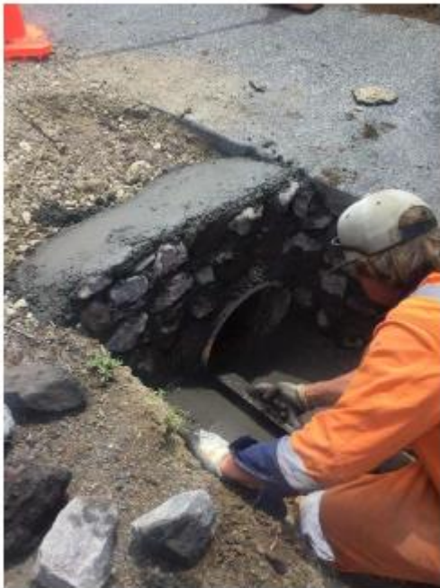
Lance installing a headwall on Blacks Rd
