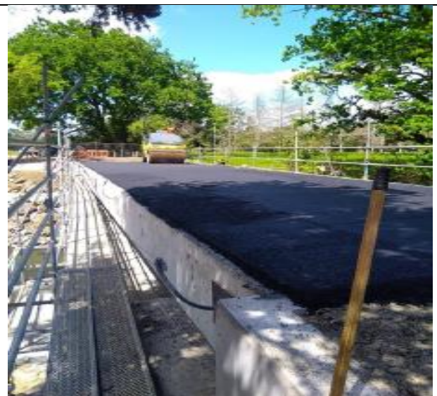
Otaua Road Bridge/Deck Surfacing work in progress
