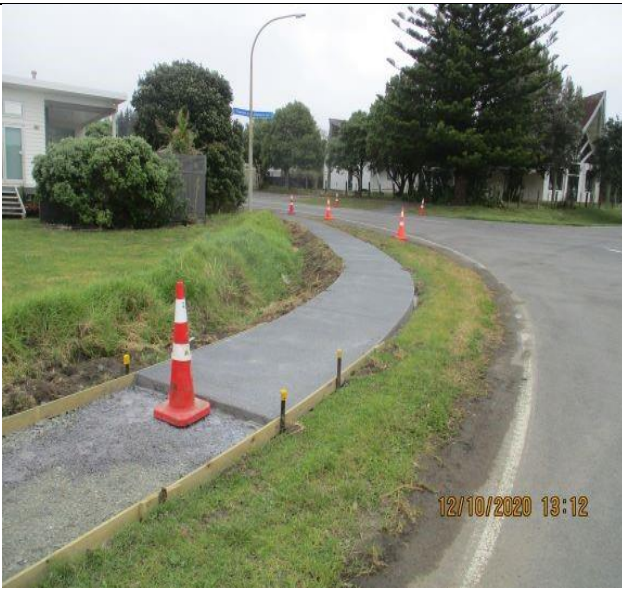
Mamaru/Footpath construction – Concreting
