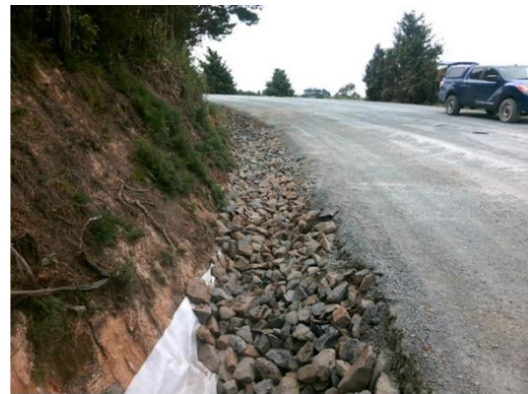
Mine Rd Stage 1 Water table reconstruction
