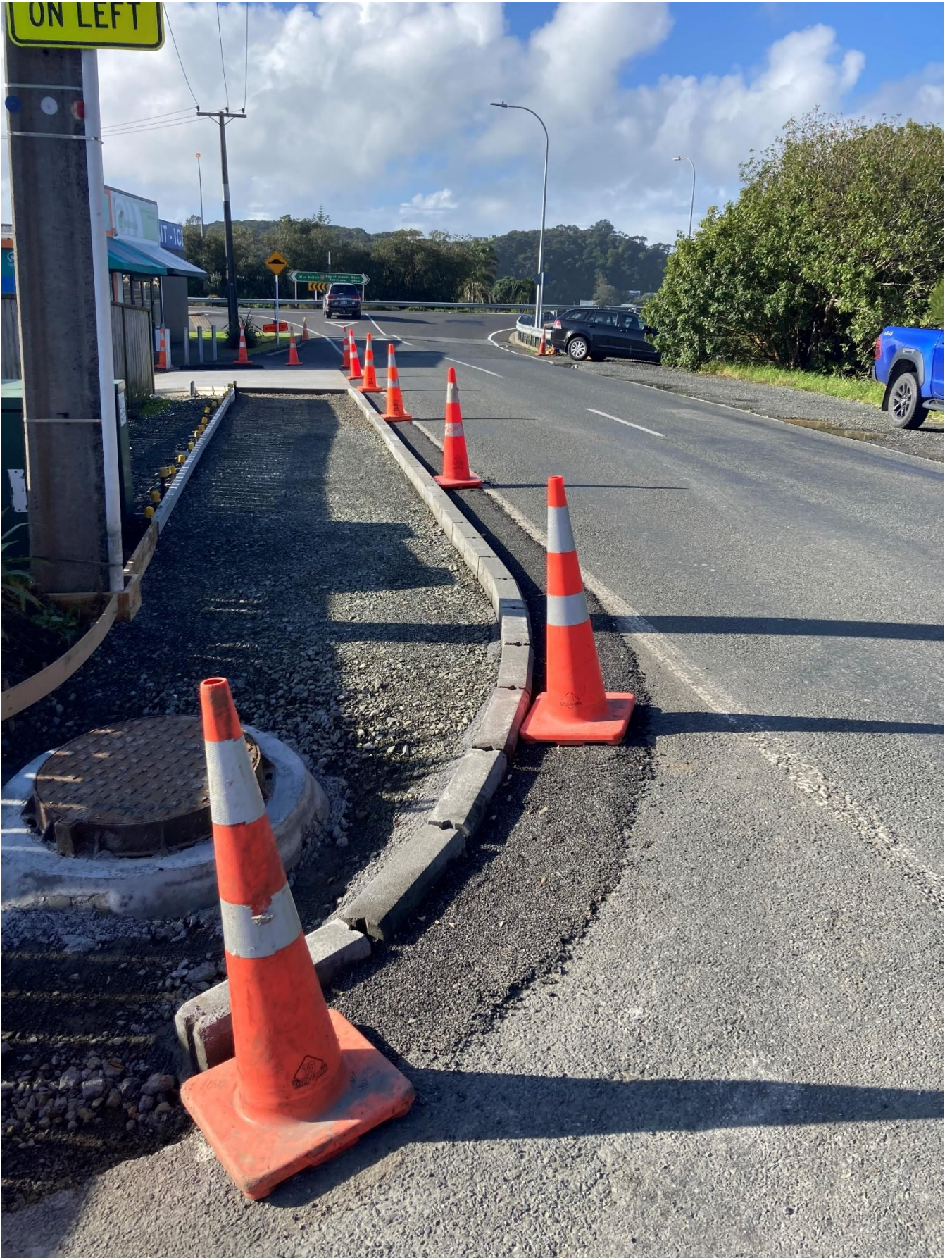
Oruru Rd New Footpath Construction
