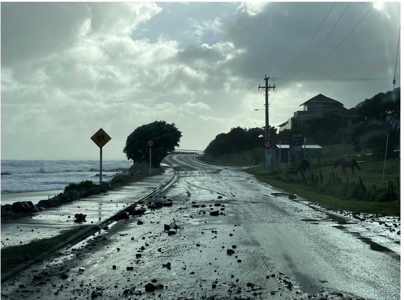
Foreshore Rd Ahipara Tsunami Surge
