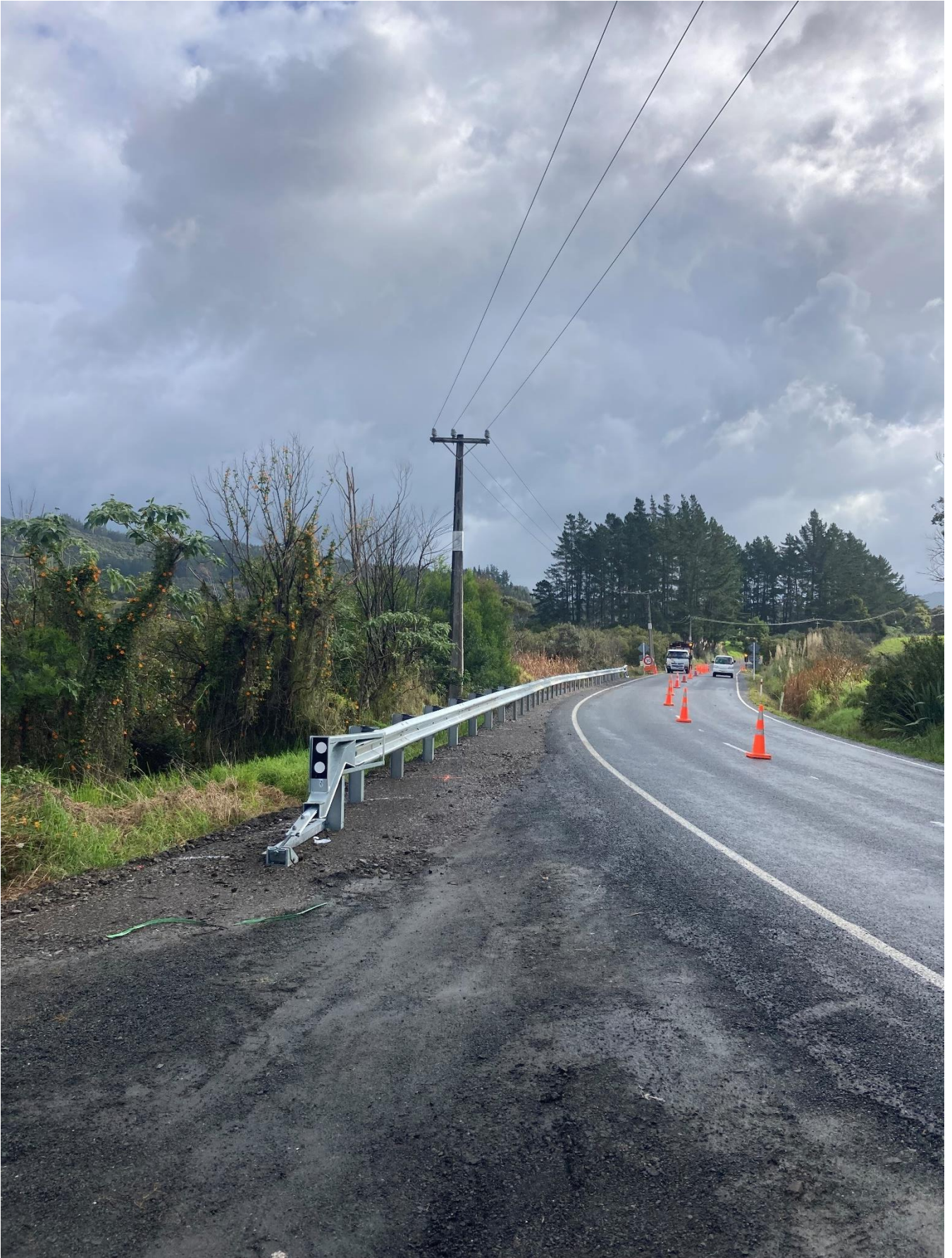
Mangamuka Rd New Guardrail Install HRRi Contract
