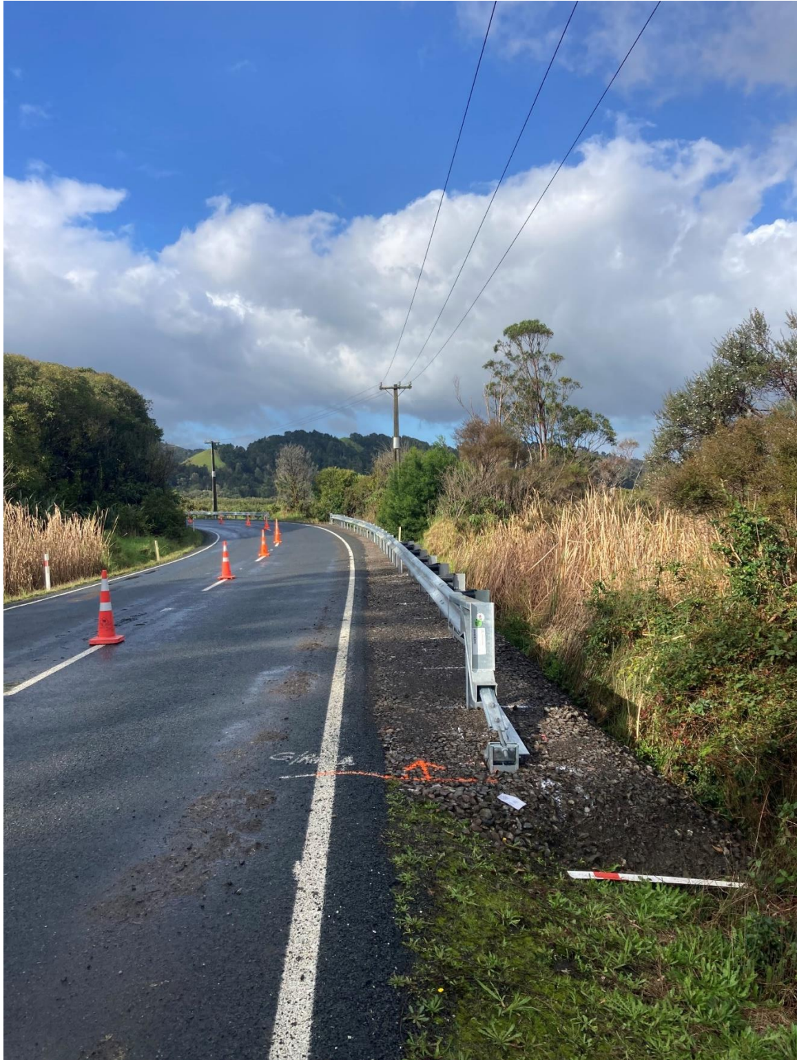
Mangamuka Rd New Guardrail Install HRRi Contract
