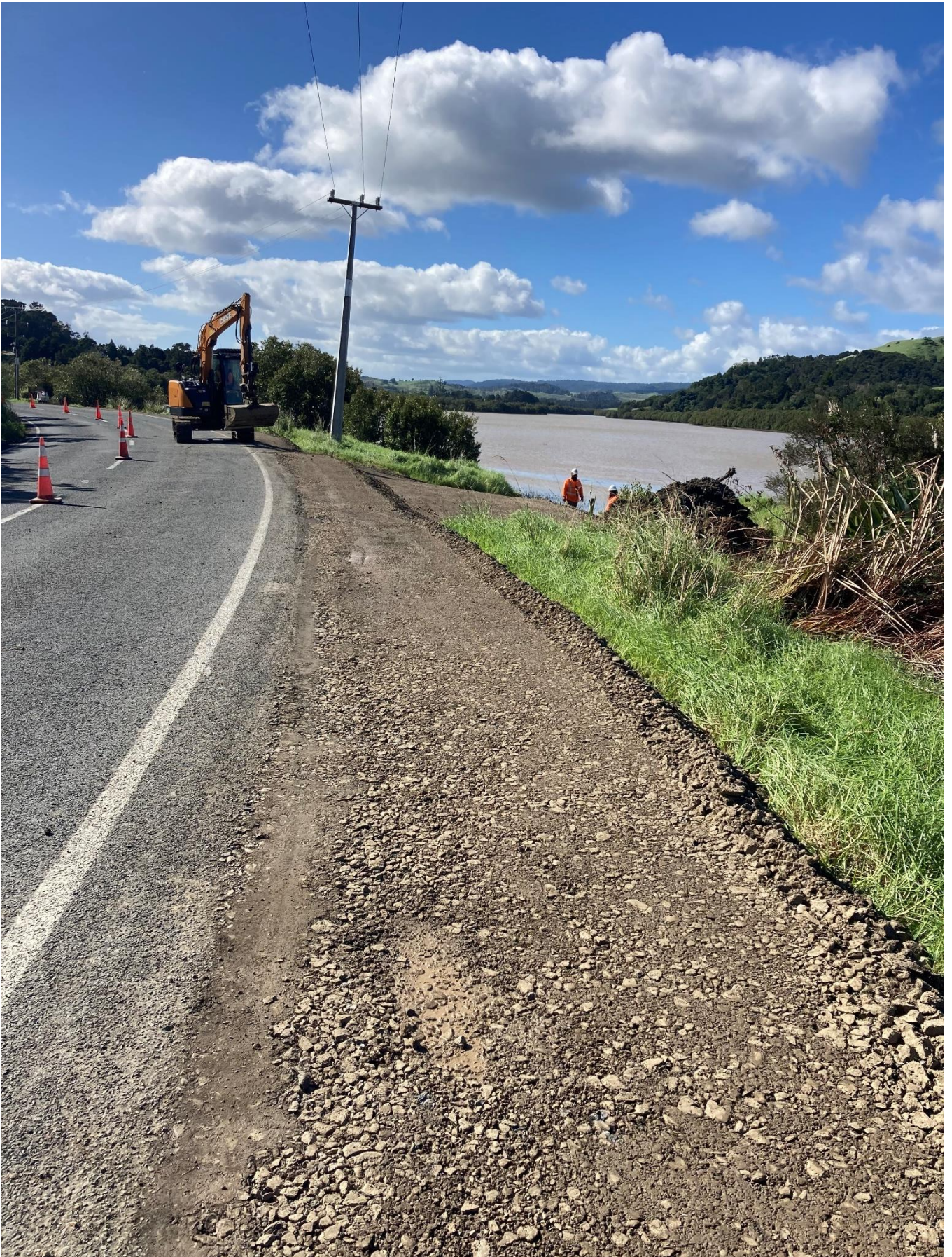
Mangamuka Rd New Guardrail Install HRRi Contract
