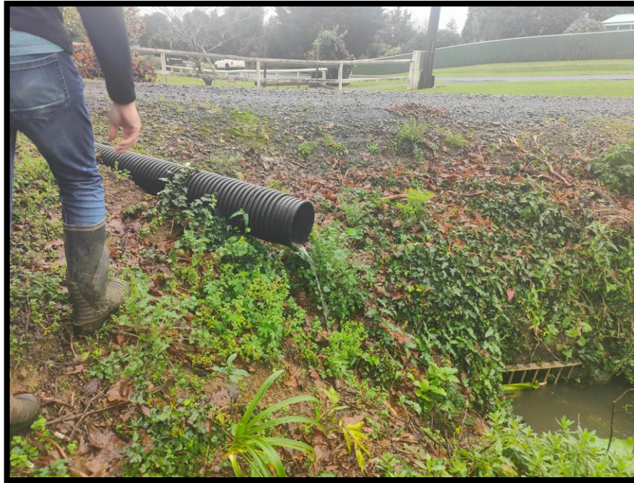
Figure 3 – Existing plastic culvert to be replaced
