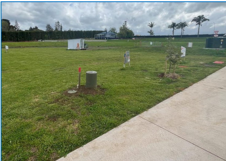
Photograph 1: View west over the subject site from Te Uru Lane. Existing service connections are visible.
