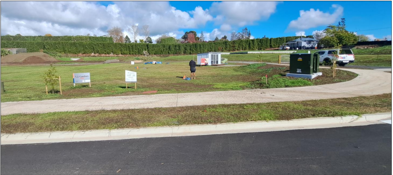
Figure 3: Site photograph of the property (southwest direction). Orange cones depict the building site.
