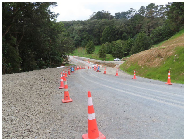
Figure 4) Last section of road realignment progressing, this section of road required redesign due to the 2.1dia culvert extension requirements, the redesign was seen as a benefit as it also provided safety & environmental improvements by shifting the traffic away from the stream inlet and the shared landowner farm accessway and removing a sharp corner to provide a safer journey for all road users.
