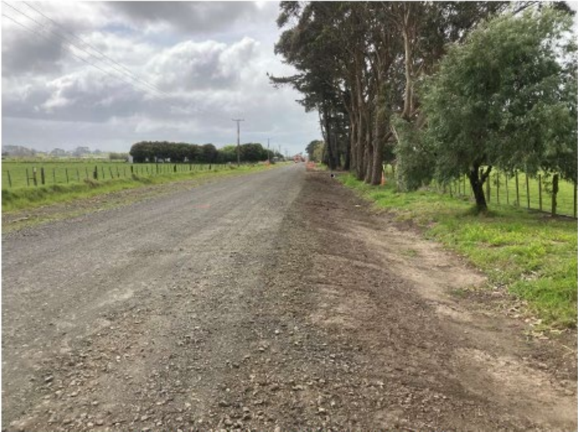
Clearing / Water tabling on Brass Road Seal Extension
