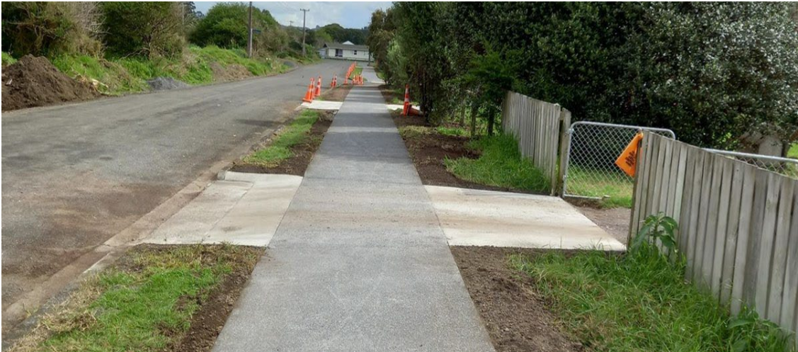
Reed Street – New Footpath
