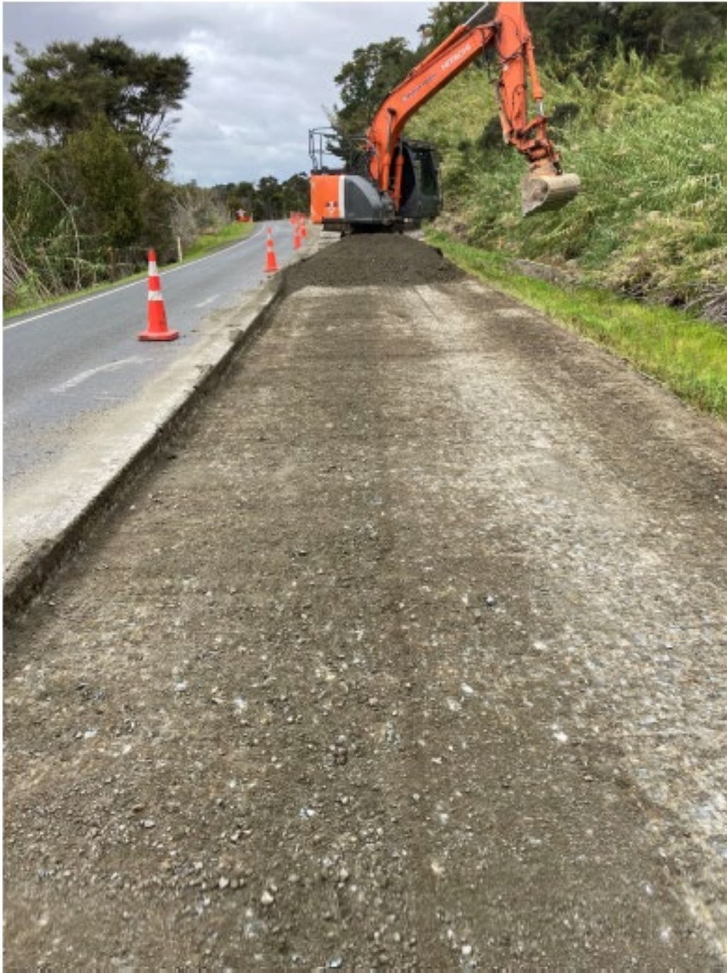
Pavement undercut on the Kohukohu Rd Pavement Rehabilitation
