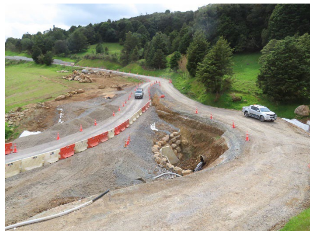
Figure 4) Last section of road realignment progressing, this section of road required redesign due to the 2.1dia culvert extension requirements, the redesign was seen as a benefit as it also provided safety & environmental improvements by shifting the traffic away from the stream inlet and the shared landowner farm accessway and removing a sharp corner to provide a safer journey for all road users.
