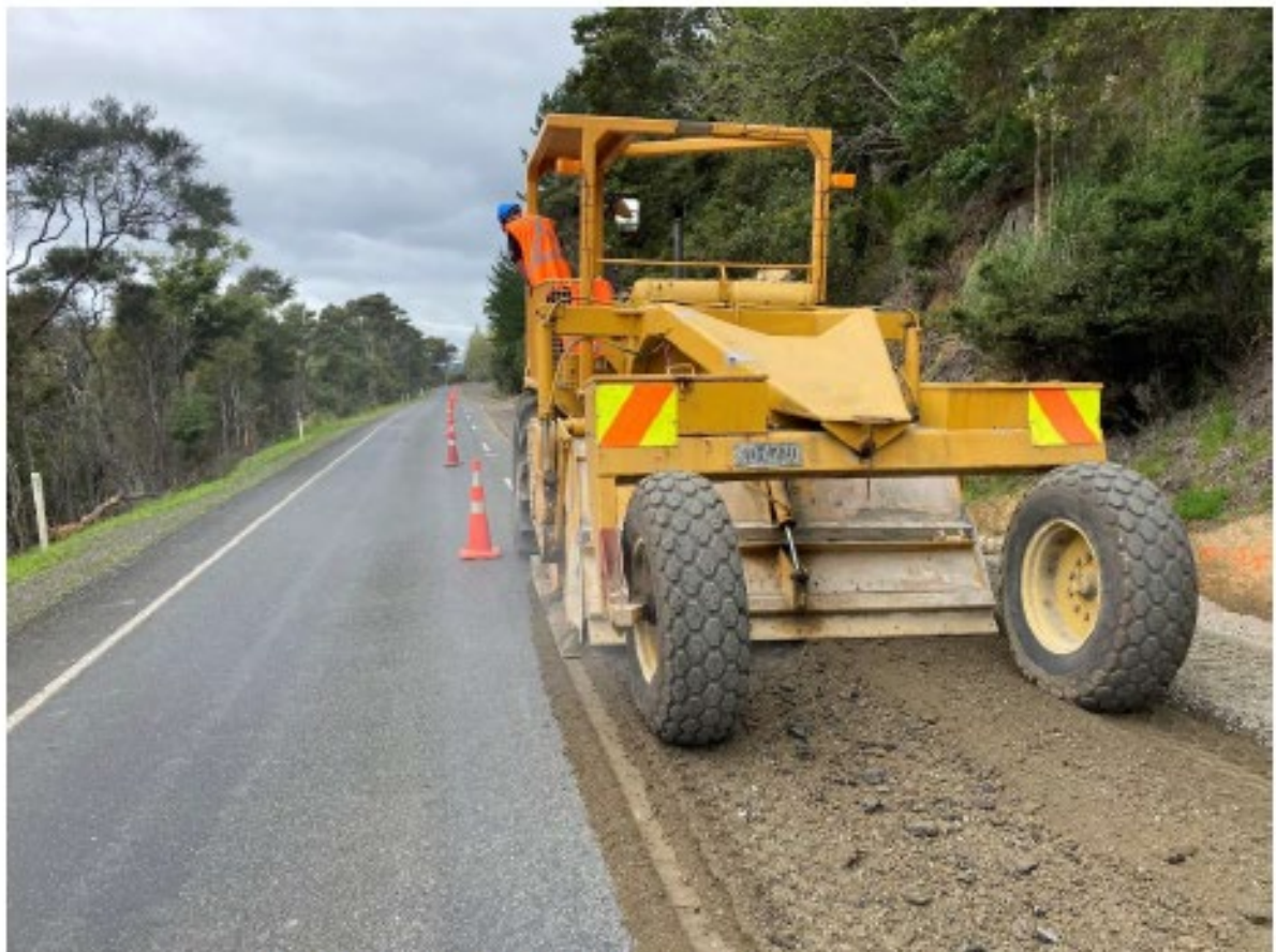
Pre-hoeing on the Kohukohu Rd Pavement Rehabilitation
