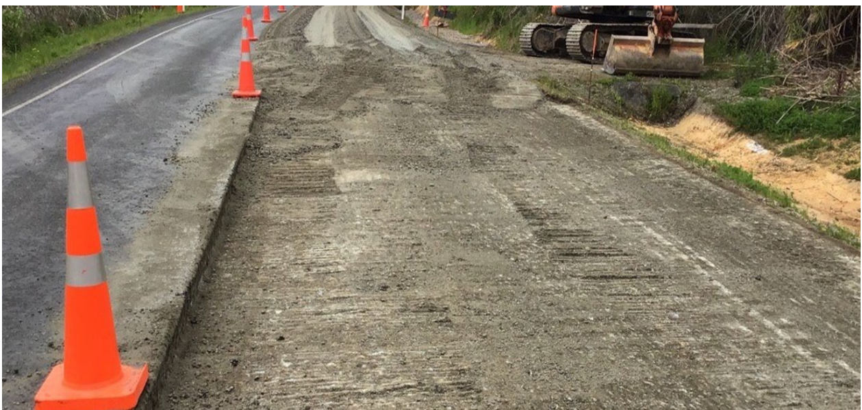
Kohukkohu Road Rehabilitation
