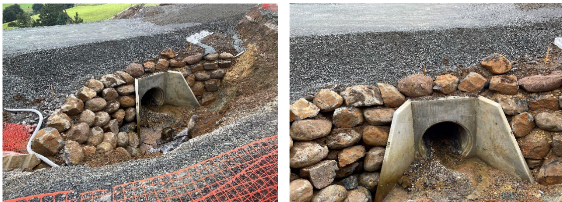
Figure 2) 2.1dia culvert headwall, wingwalls and benched in rock walls
