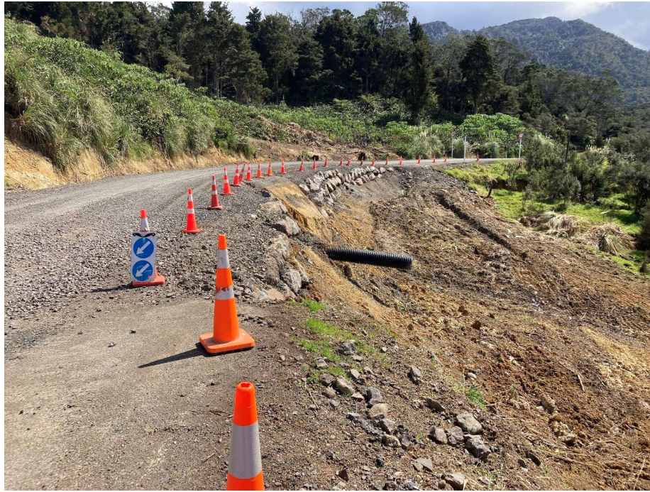
West Coast Rd (Panguru) slip temporary repairs completed this month
