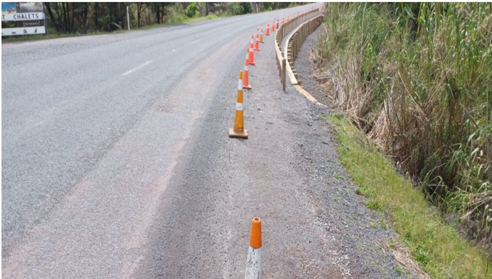
Aucks Road – Slip Repair
