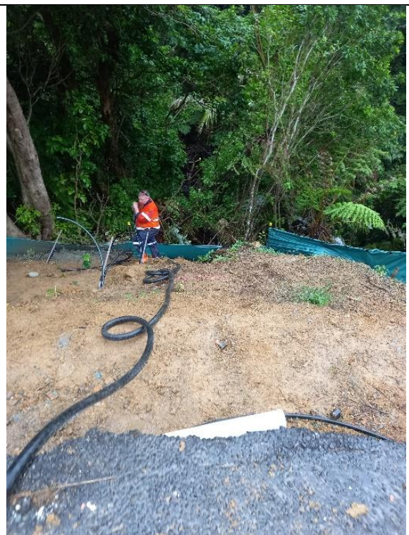
Manawaora Slip Repair – Installation and grouting of Sacrificial Soil Nails
