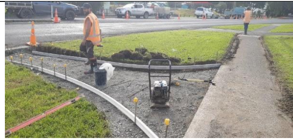
Dominion Rd Bank Street (Kaitaia) new footpath crossing connection
