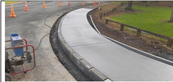
Dominion Rd Bank Street (Kaitaia) narrowing of Bell mouth and new footpath
