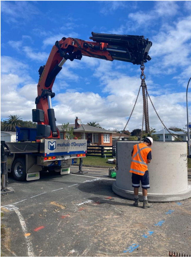
Sommerville Ave SW Upgrade Manhole Delivery and Installation
