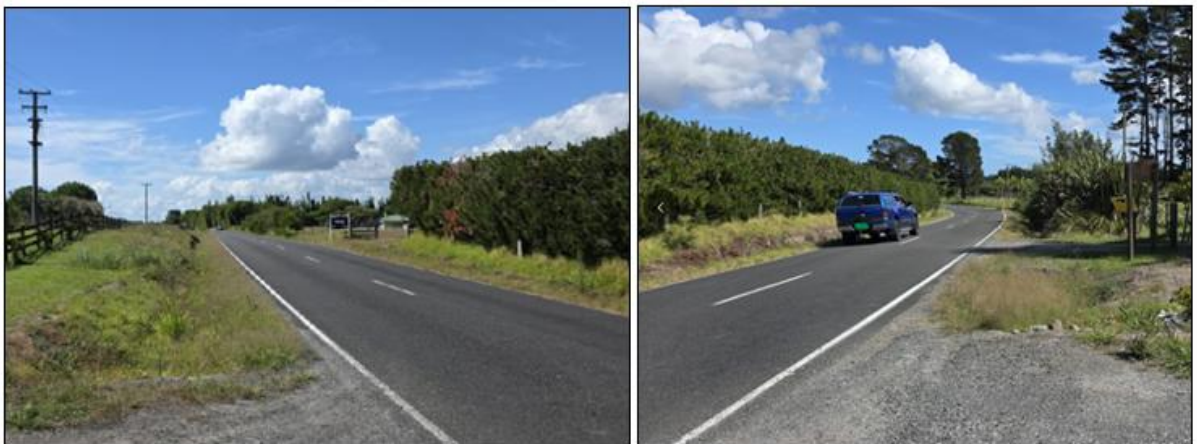
Figure 11: Photographs demonstrating sight distances from existing access to proposed Lot 2 (left looking east and right looking west).
