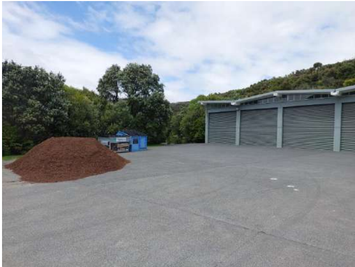
Existing sheds 1-4 and concrete apron
