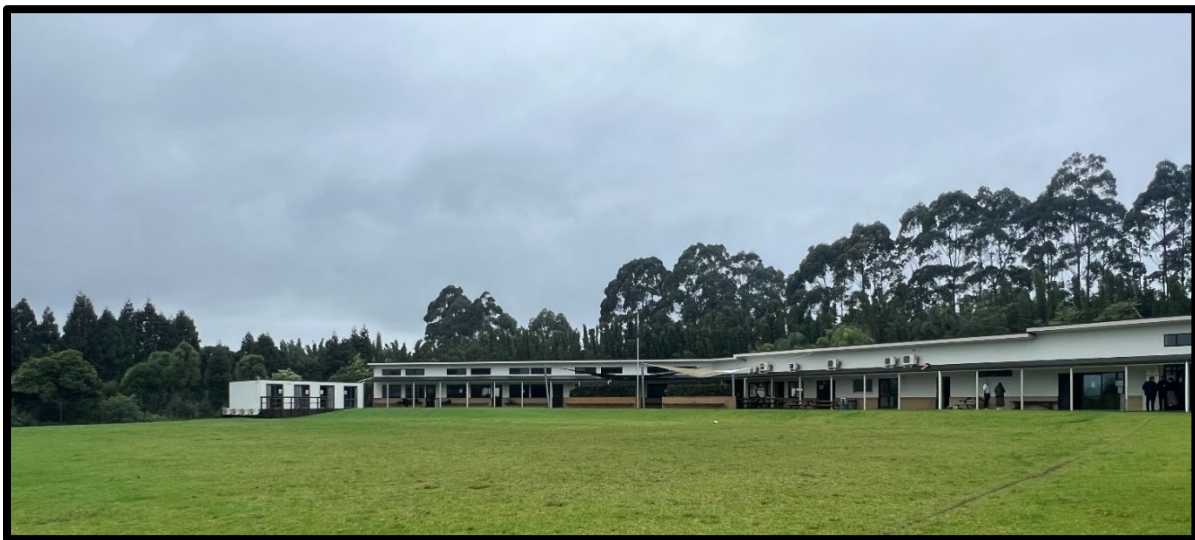
Photo 4: View of existing school looking south east
