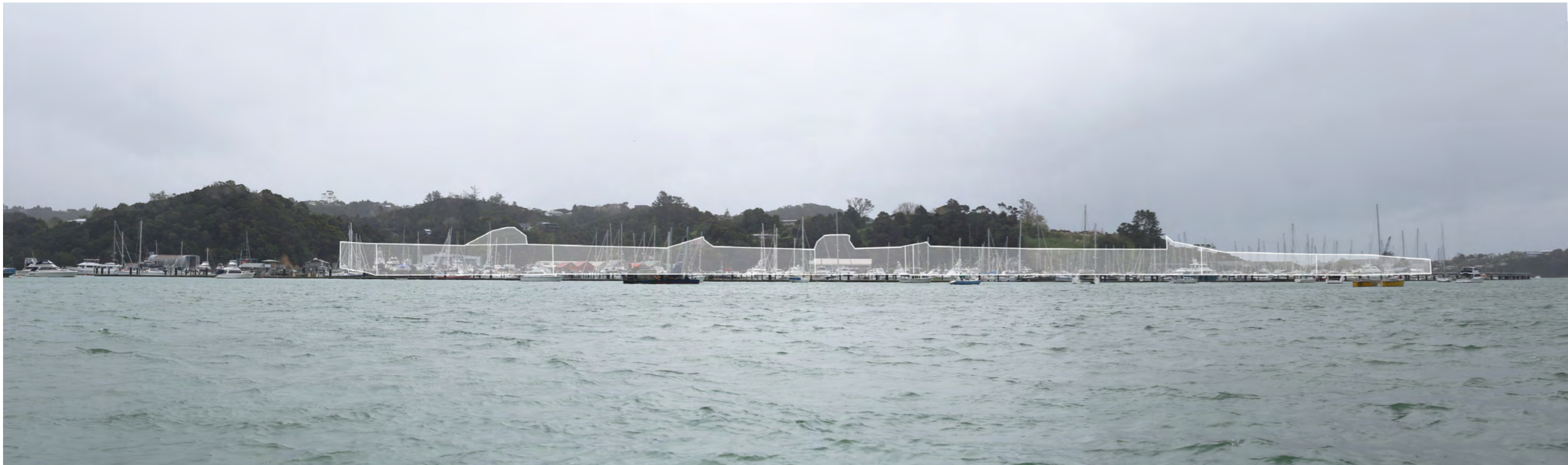
VIEW FROM THE KAWAKAWA RIVER, LOOKING NORTHWEST TOWARDS OPUA MARINA DEVELOPMENT AREA
