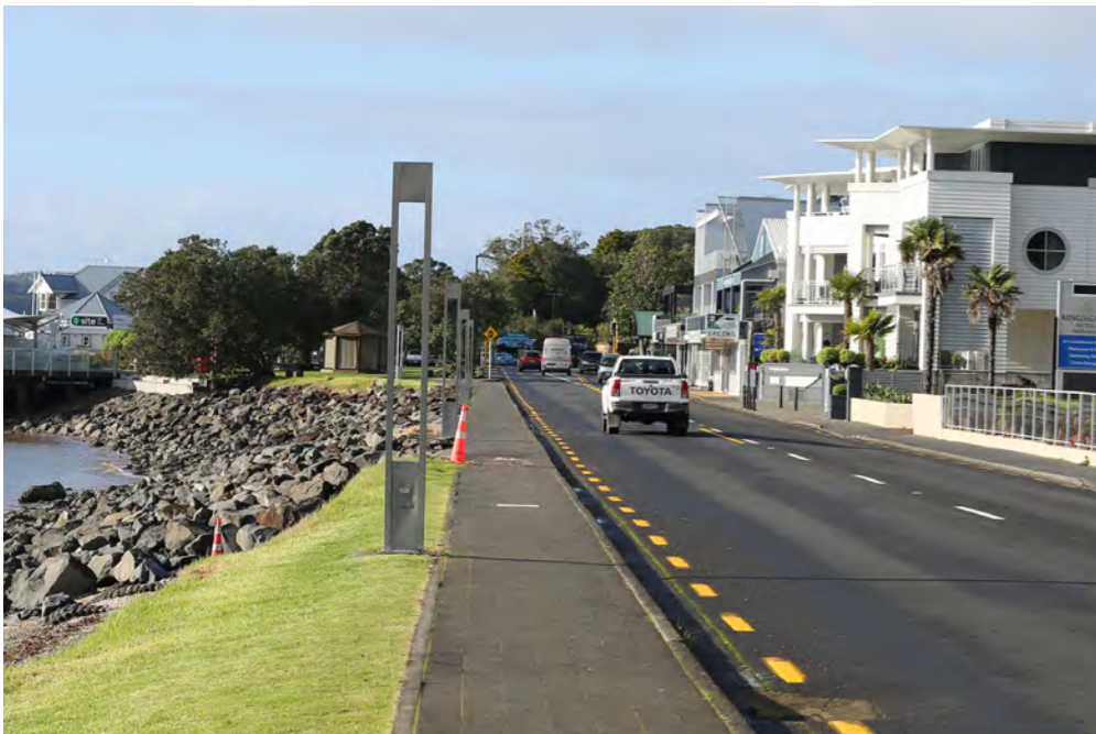
Paihia - relationship between the water and built development
