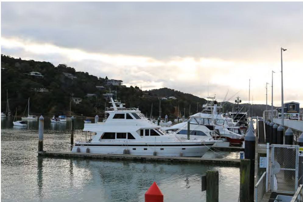
Opua Marina, berths and wharf
