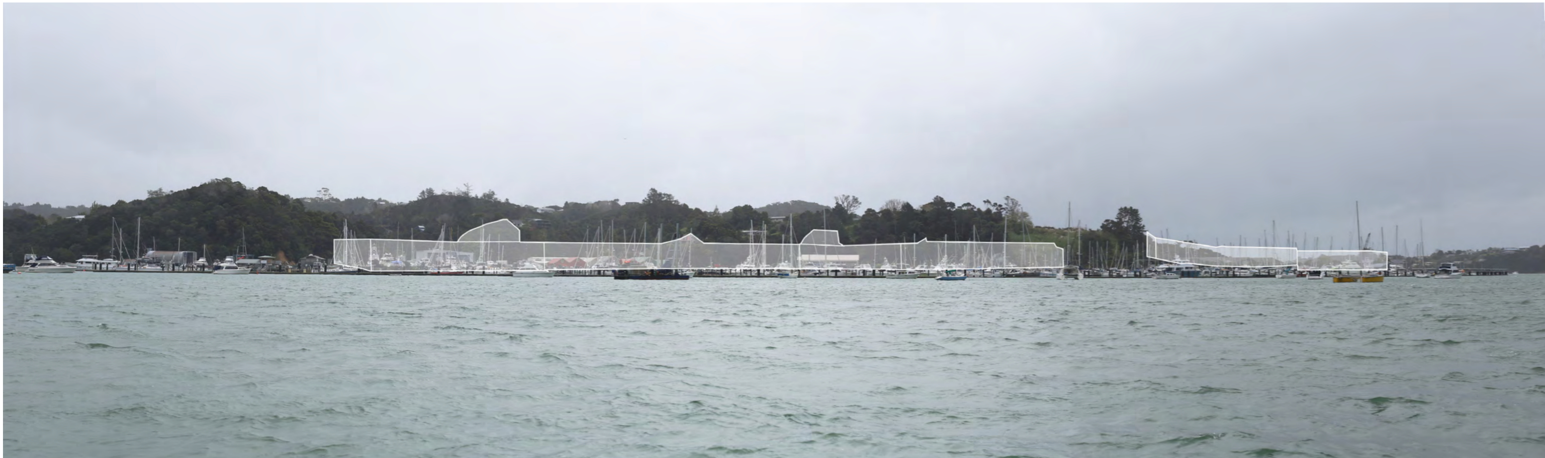
VIEW FROM THE KAWAKAWA RIVER, LOOKING NORTHWEST TOWARDS OPUA MARINA DEVELOPMENT AREA
