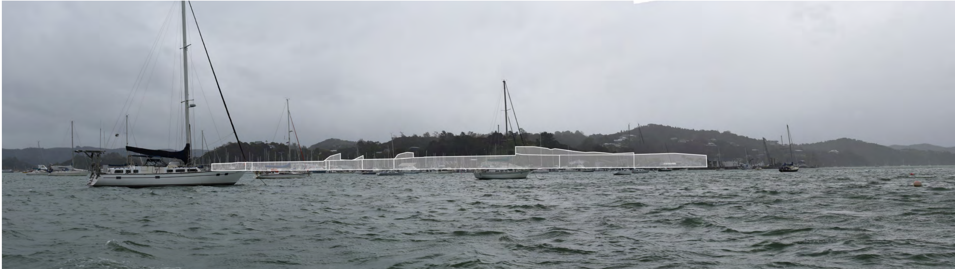
VIEW FROM THE INTERSECTION OF KAWAKAWA RIVER AND WAIKARE INLET, TO THE WEST OF MOTUTOKAPE ISLAND, LOOKING WEST TOWARDS OPUA MARINA DEVELOPMENT AREA
