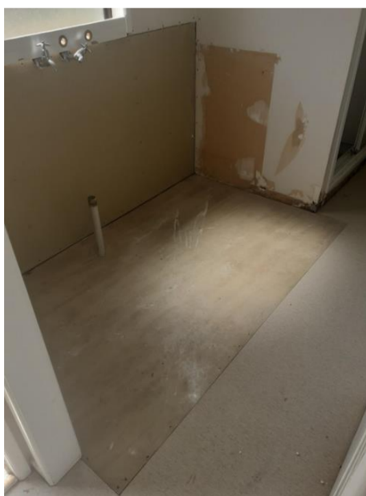
Unit 2, Waima washtub removed, damaged wall lining, and flooring replaced
