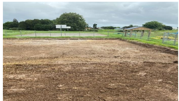
Site prep completed for Allen Bell Park
