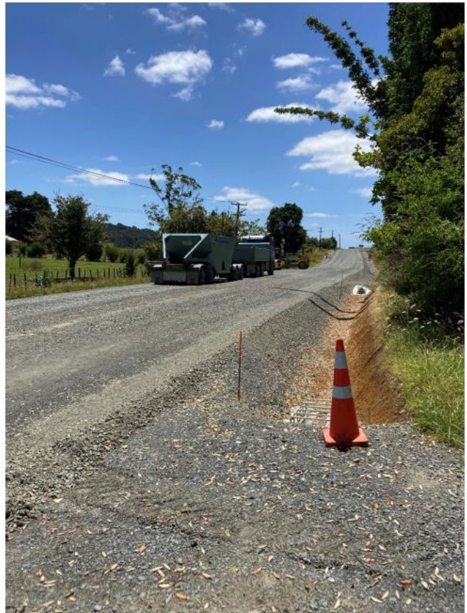
Figure 10: Oruru Rd Rehabilitation Site 1 Pavement Overlay
