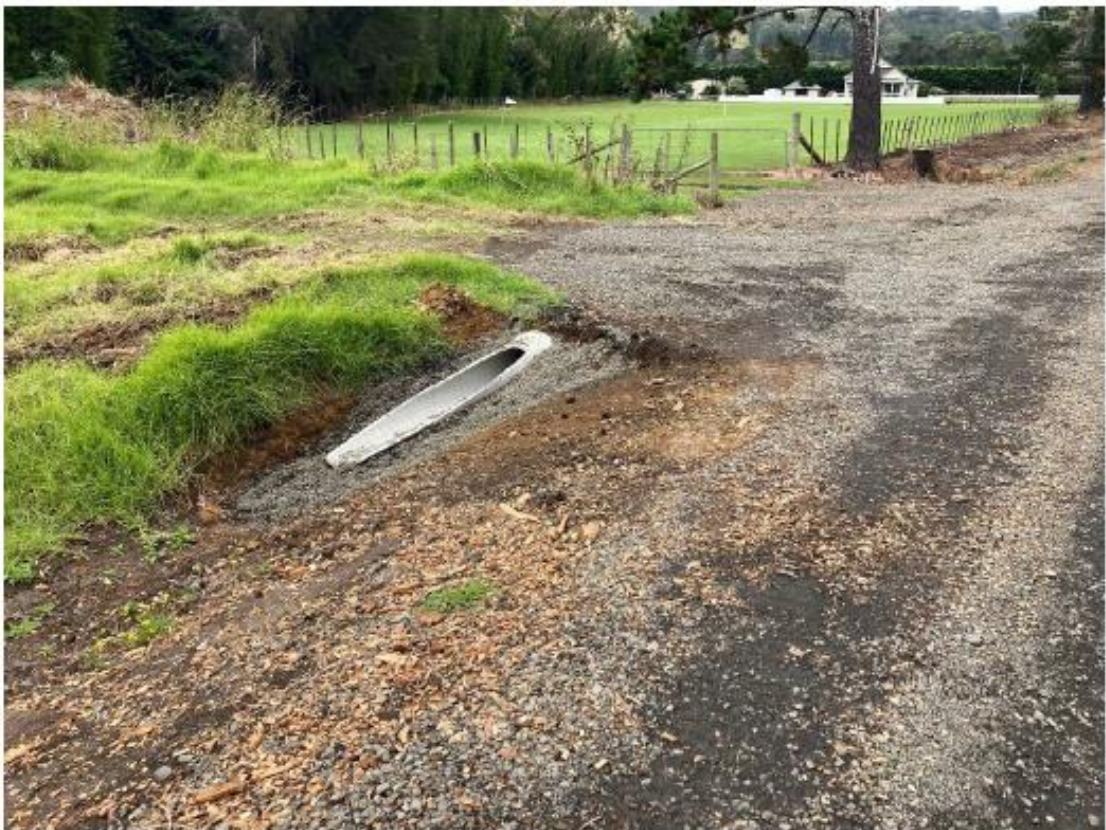
Figure 14: Brass Rd Seal Extension Drainage Works
