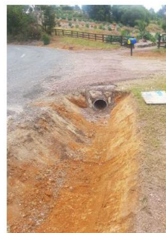
Valencia Lane – 18m of culvert replacement
