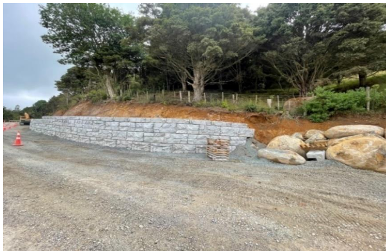
New retaining wall progressing
