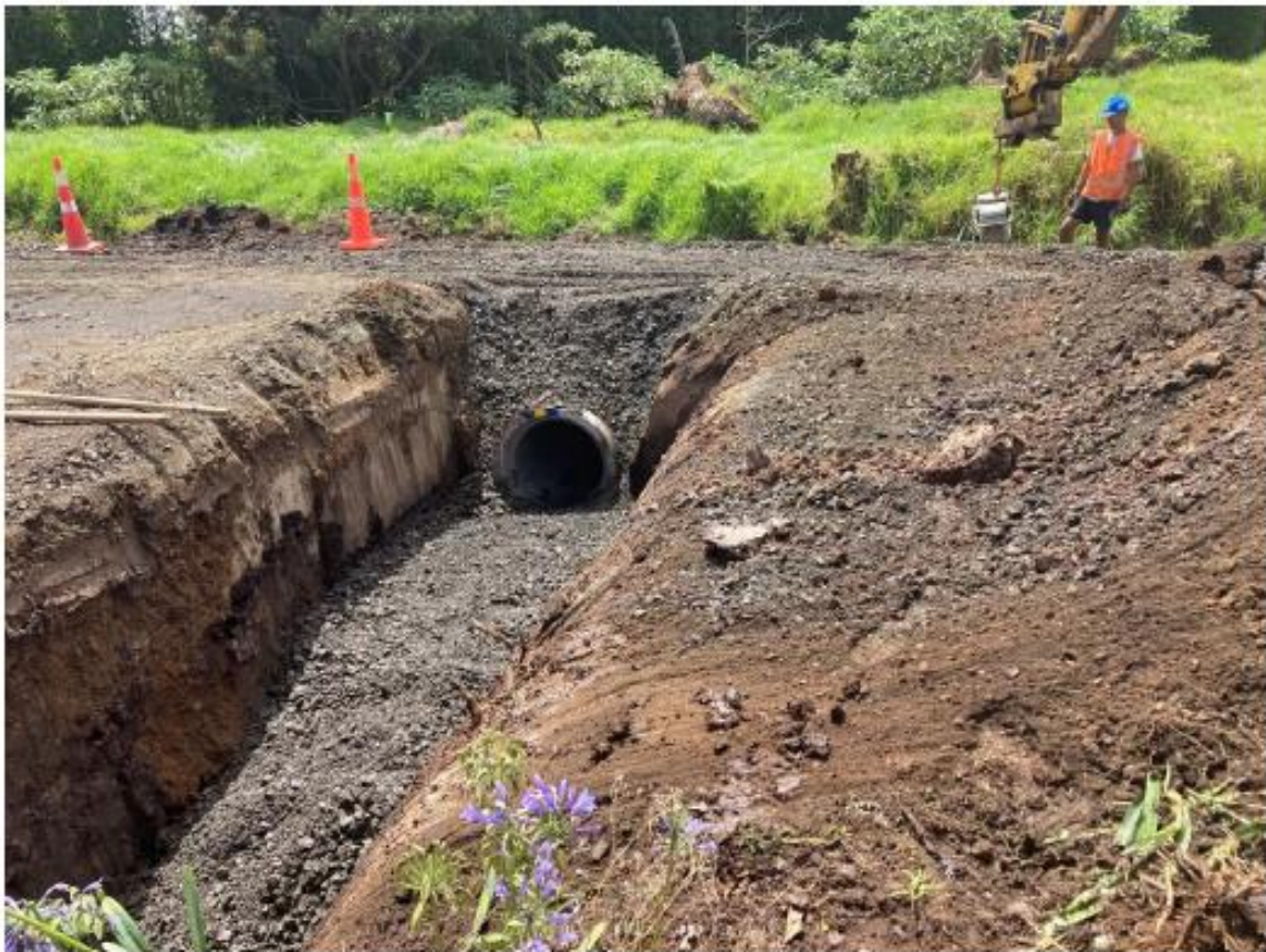
Figure 12: Brass Rd Seal Extension Drainage Works
