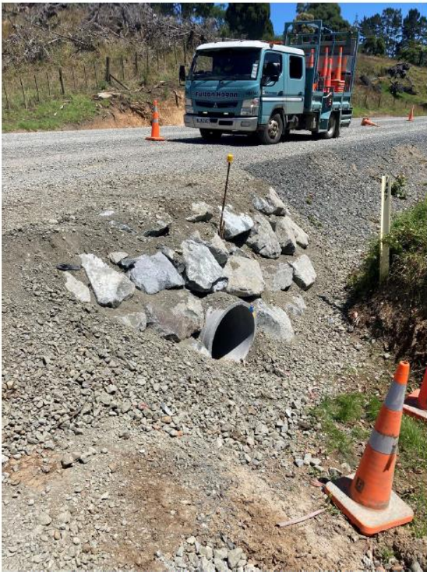
Figure 4: Oruru Rd Rehabilitation Site 2 Headwall Construction
