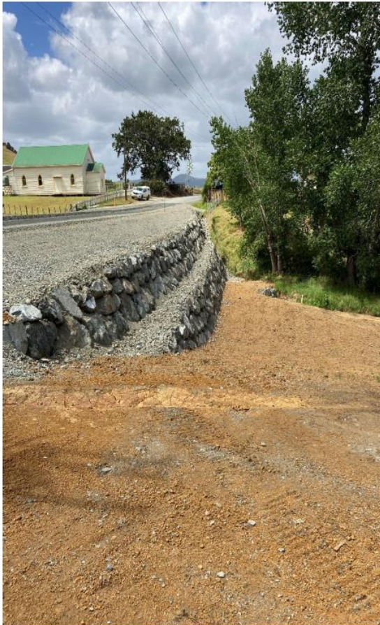
Figure 9: Oruru Rd Rehabilitation Site 1 Rockwall Widening Complete
