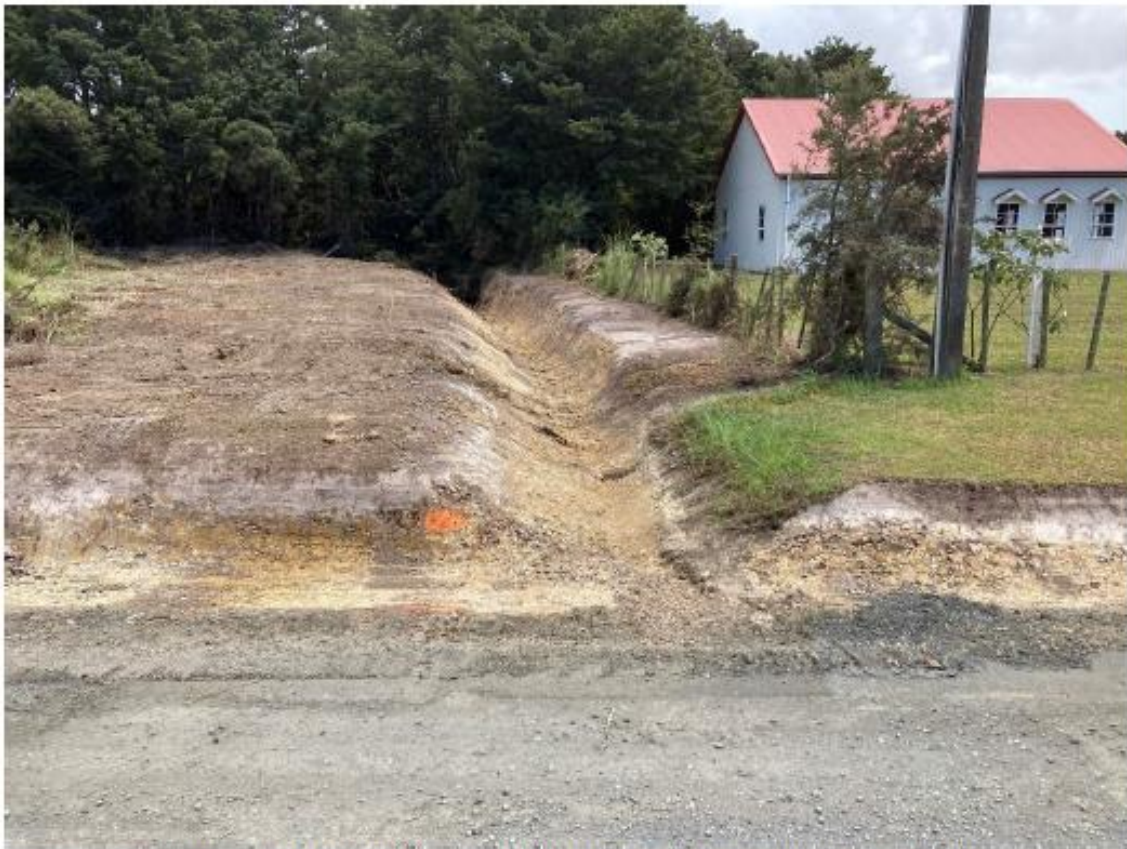
Figure 16: Parapara Toatoa Rd Seal Extension Clearing
