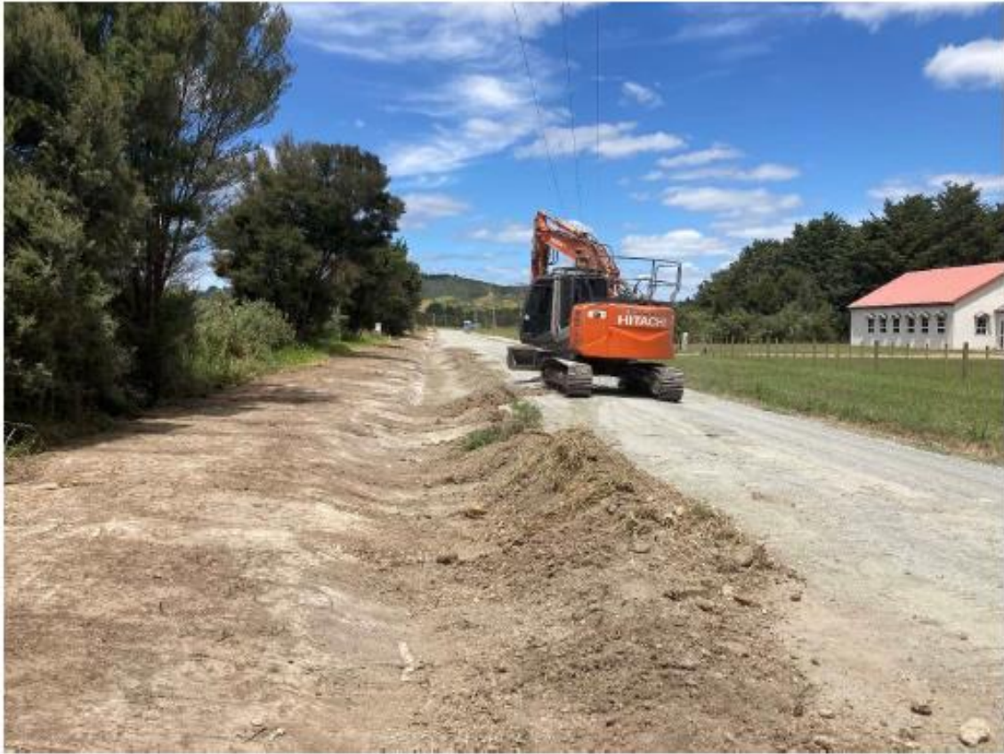
Figure 15: Parapara Toatoa Rd Seal Extension Clearing
