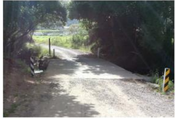
Pakanae Cemetery Rd – Replaced missing BEM
