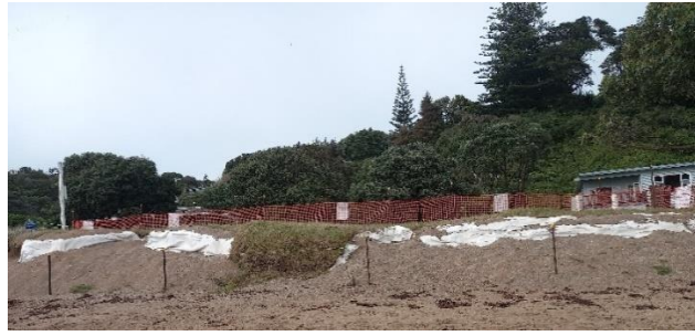
Koiwi site and erosion control work – Long Beach, Russell
