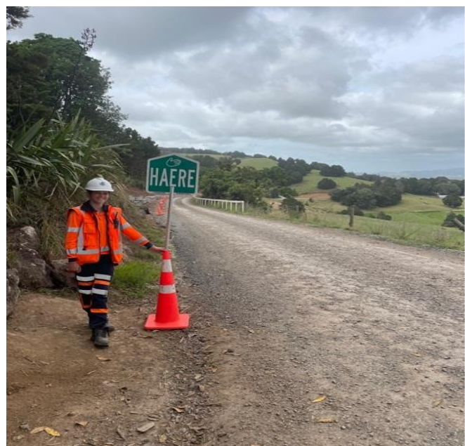
Traffic management located next to the Pa
