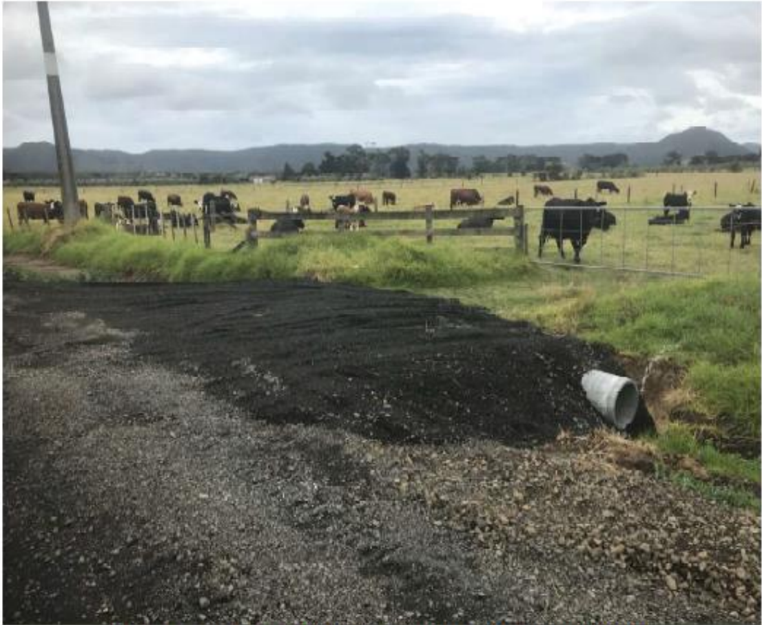
Figure 13: Brass Rd Seal Extension Drainage Works
