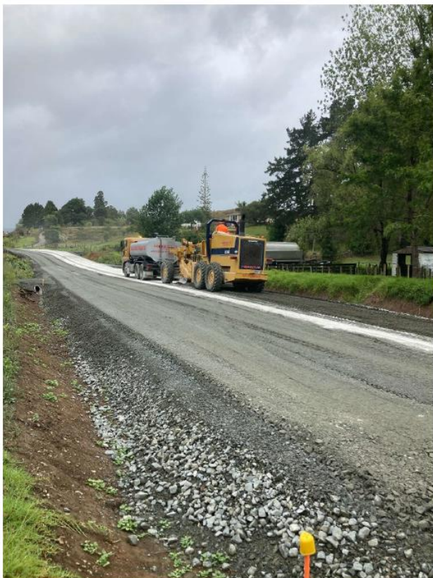
Figure 6: Oruru Rd Rehabilitation Site 2 Stabilising
