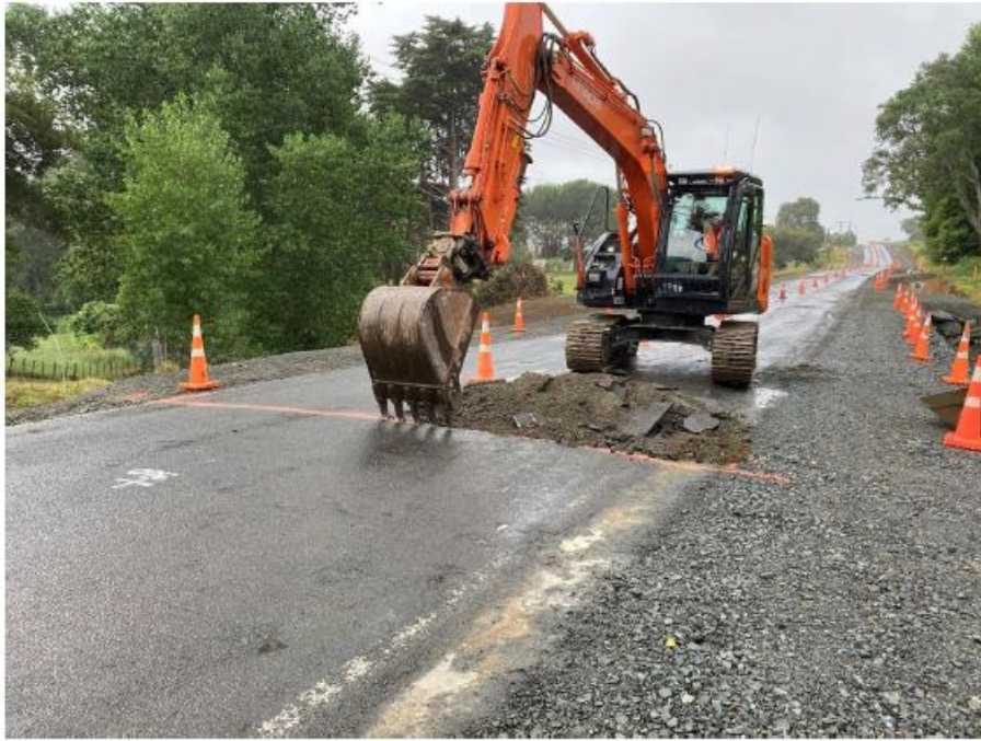
Figure 8: Oruru Rd Rehabilitation Site 1 Pavement Tie-ins
