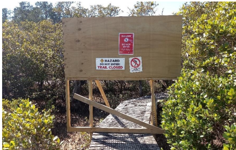
Boardwalk barrier removed by members of the public - Paihia-Opua Walkway
