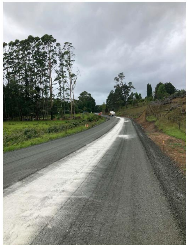
Figure 5: Oruru Rd Rehabilitation Site 2 Stabilising
