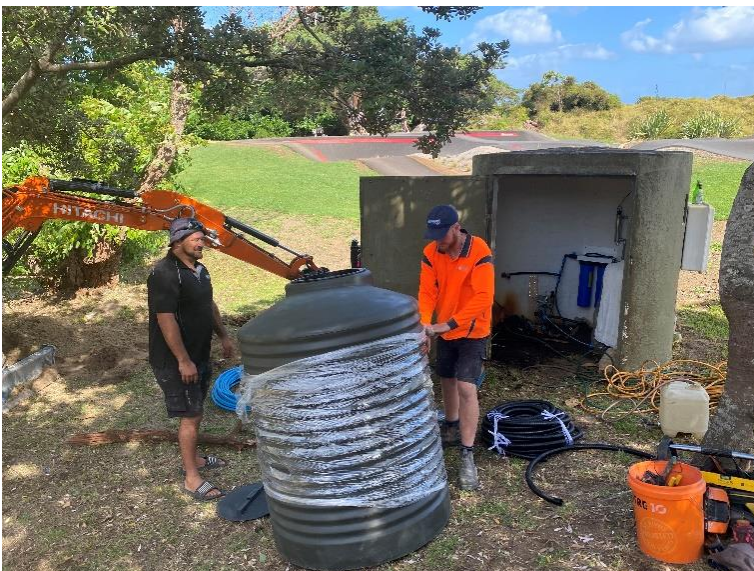
New tank being installed to increase pressure
