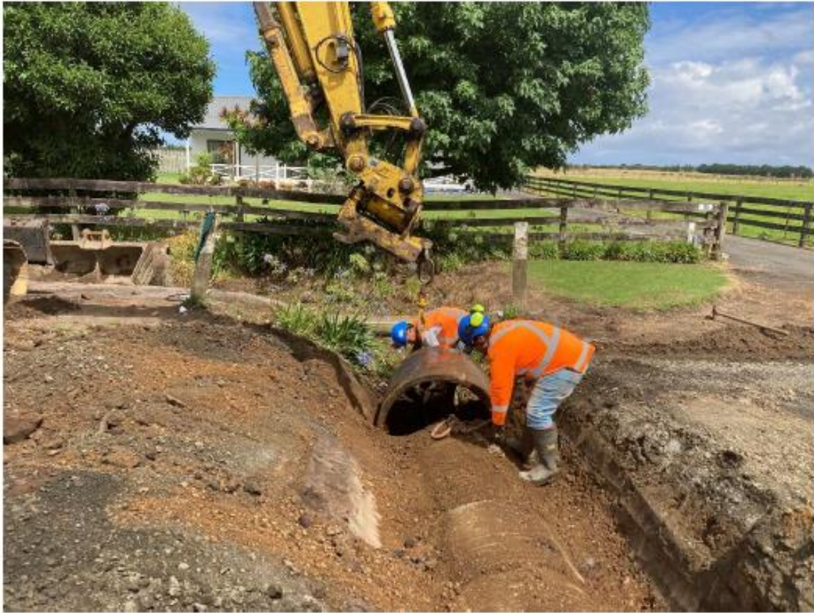
Figure 11: Brass Rd Seal Extension Drainage Works
