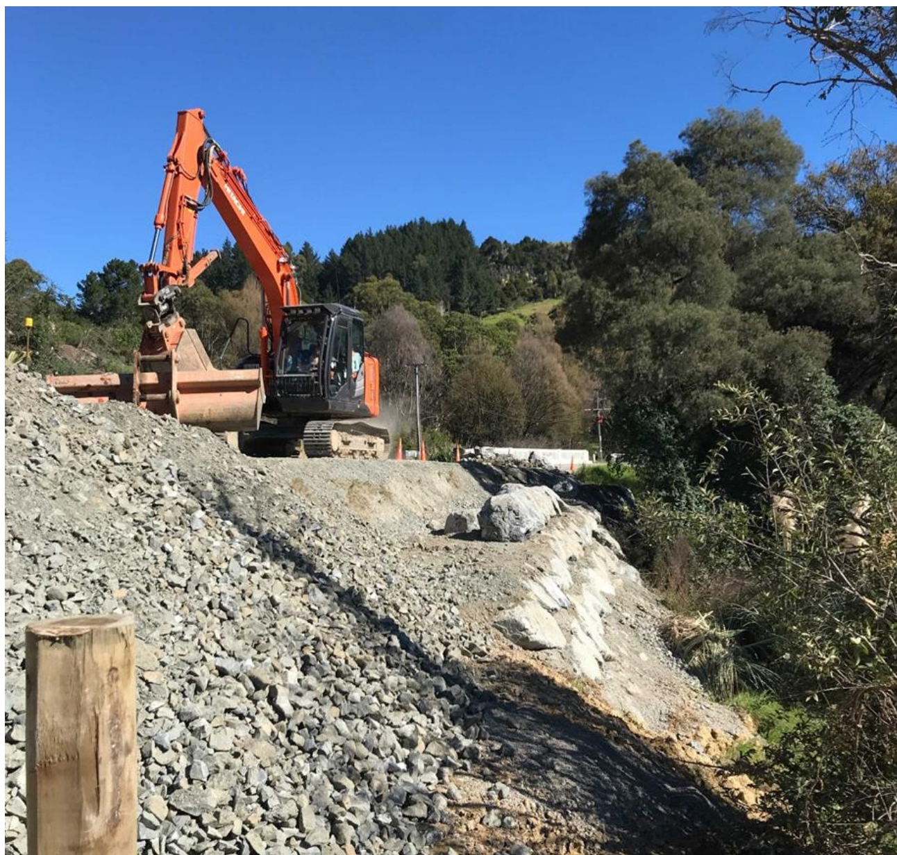
Plenty of Rock Wall construction in progress at Peria on Section 5
