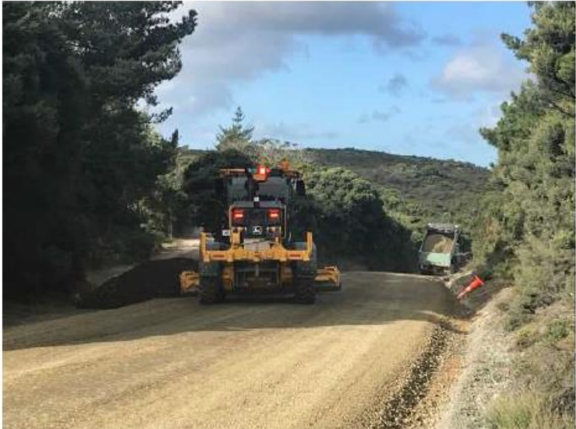
Figure 15: Te Hapua Rd Heavy Metal Overlay
