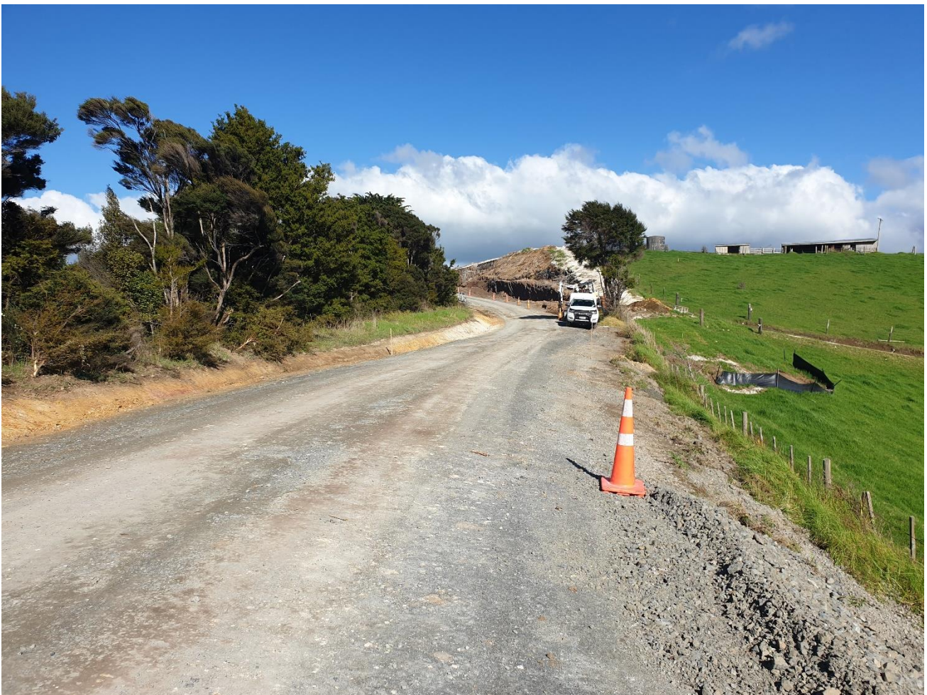
Ruapekapeka Road Stage 1 pavement construction
