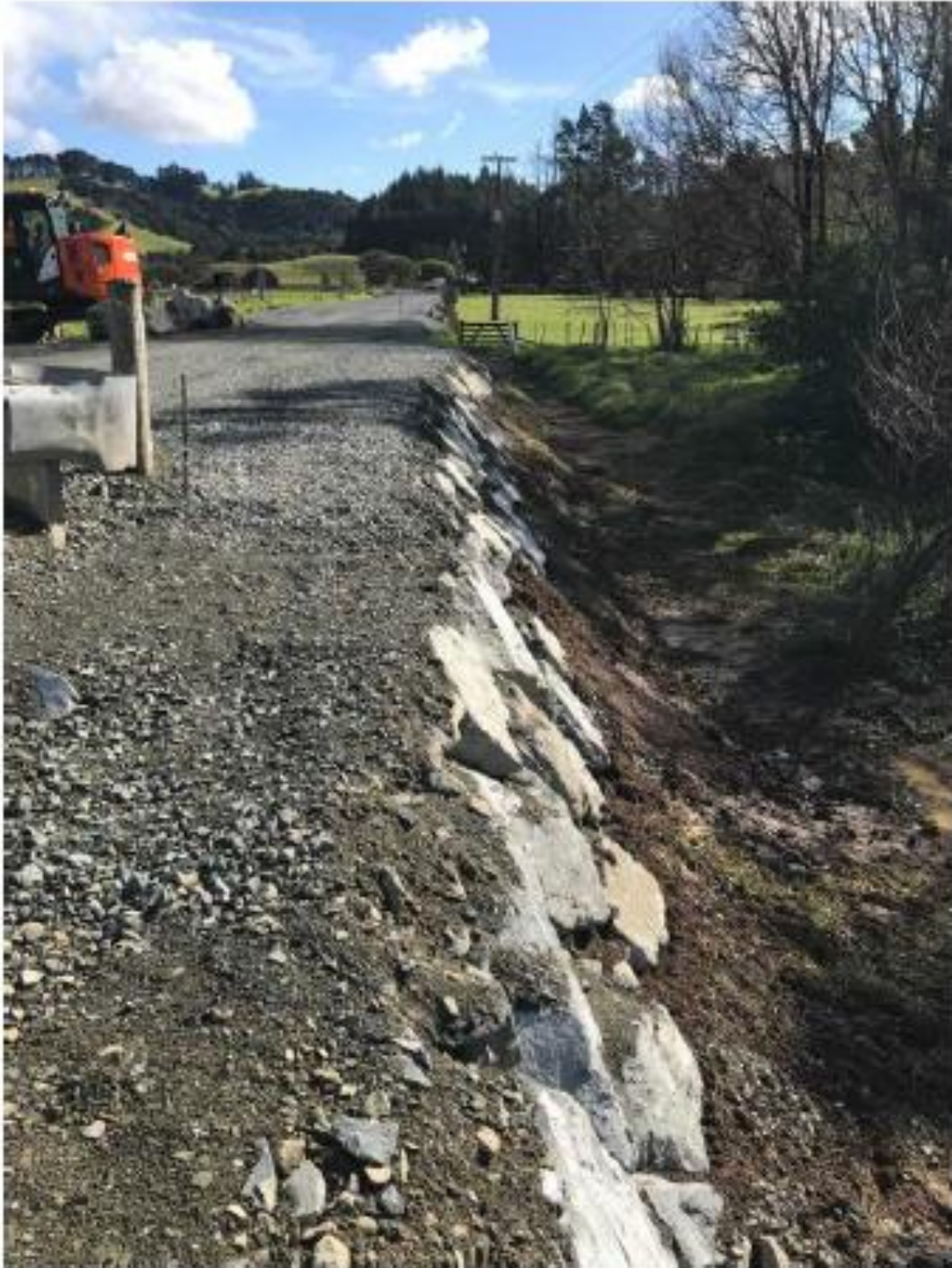
Figure 10: Section 5 Rock wall construction
