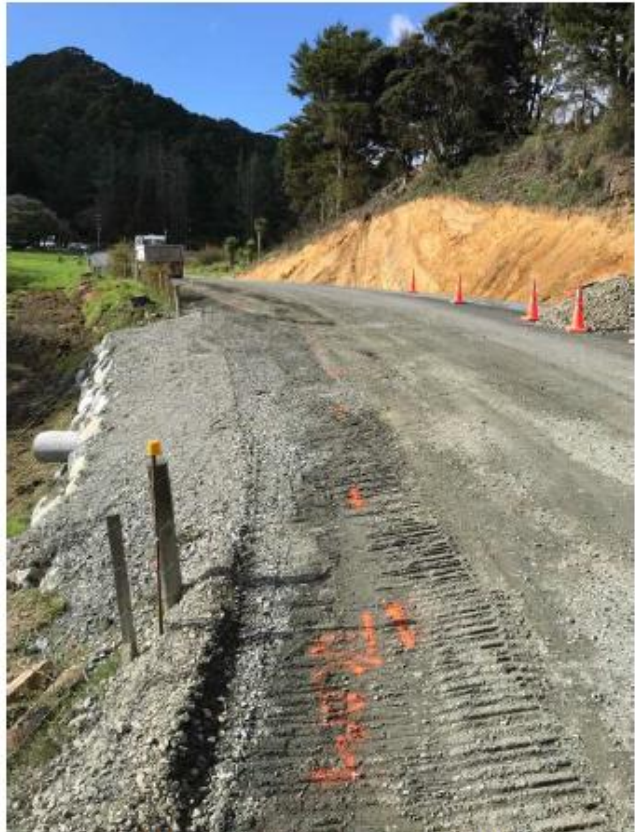
Figure 9: Section 5 Rock wall construction
