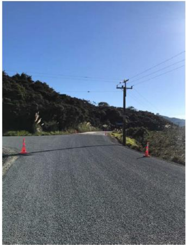
Figure 3: West Coast Rd Section C Seal Complete
