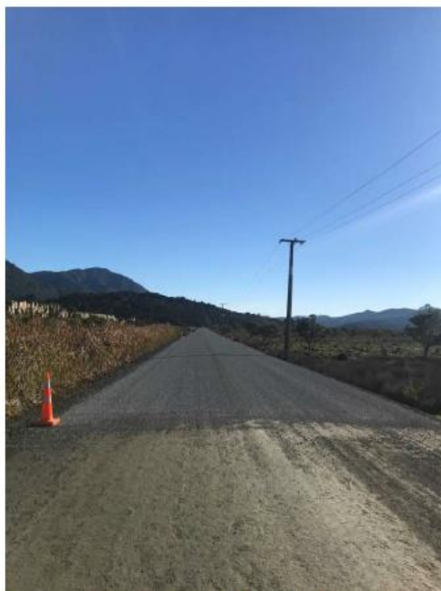
Figure 1: West Coast Rd Section C Seal Complete
