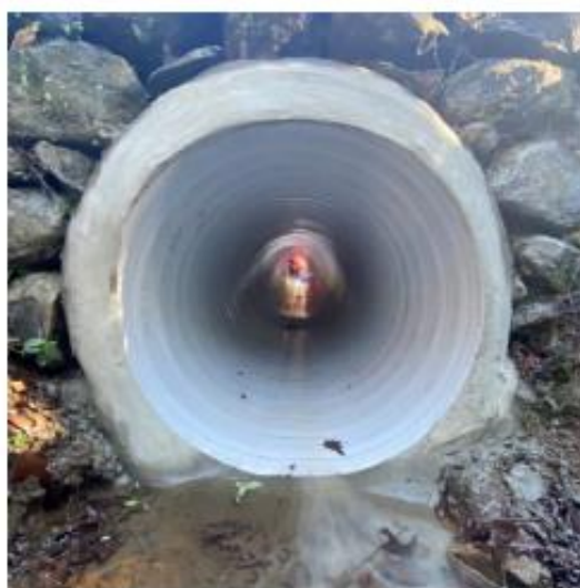
Waimate North Rd – Culvert Lining (Before and After)
