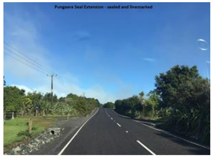
Pungaere Road/Seal Extension
