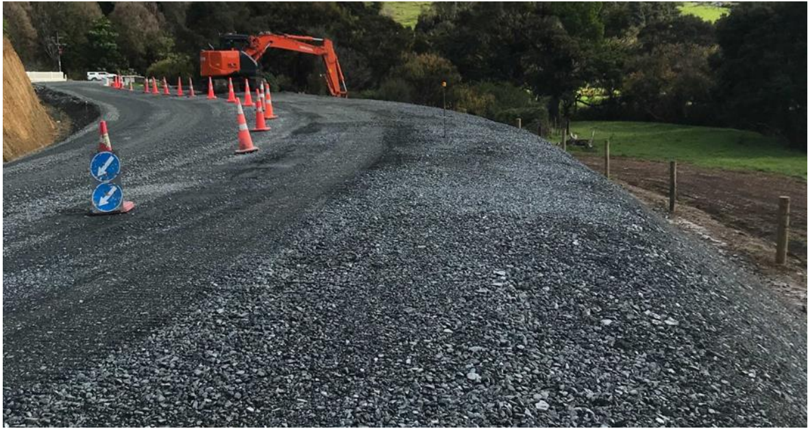
Shoulder support at Peria on Section 5
