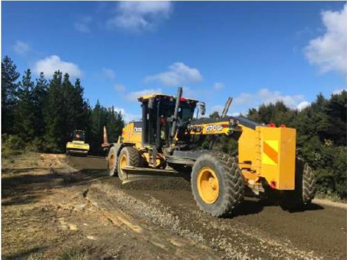
Figure 18: Spirits Bay Rd Heavy Metal Overlay
