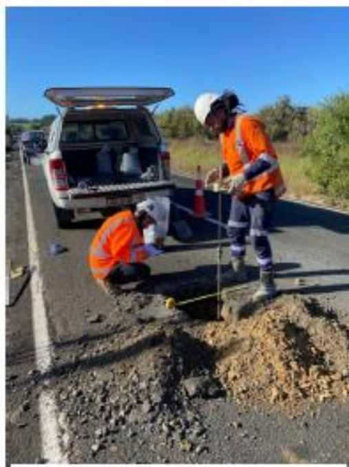
Waikare Rd Rehab – Test Pits
