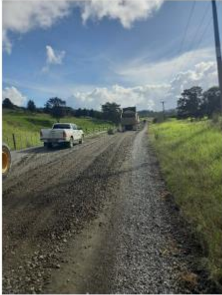
Horeke Rd – Heavy Metalling
