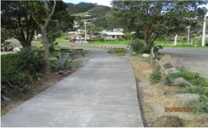
Ahipara Foreshore/New Footpaths
