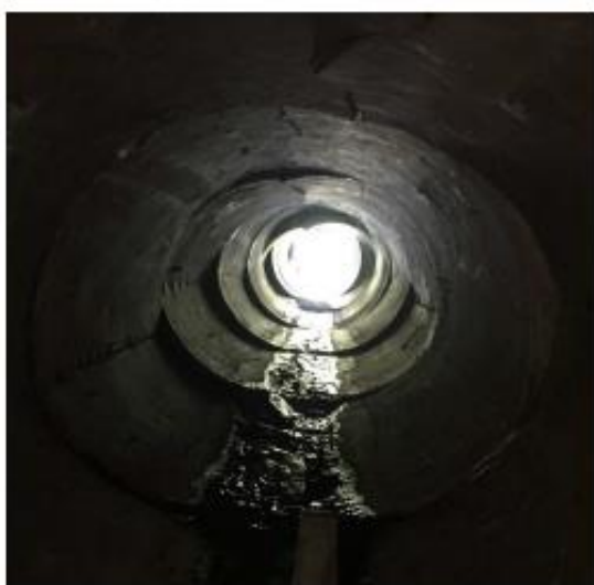
Waimate North Rd – Culvert Lining (Before and After)
