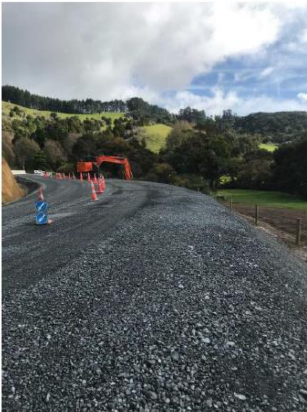
Figure 8: Section 5 Corner widening
