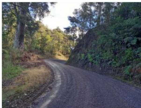
Whangae Rd – Maintenance Metalling
