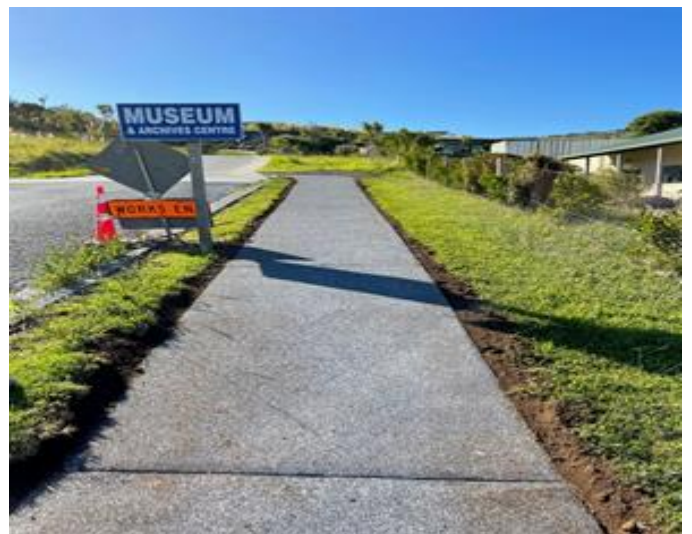
Opononi Footpath - Waianga Place/Footpath construction
