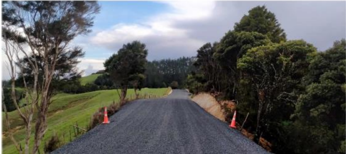
Ruapekapeka Rd – Unsealed Section widening and overlay
