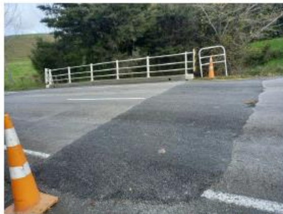
Ngapipito Rd – Bridge Approaches
