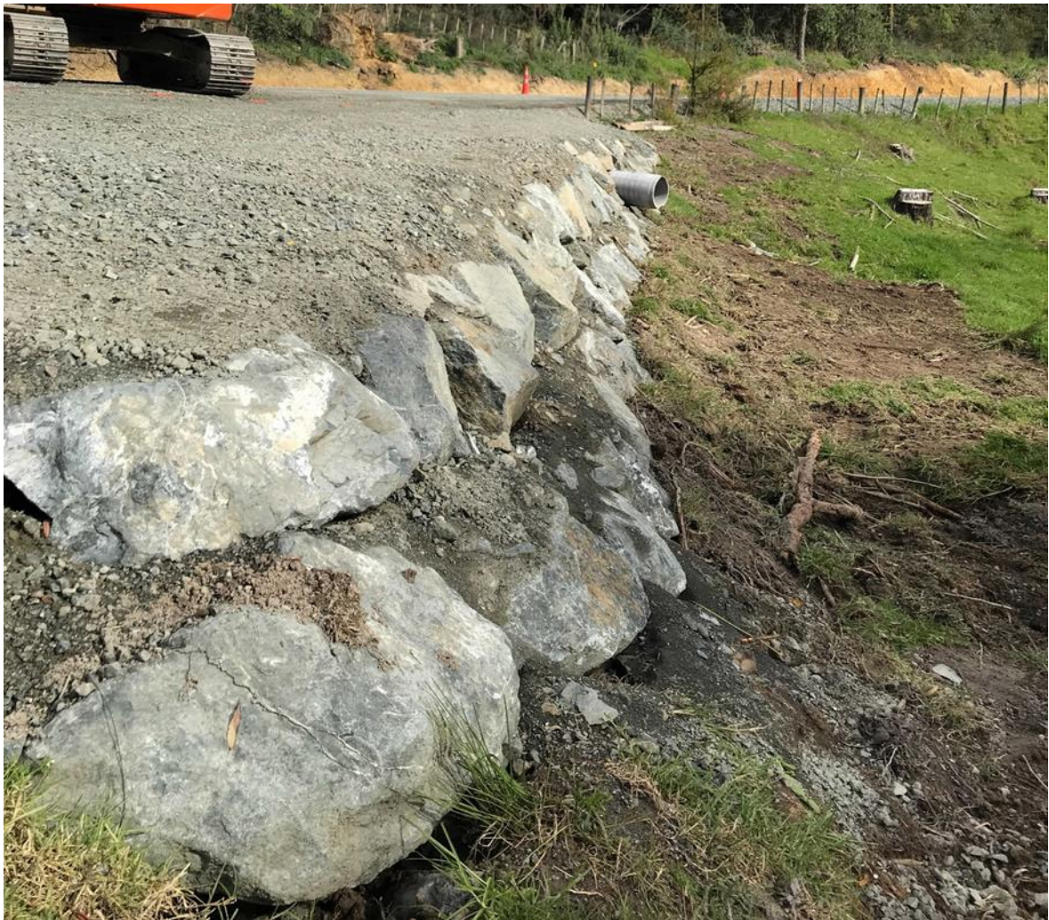
More Section 5 rock wall at Peria
