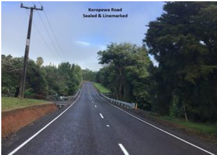
Koropewa Road/Seal Extension
