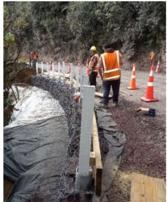
Waikare Rd – Preventative Maintenance (in progress)
