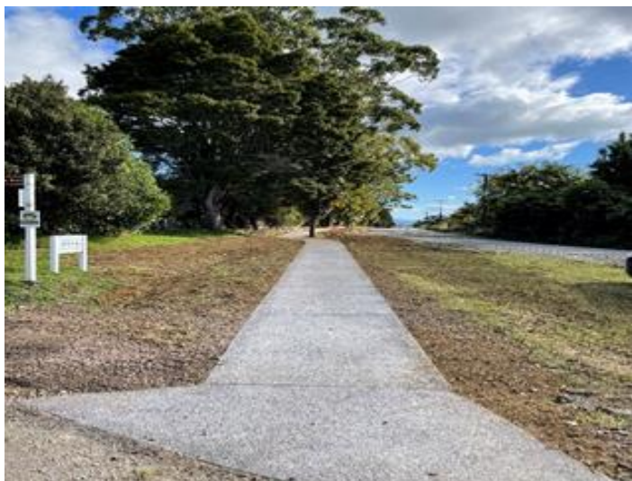
Horeke Road to Cemetery 294-330/Footpath construction
