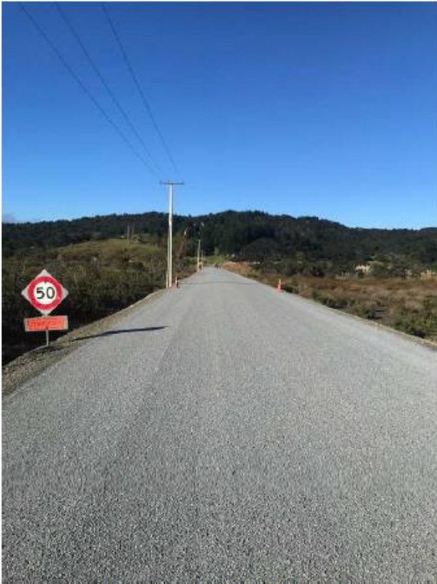
Figure 2: West Coast Rd Section C Seal Complete
