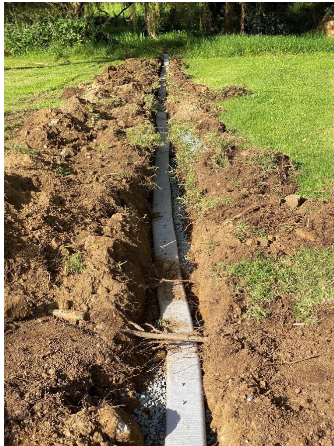
Gateway students getting shown the mega-flow drainage pipe and how it works with the layers of filter cloth, metal and soil by the contractor from Far North Roding doing the sub soil drainage work at Awanui Park.
