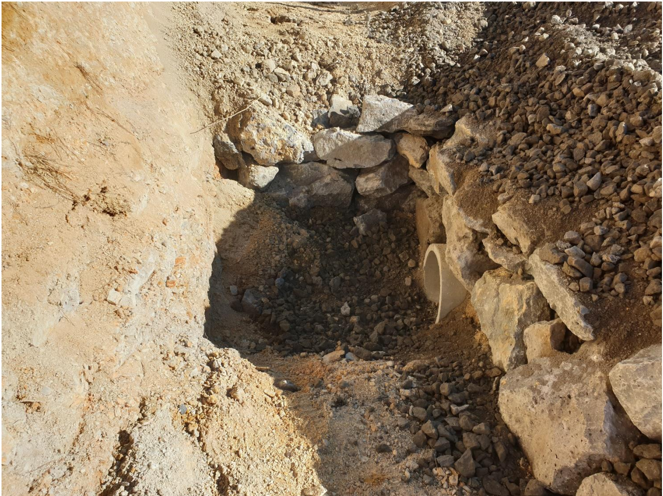
Ngapipito Road drainage and culvert upgrades are complete on sections 1 and 2
