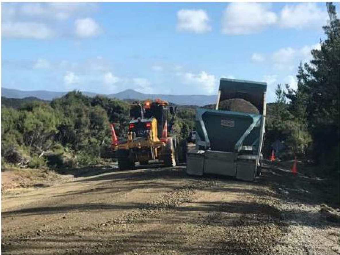
Figure 19: Spirits Bay Rd Heavy Metal Overlay
