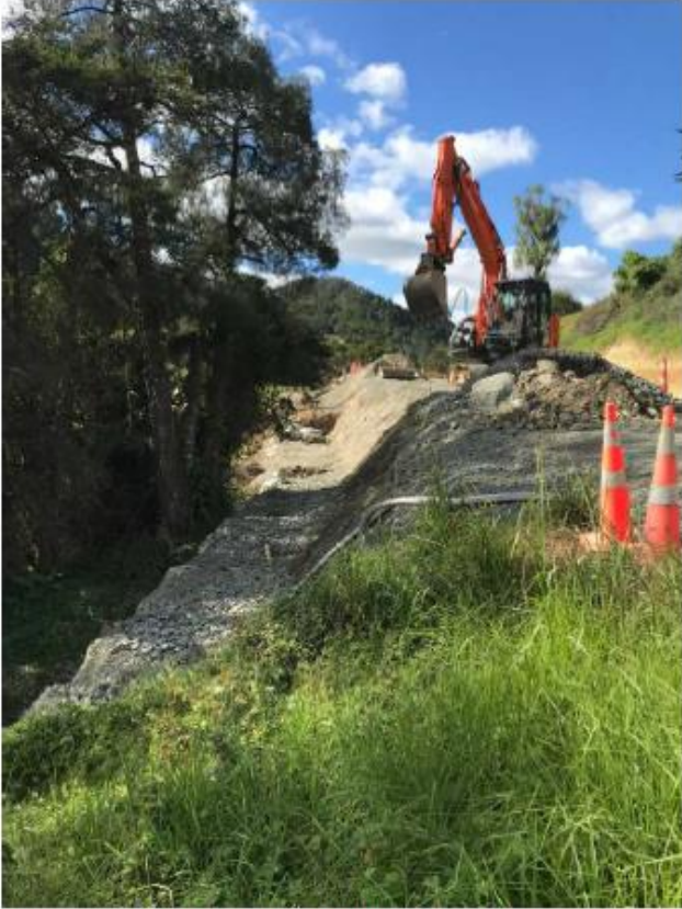
Figure 6: Section 5 Rock wall construction
