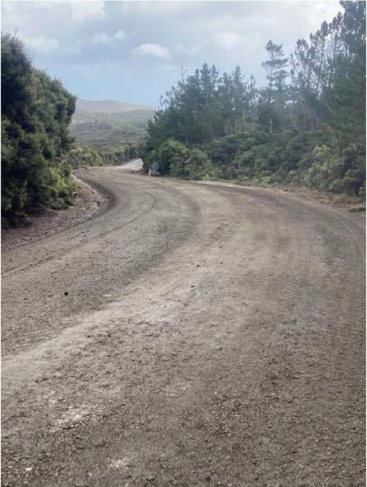
Figure 17: Spirits Bay Rd Heavy Metal Overlay
