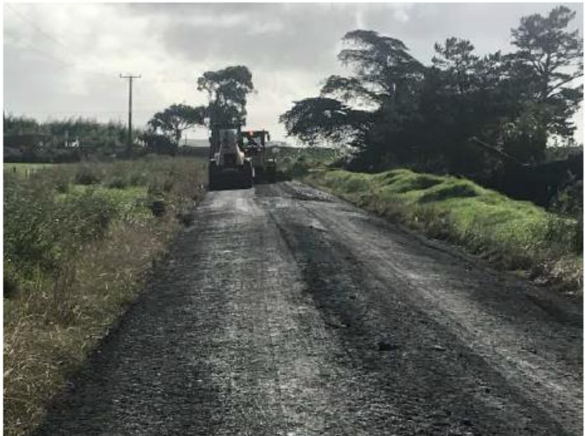
Figure 21: Brass Road Heavy Metal Overlay
