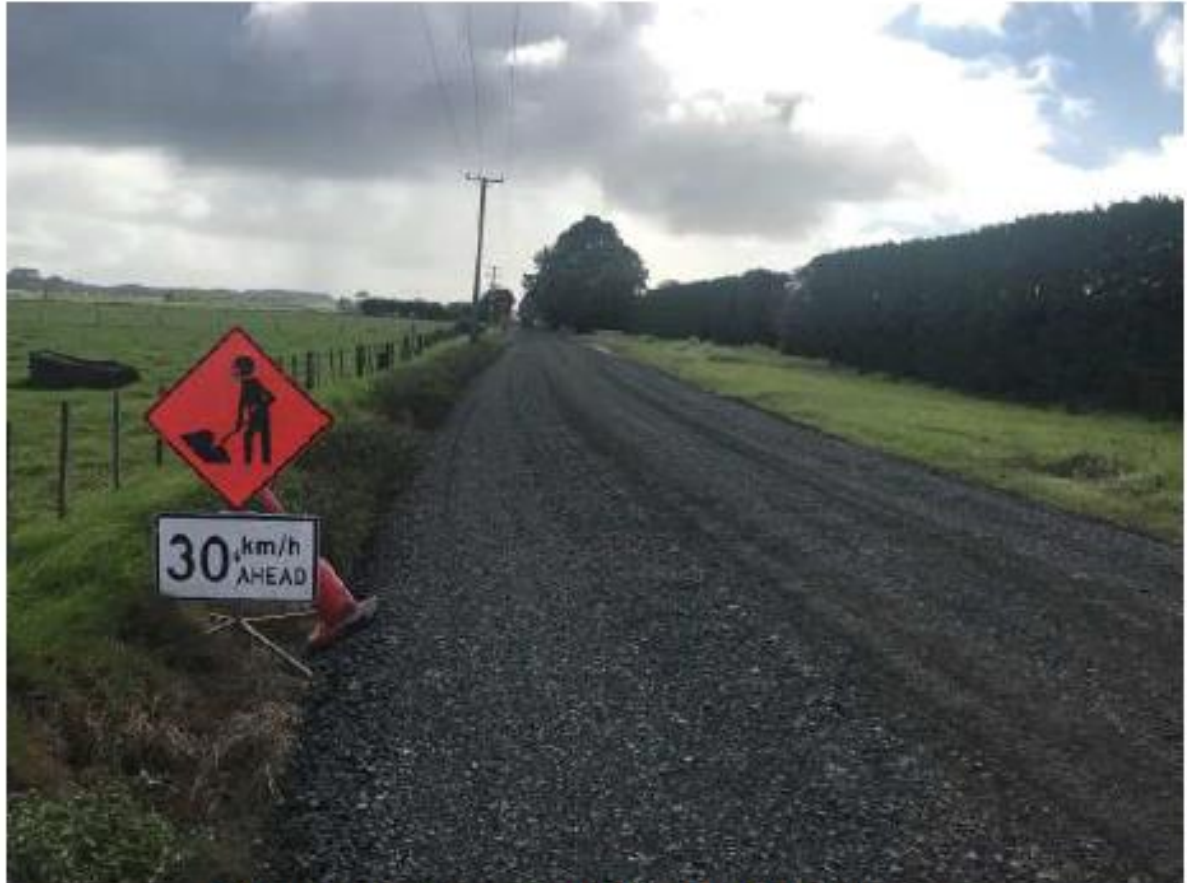
Figure 20: Brass Road Heavy Metal Overlay
