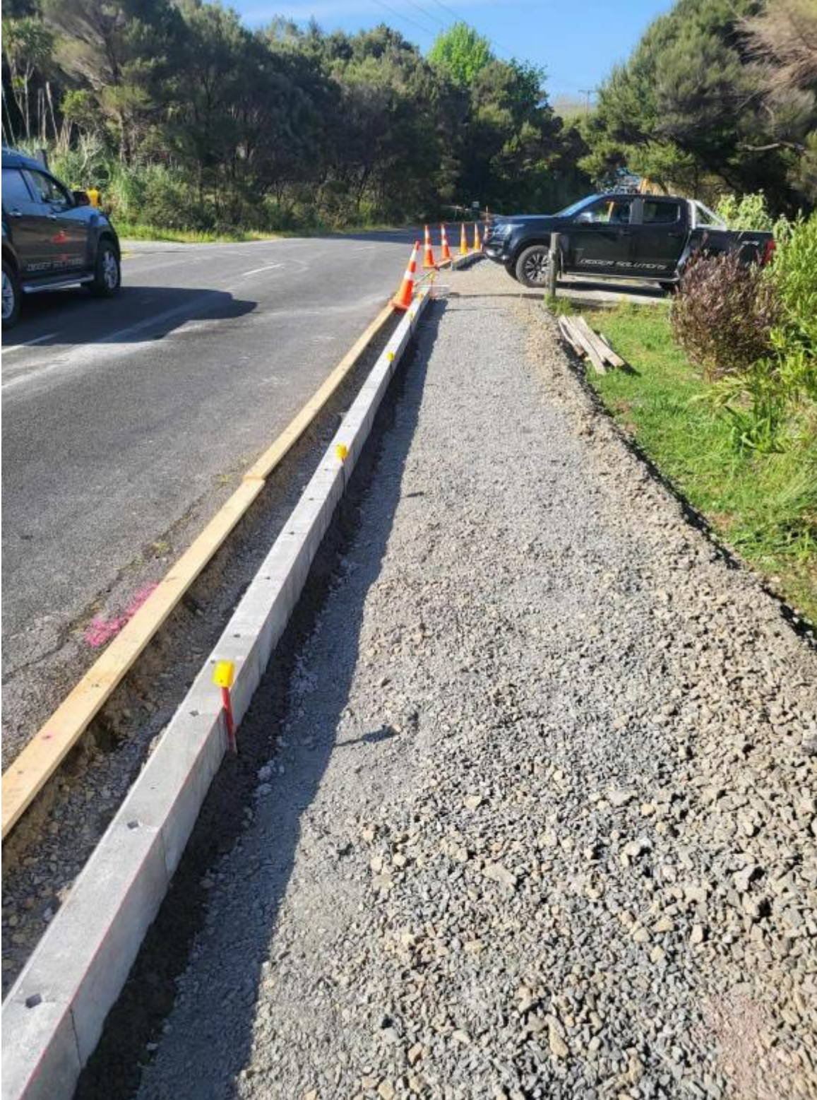
Cable Bay Block Road New Footpath Prep
