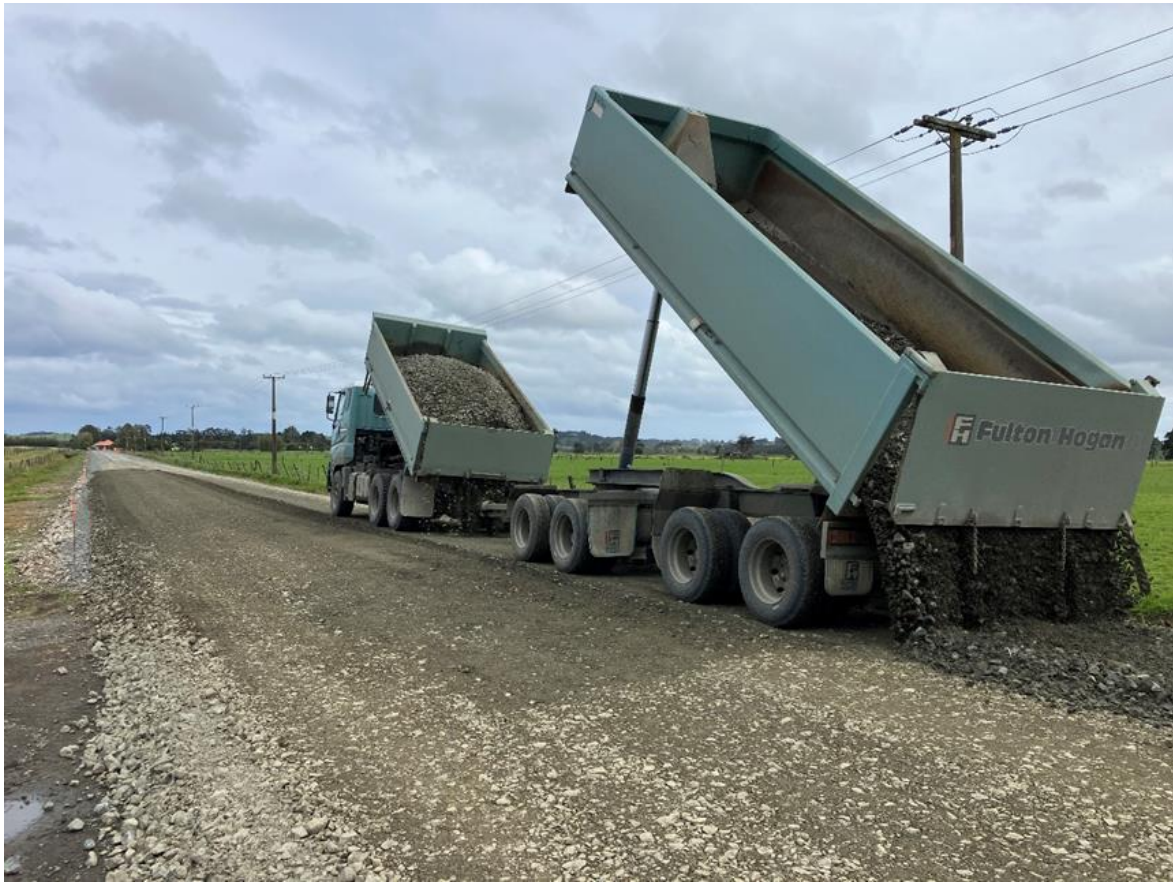
Gill Rd Pavement Rehabilitation Overlay
