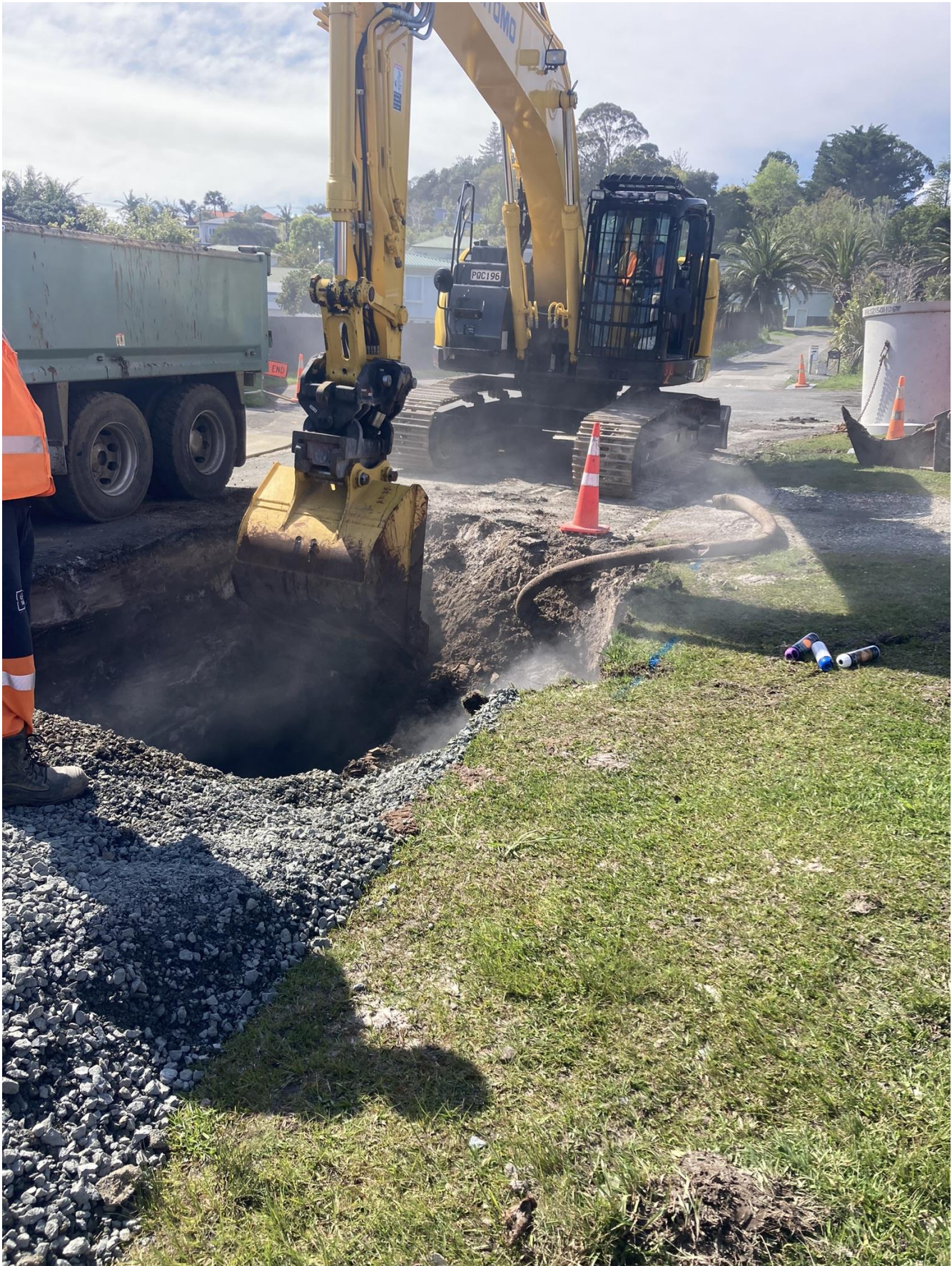
Sommerville Ave SW Upgrade Installation
