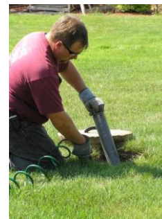
Lifting and hosing down effluent outlet filter
