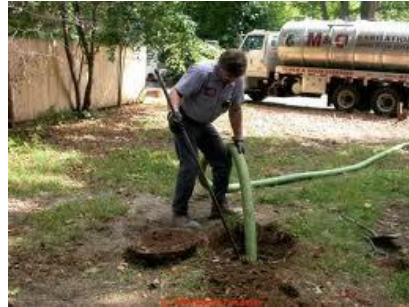
Septic tank pumpout
