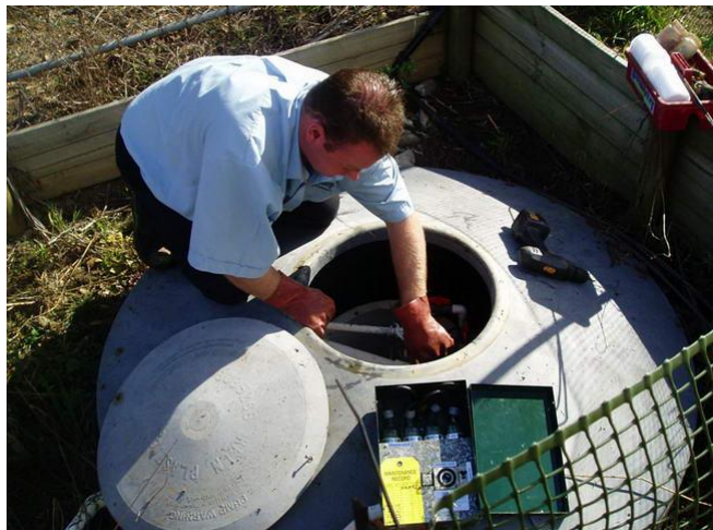
Servicing an advanced wastewater treatment unit
