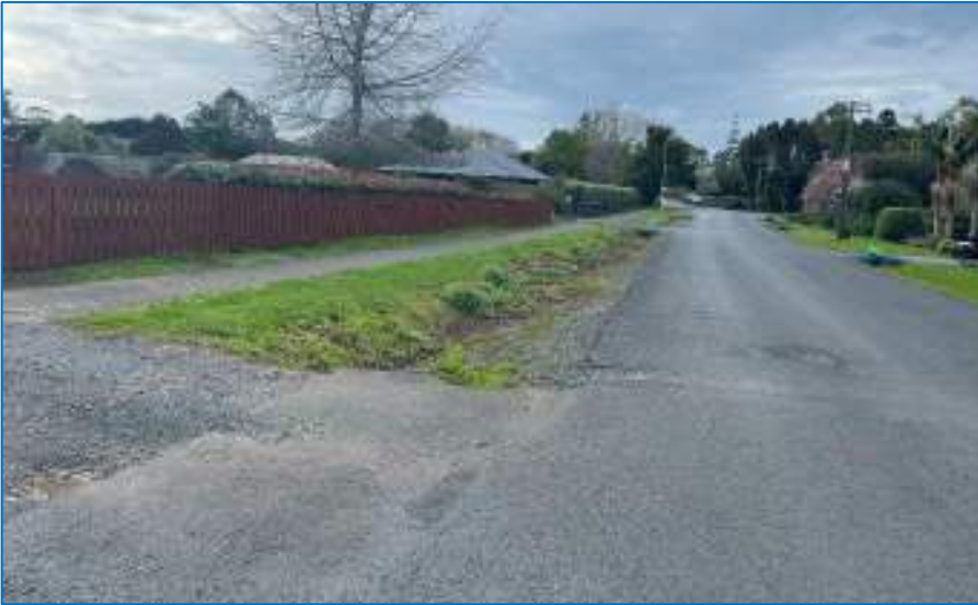
Photograph 1: Subject site's road frontage to Limelight Lane, showing the existing vehicle crossing to Lot 3. The shared vehicle crossing to Lots 1 and 2 will be formed at the northern end of the road frontage at the end of the fence.
