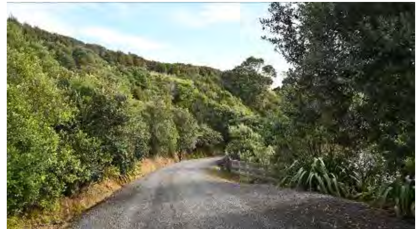
Photograph 2: The heavily vegetated slopes associated with the access drive as it descends towards the houses on the property. The contrast with the stark face that existed here in 2015 when the drone images found in Attachment Four is very marked.
