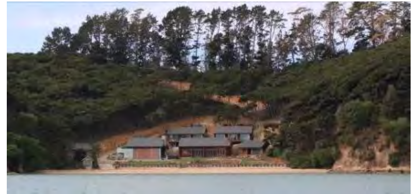
Photograph 8: A recently constructed house on the opposite coast, demonstrating the adverse effects of a building crowding the shore, the loss of naturalness that results from conventional seawalls and boat ramps, and considerable unmitigated earthworks. It is these sorts of impacts that the proposal has sought to avoid in its scale and the way that it is configured.
