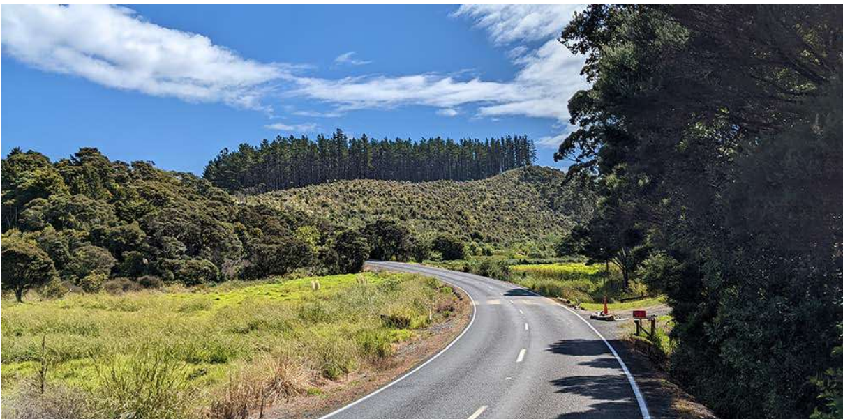
Photograph 3 Looking north-west from outside 515 Rawhiti Road towards the remaining pines along the ridge, with revegetation below them
