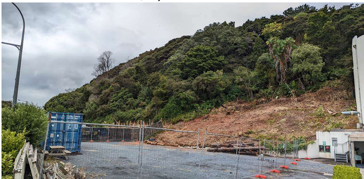
Photograph 6 Earthworks and construction activities on numbers 120-128 in March 2024
