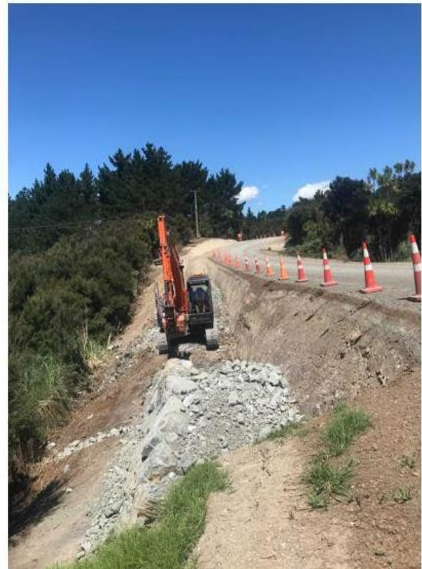
Figure 2: Rock wall construction
