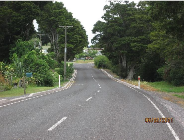
Porotu Road/ Seal extension
