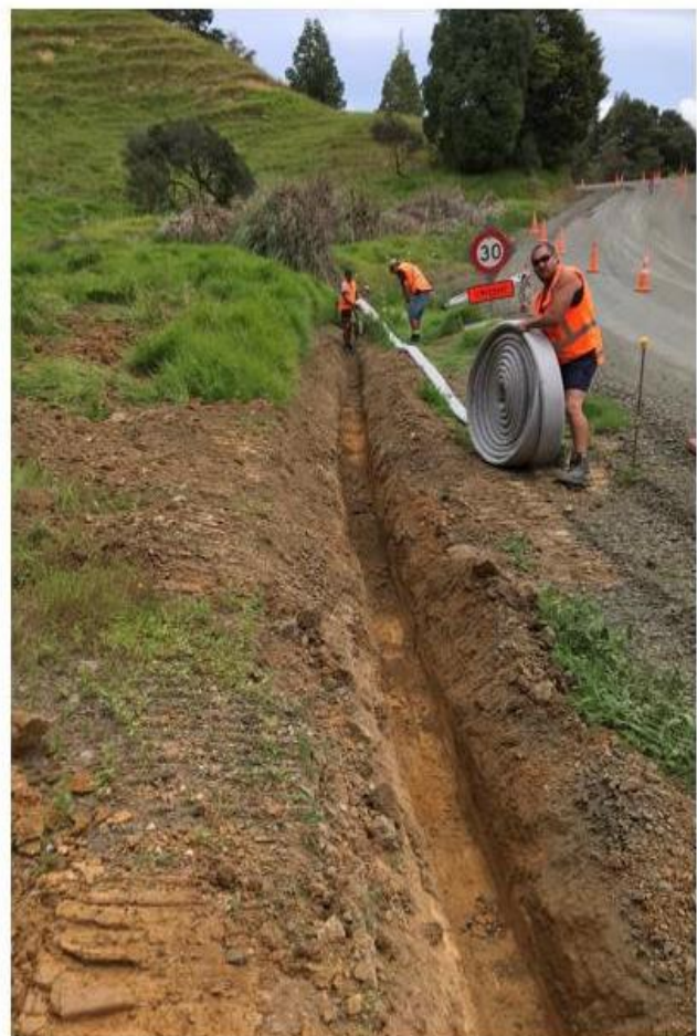
Figure 2: Laying subsoil in water table.
