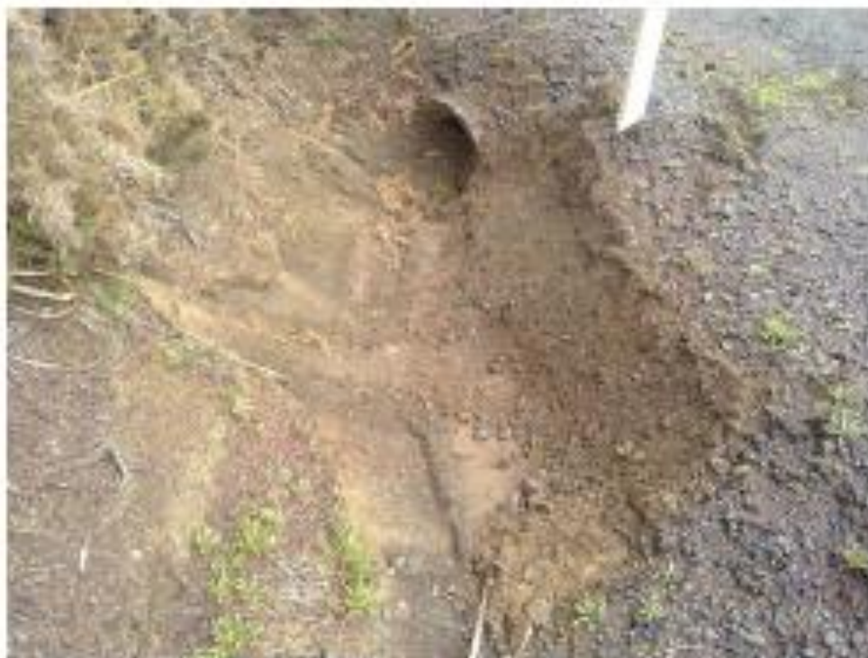
Kelly Rd - Routine Culvert Clearing
