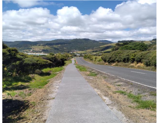
Signal Station Road/ Concrete Footpath
