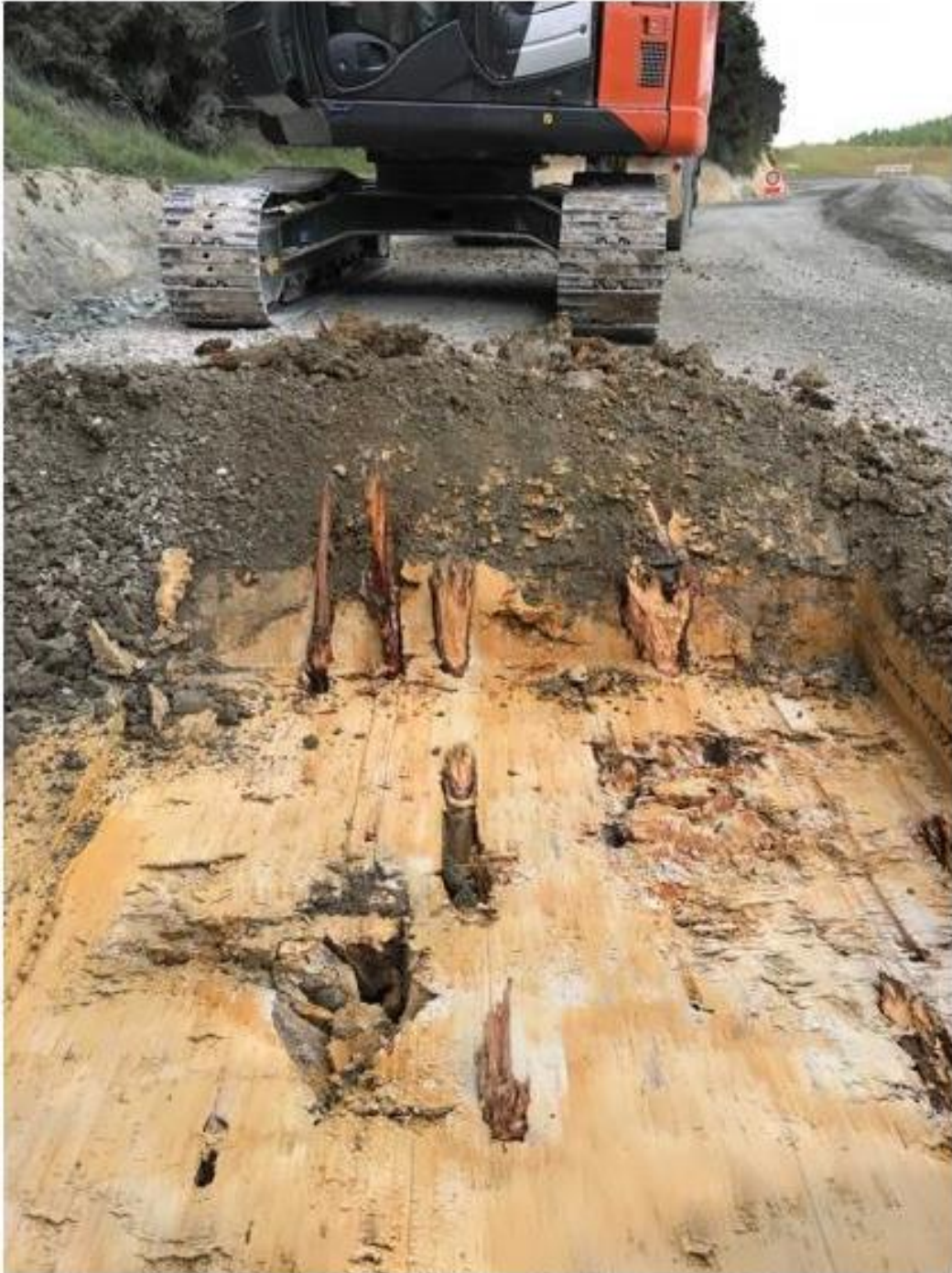
Figure 5: Dig out on soft patch in Section Two
