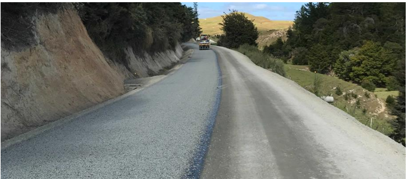
Sealing in progress at Peria on Section 2
