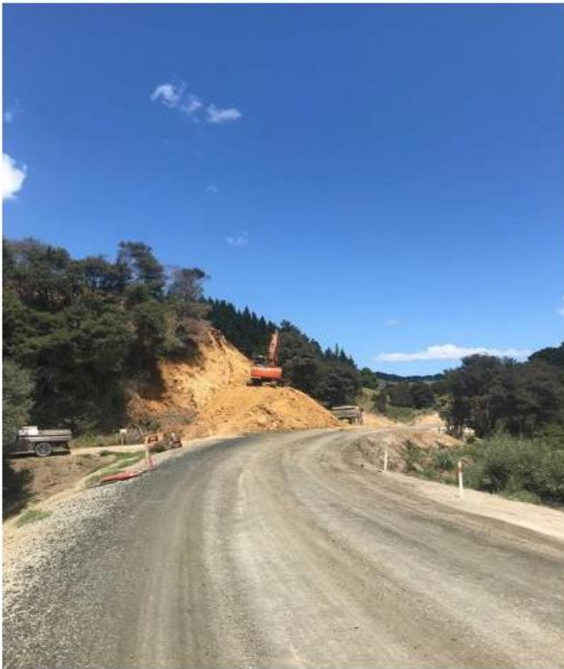
Figure 4: Clearing and corner widening in Section Four
