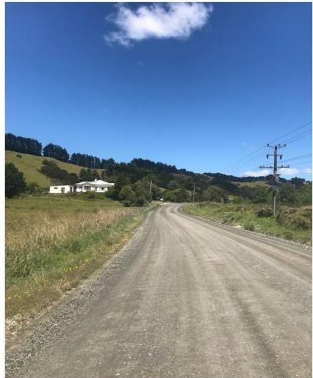
Figure 5: Dust suppressant completed in Sections Four and Five
