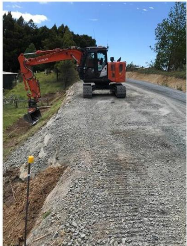
Figure 6: Rock wall complete in Section Three
