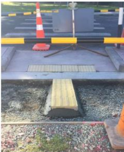
Tactile and footpath installation underway on Otiria Rd, Moerewa
