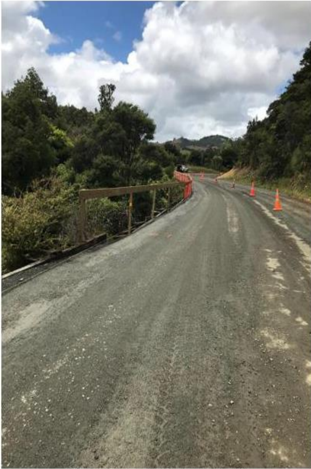
Figure 3: Temporary edge protection rail.
