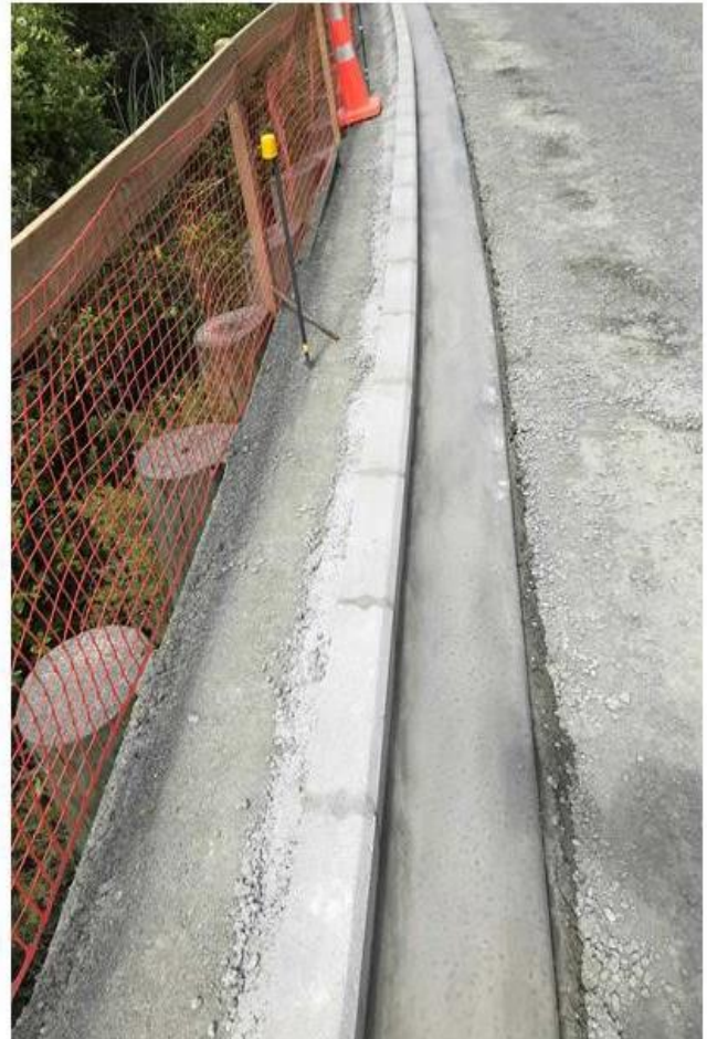
Figure 2: Completed kerb and channel at ch510-575.
