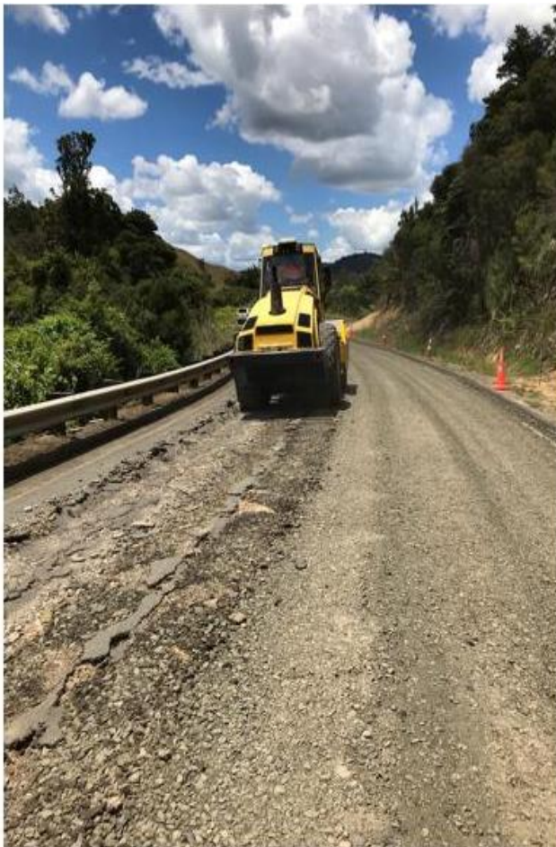
Figure 1: The ripped up pavement being compacted.
