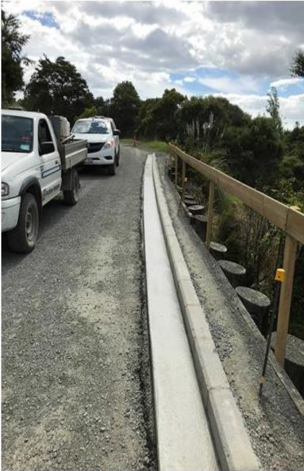
Figure 1: Completed kerb and channel at ch510-575.
