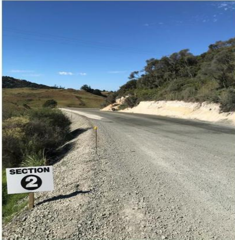
Figure 1: Section Two ready for seal
