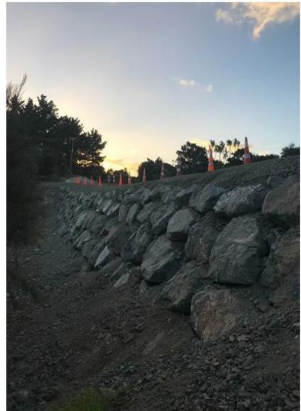
Figure 2: Rock wall construction complete
