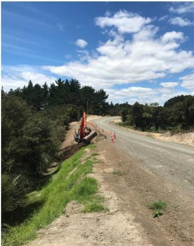
Figure 1: Construction of rock wall.
