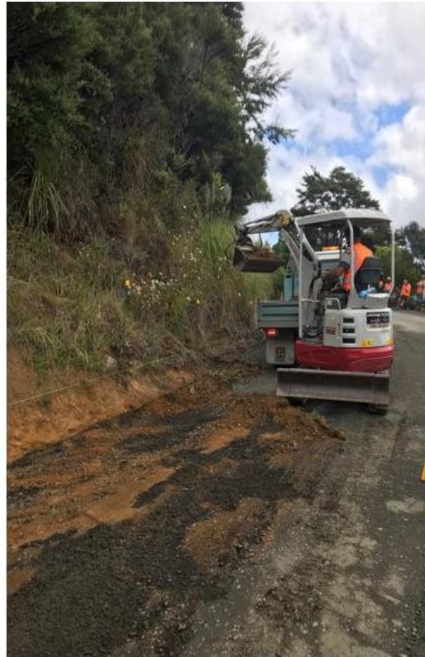
Figure 4: prepping for kerb.
