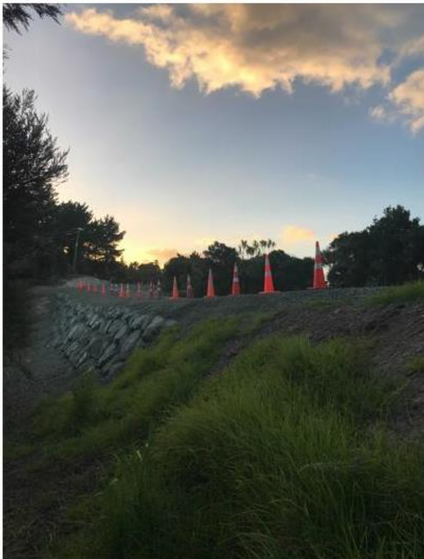
Figure 1: Rock wall construction complete
