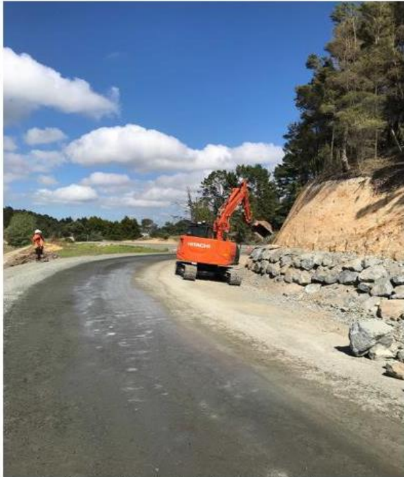
Figure 2: Construction of rock wall in Section 3.
