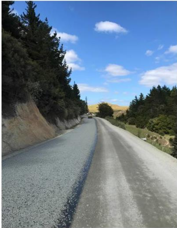
Figure 3: Sealing in progress Section Two
