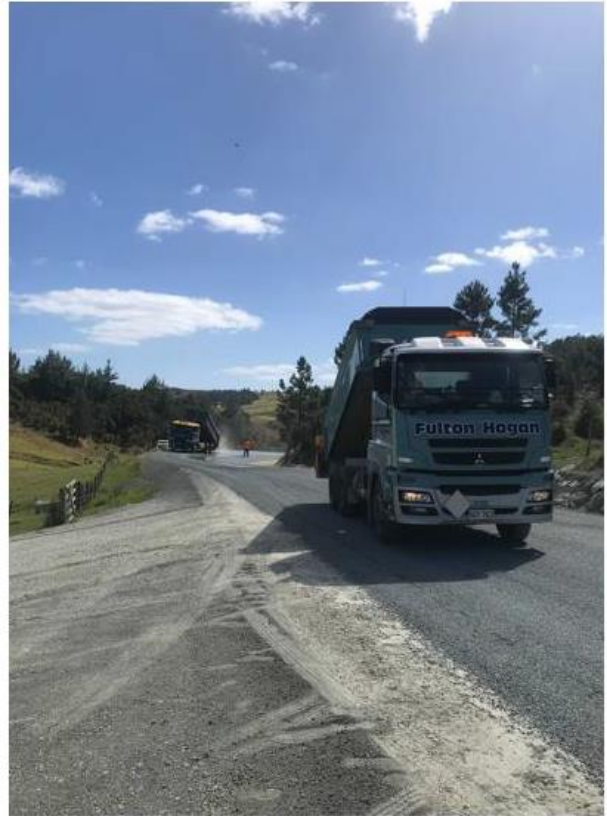
Figure 4: Sealing in progress Section Two
