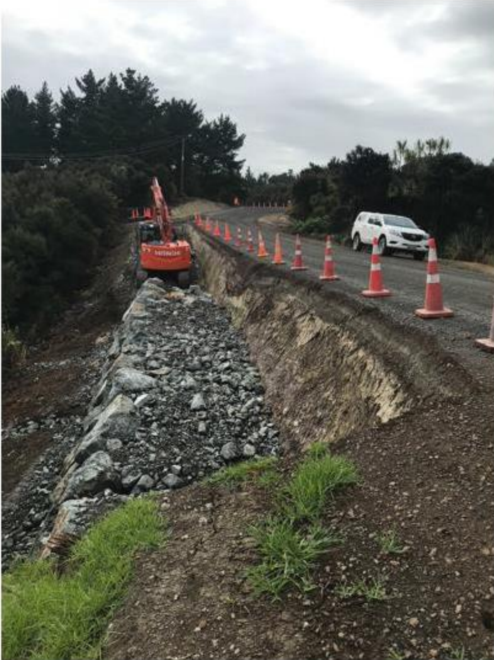
Figure 1: Rock wall construction in progress
