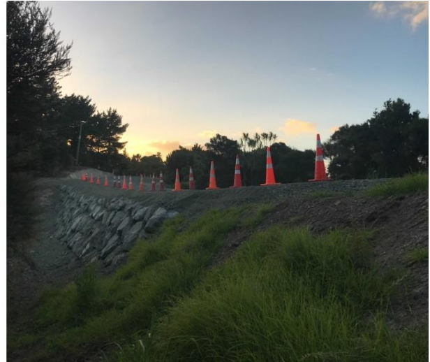
Church Road/Rock wall shoulder support
