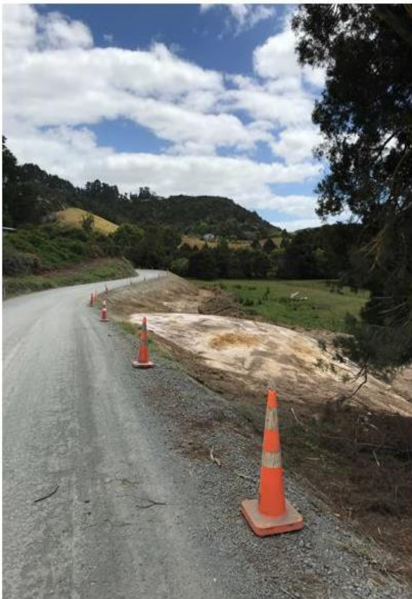
Figure 5: Tip Site #5 ready for CTW from the end of Section Five
