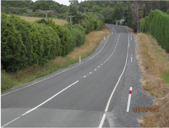
Pungaere Road/ Rehab
