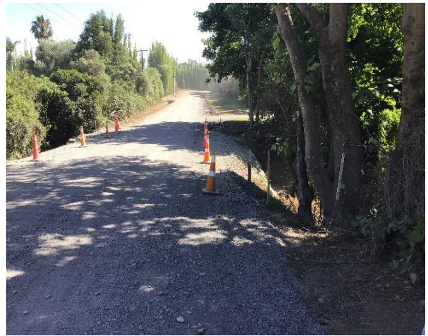
Koropewa/ Culvert widening
