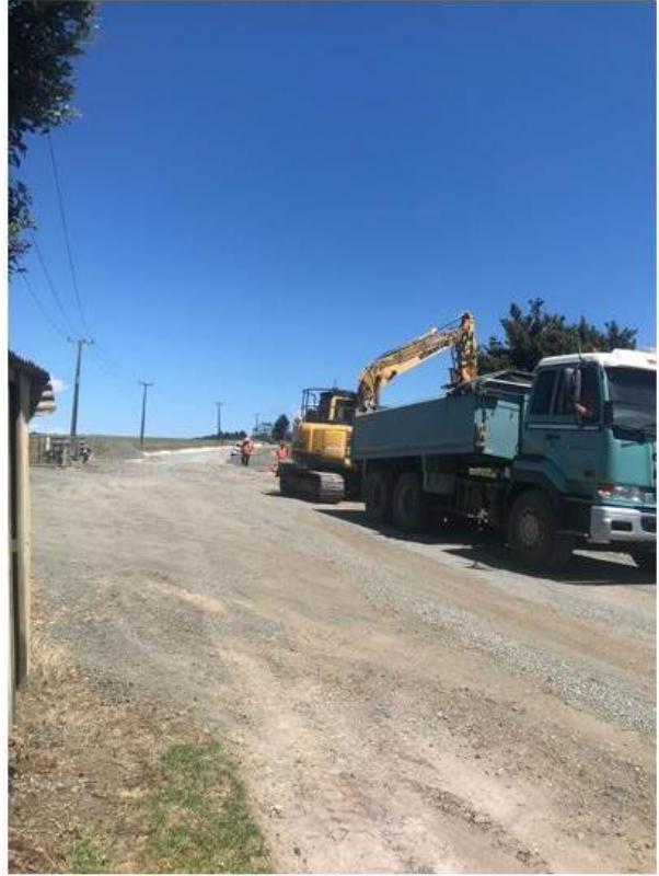
Figure 5: Culvert replacements in progress
