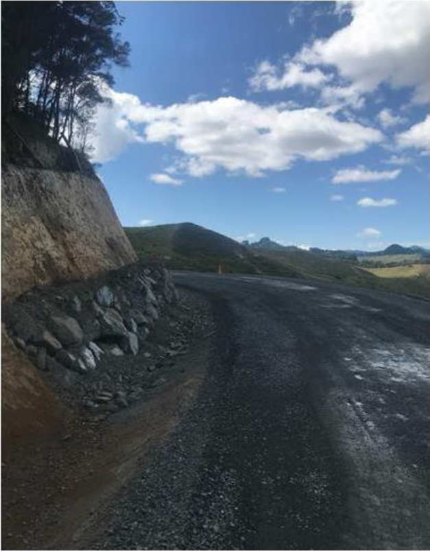
Figure 6: Corner widening and rock wall completed in Section 3
