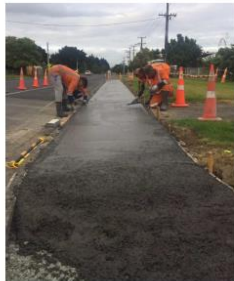
Tactile and footpath installation underway on Otiria Rd, Moerewa
