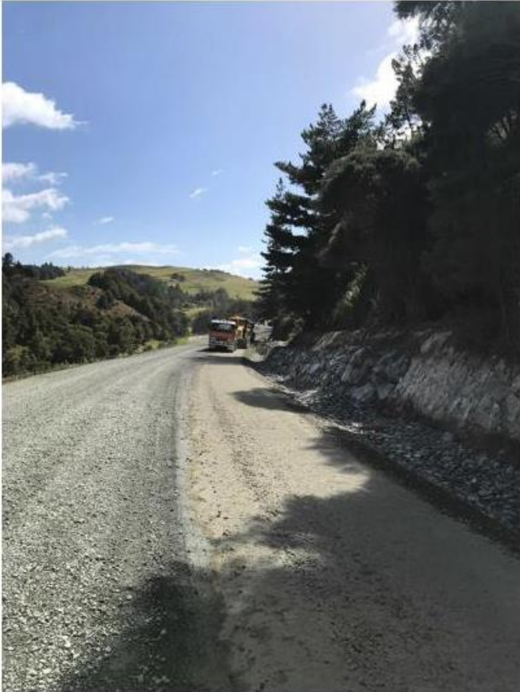
Figure 1: Stabilising in progress Section Two
