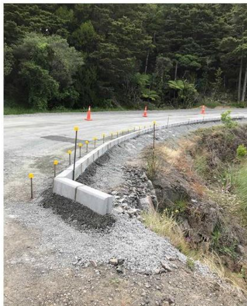
Figure 1: Completed kerb and channel at ch510-575.
