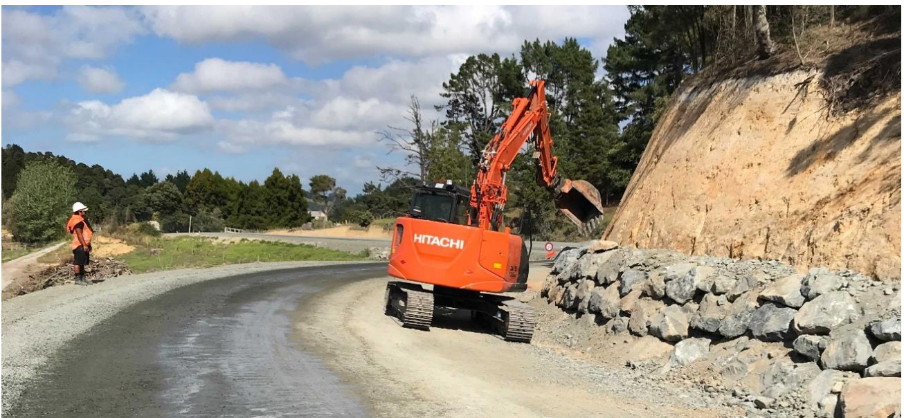
Construction of rock wall in Section 3.
