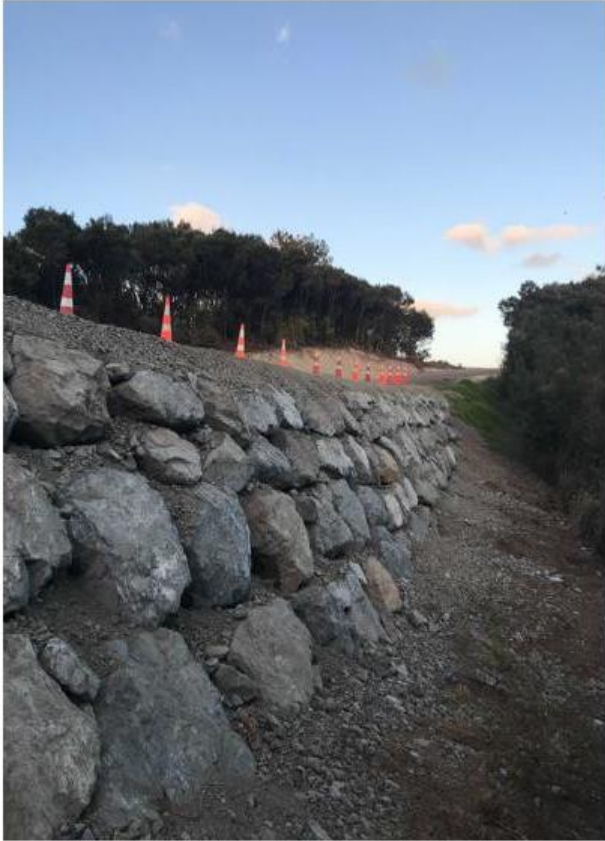
Figure 3: Rock wall construction complete
