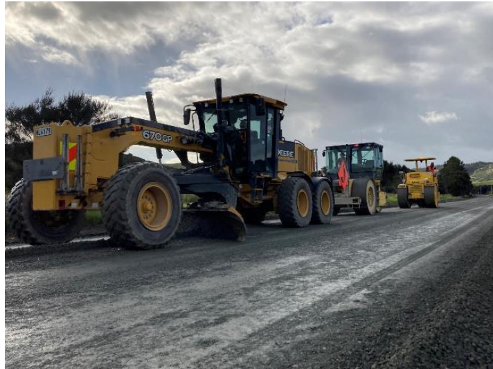
Figure 16: Parapara- Toatoa Rd Pavement Stabilising
