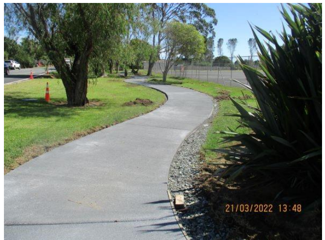
South Road – connection to Te Hiku Car park
