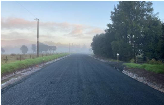
Figure 12: Parapara-Tootoa Rd Pavement Overlay
