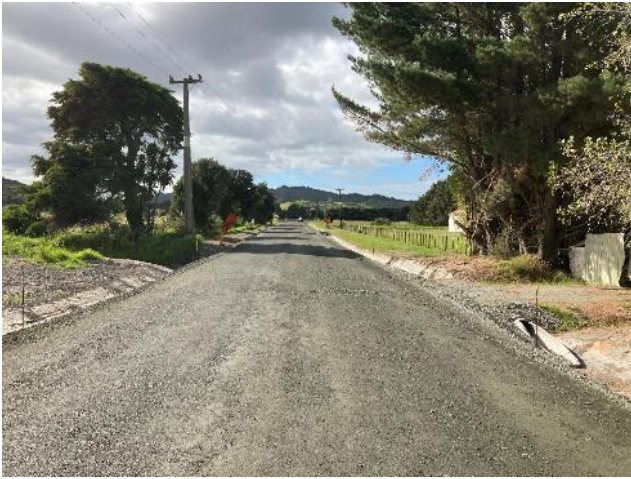
Figure 10: Parapara-Tootoa Rd Pavement Overlay
