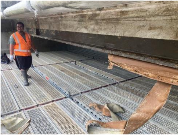
Figure 4: Peria Rd Bridge Beam Repairs
