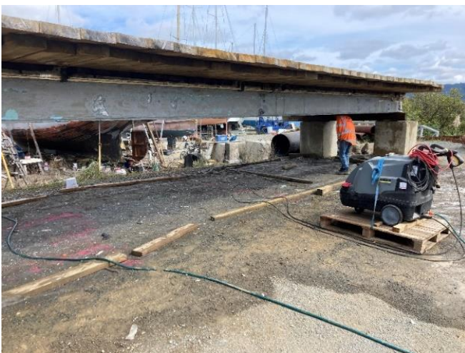
Puhata Road Bridge D50 Replacement
