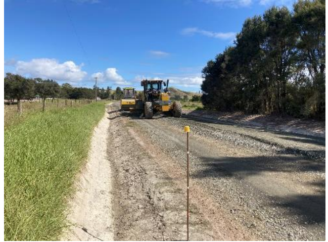
Figure 11: Parapara-Tootoa Rd Pavement Overlay
