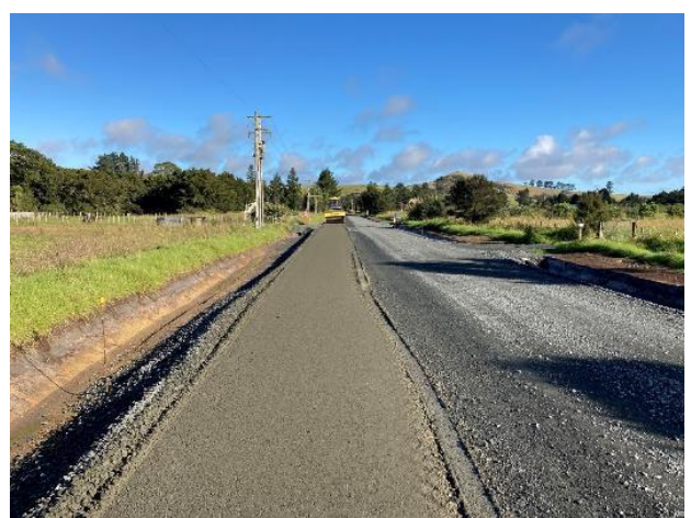
Figure 15: Parapara-Tootoa Rd Pavement Stabilising
