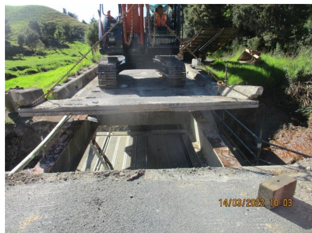
Figure 7: Peria Rd Bridge Deck Replacement
