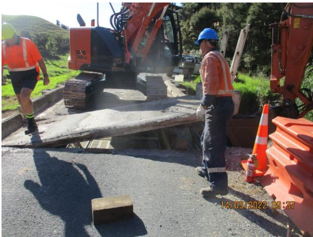
Figure 6: Peria Rd Bridge Deck Replacement
