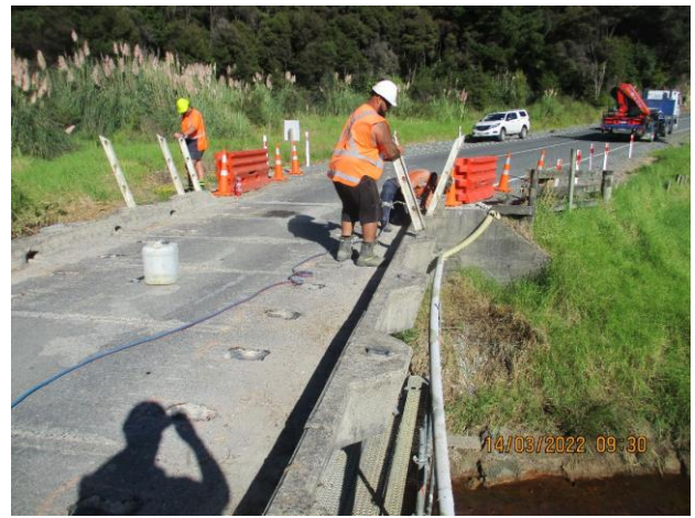
Figure 5: Peria Rd Bridge Deck Replacement
