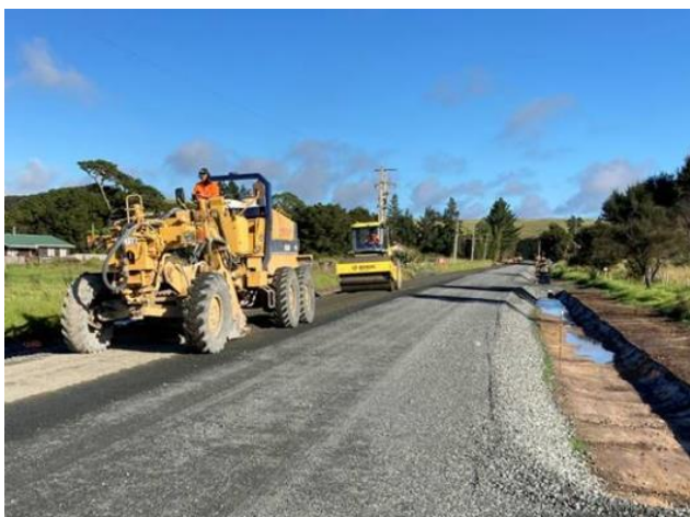
Figure 14: Parapara-Tootoa Rd Pavement Stabilising
