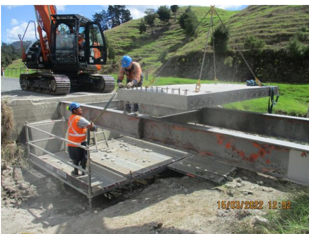
Figure 8: Peria Rd Bridge Deck Replacement
