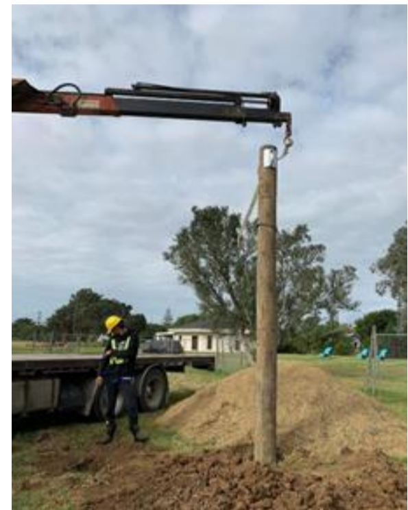
The flying fox installation with the help from local Hiab truck driver, Henry Yates assisting with the substantial posts required for construction of this double flying fox.
