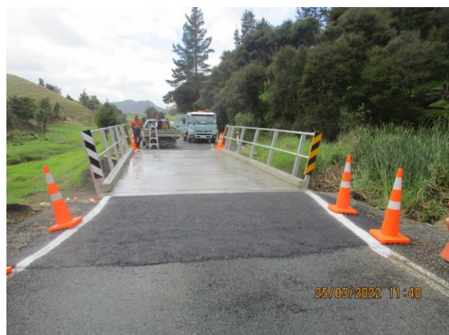
Figure 9: Peria Rd Bridge Deck Replacement
