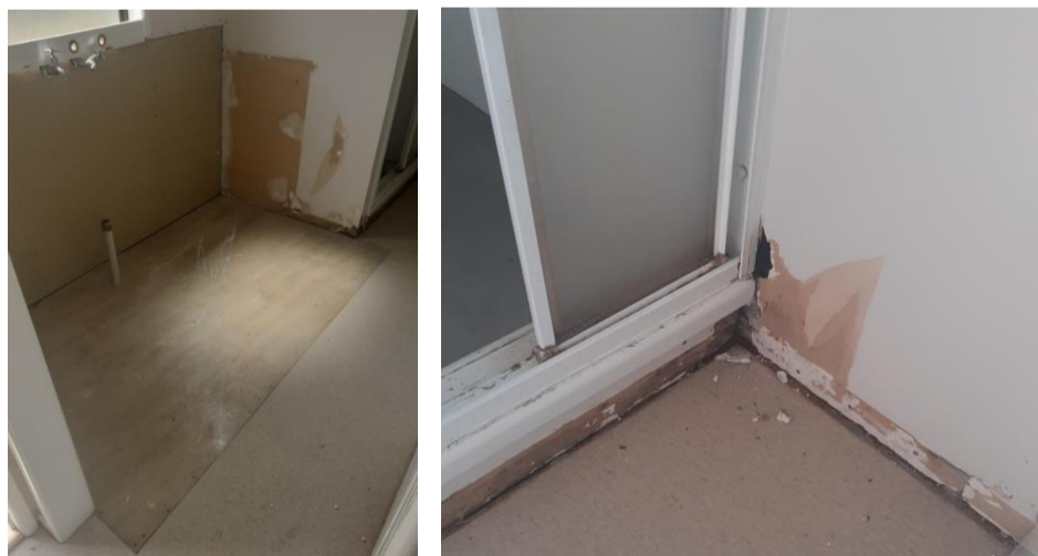
Unit 2, Waima washtub removed, damaged wall lining, and flooring replace
