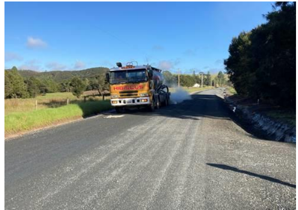
Figure 13: Parapara-Tootoa Rd Pavement Stabilising
