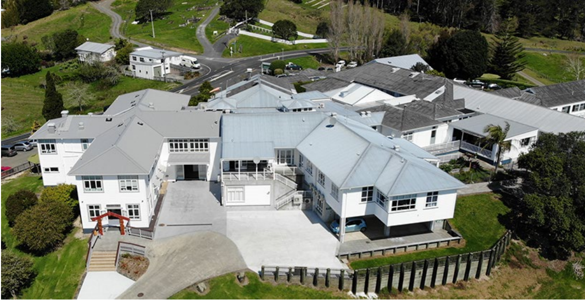
Rawene Hospital (source https://waateanews.com/2021/07/14/rawene-hospital-embraces-rongoa/ )
