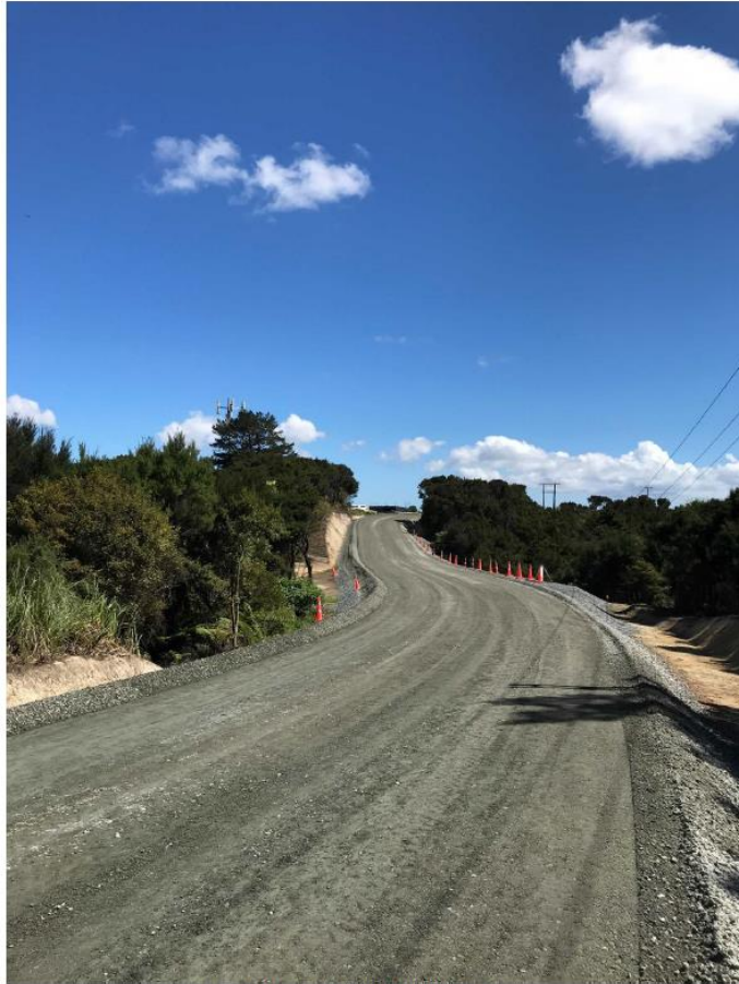
Figure 6: Section One Prepping for seal
