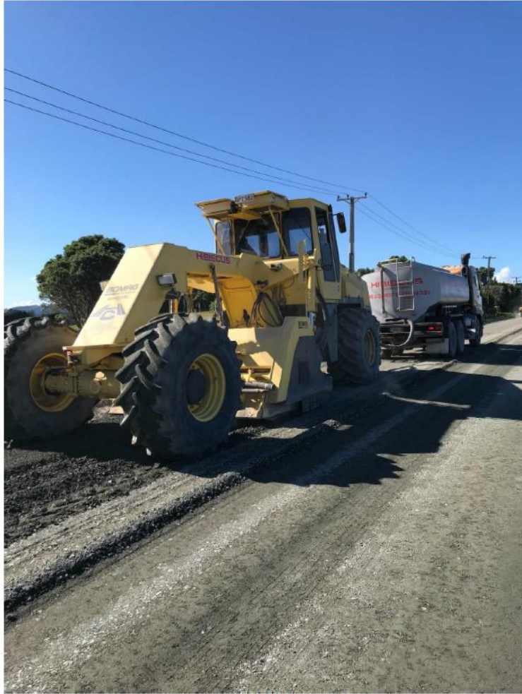
Figure 9: Section Two Stabilising in Progress
