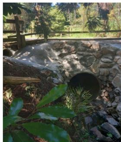
Koranae Rd – Large Concrete Headwall
