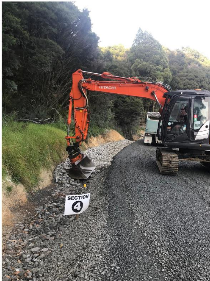
Figure 22: Section Four Scour Protection
