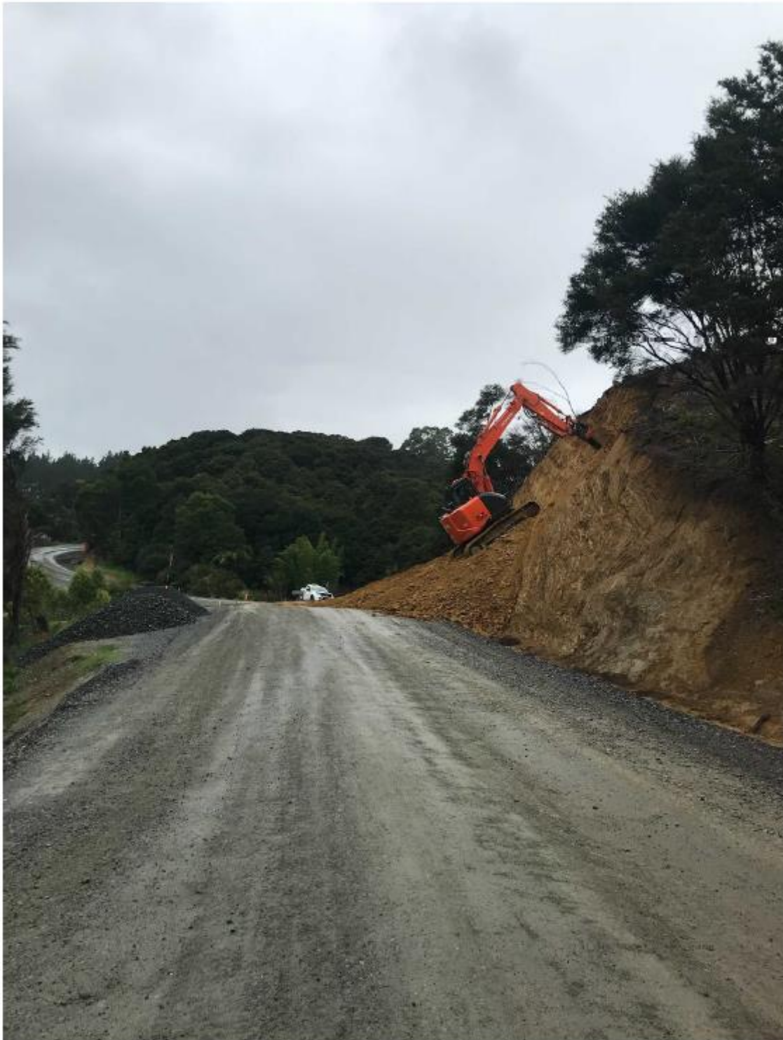
Figure 14: Section Four earthworks in preparation for rock wall
