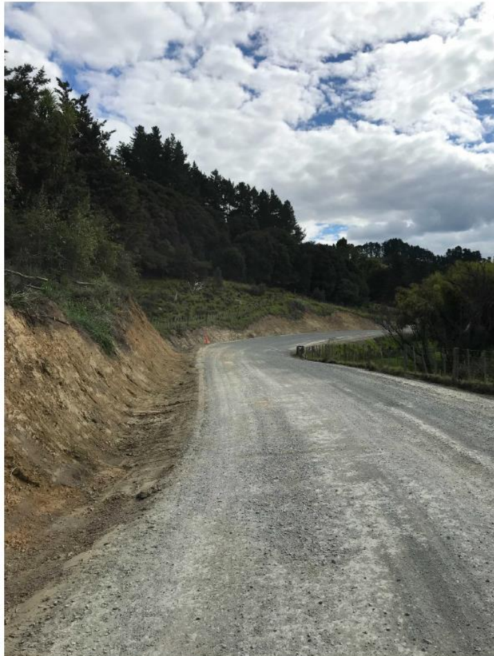
Figure 18: Section Five clearing in progress
