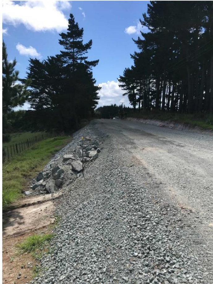
Figure 2: ROQ shoulder widening
