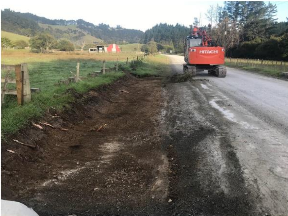
Figure 25: Section Five clearing in progress
