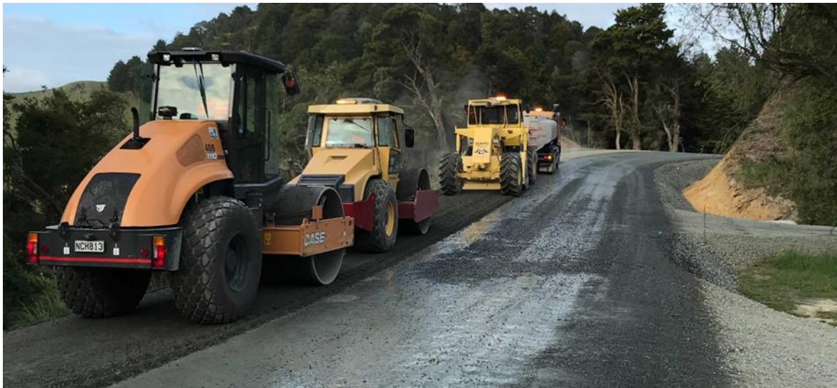
Stabilising in progress at Peria on Section 3
