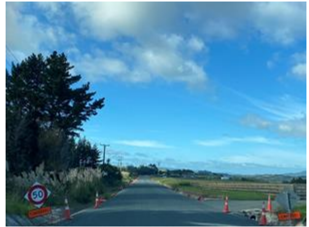
Church Road/Seal Extension first 600m sealing
