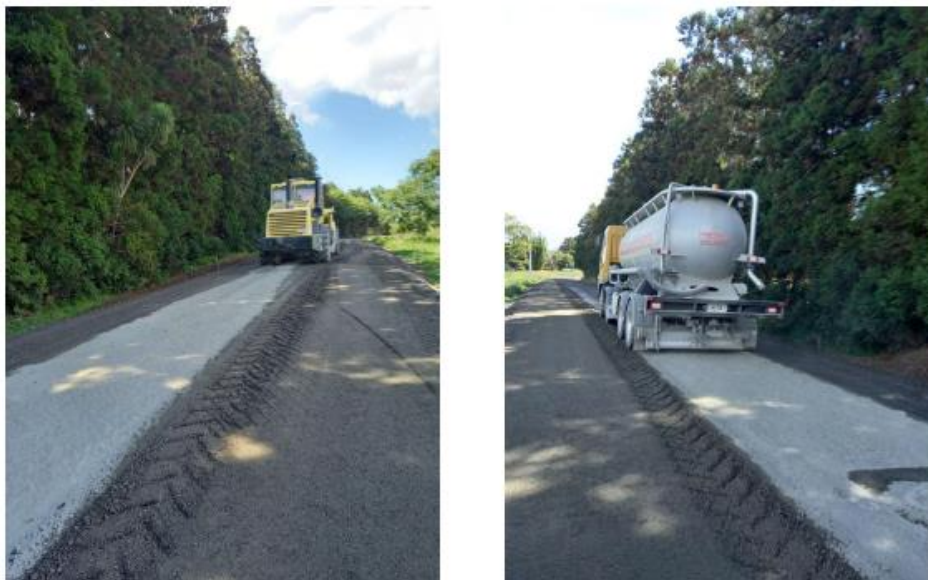
Koropewa Rd – Hibiscus Contractors spreading cement and hoeing
