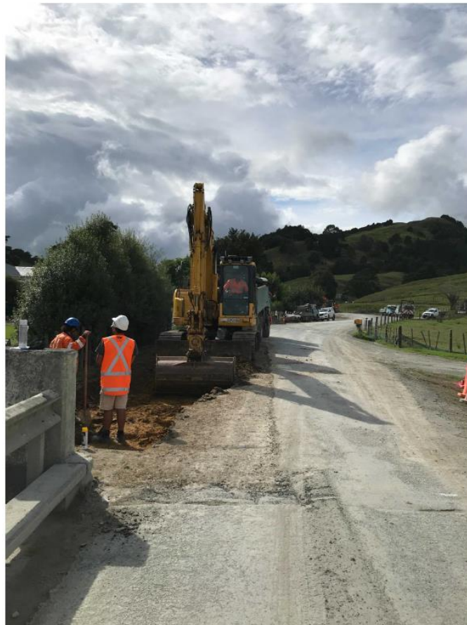
Figure 12: Section Four Bridge Undercut in progress
