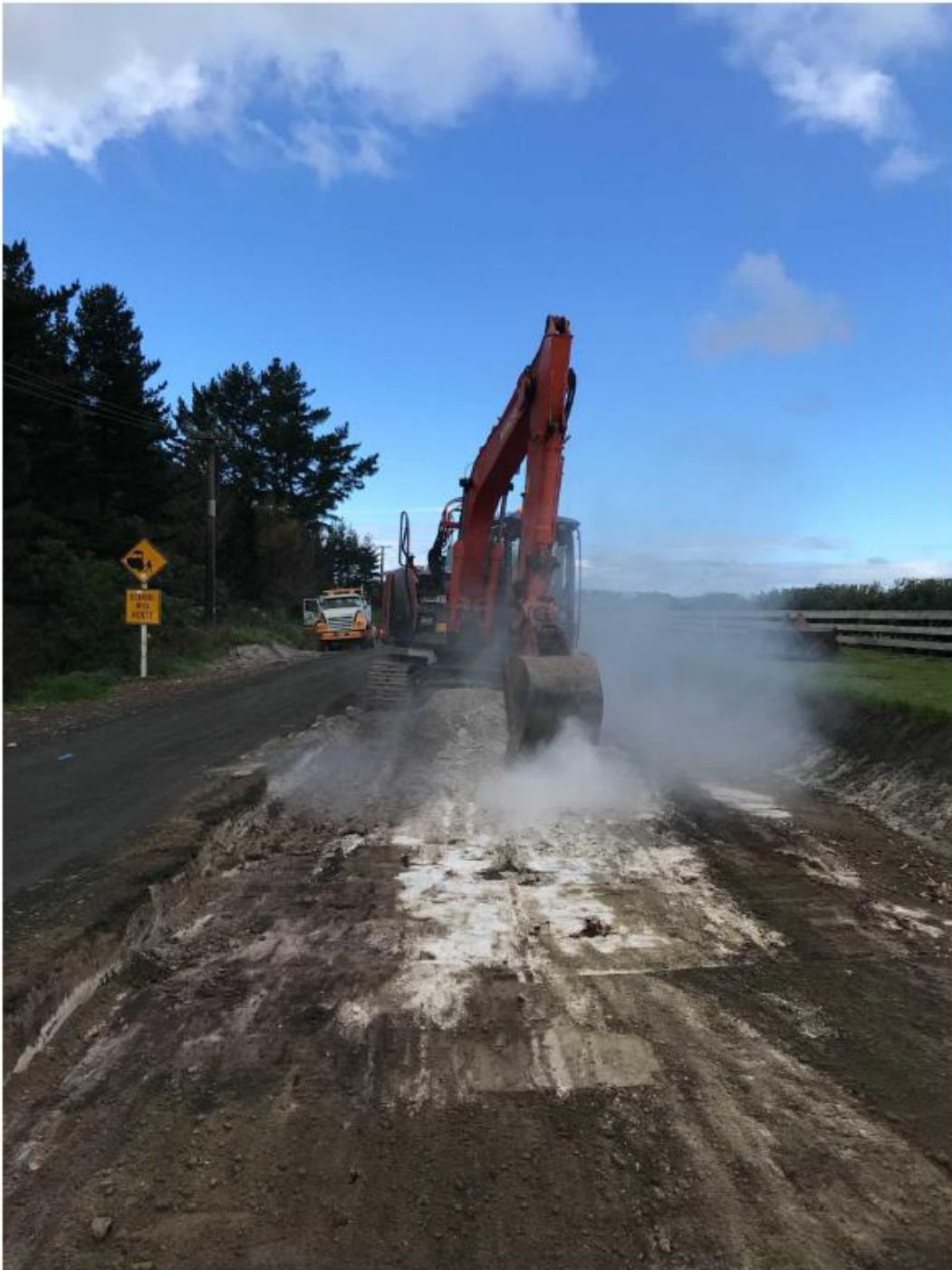
Figure 1: Pavement tie in at SH10
