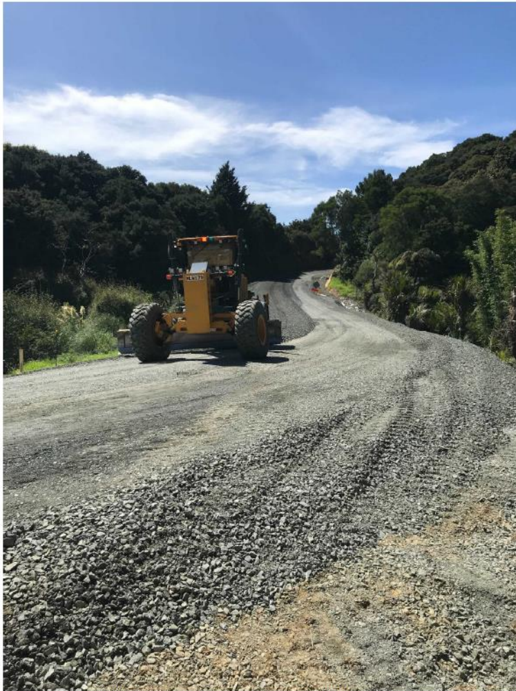
Figure 15: Section Four Overlay in progress
