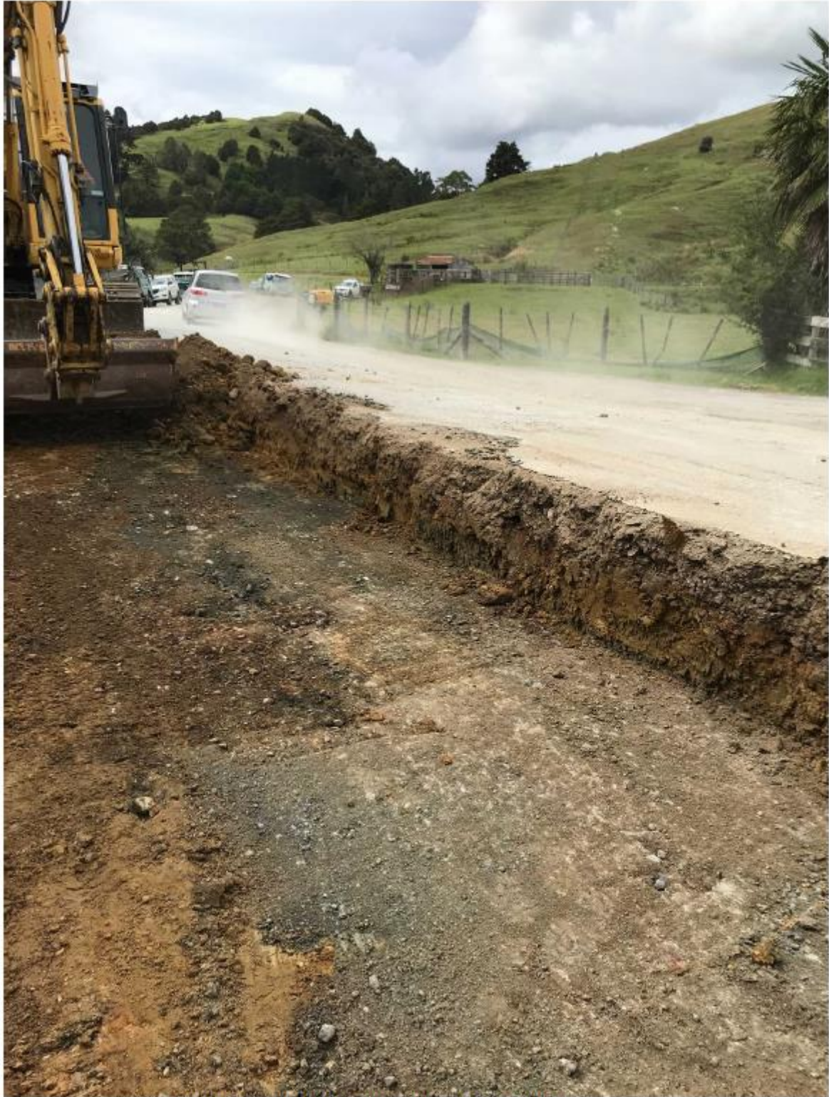
Figure 13: Section Four Bridge Undercut
