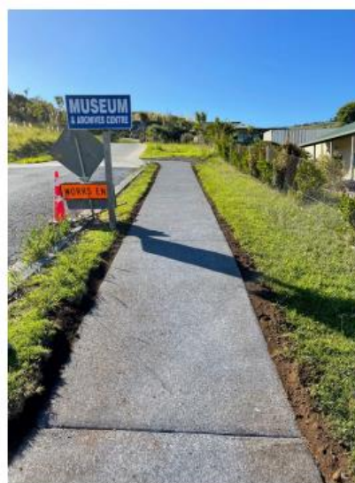
Waianga PI – Brand New Footpath
