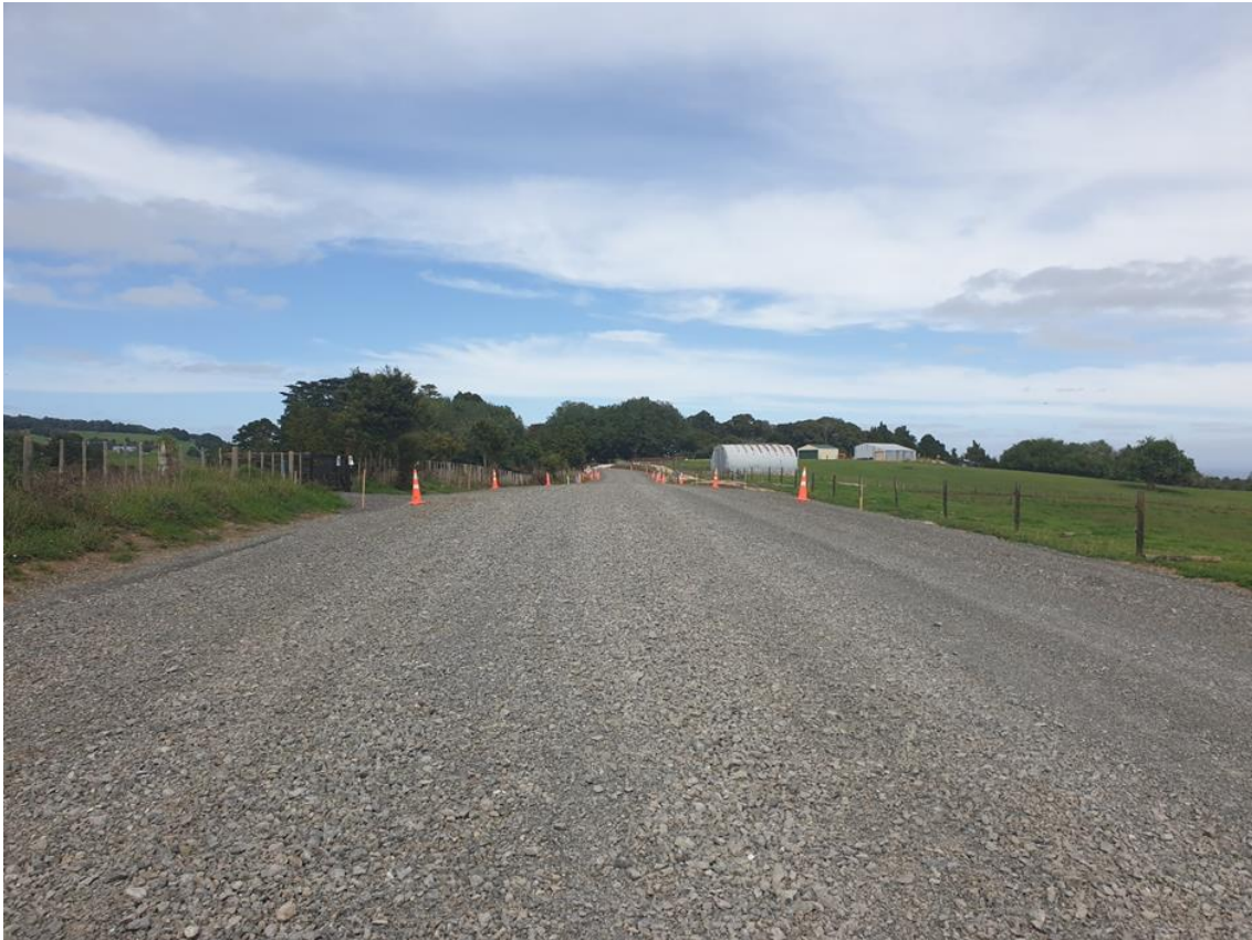
Ruapekapeka Road Stage 1 pavement construction
