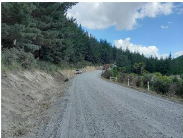
Ngapipito Rd – Enabling Works in progress
