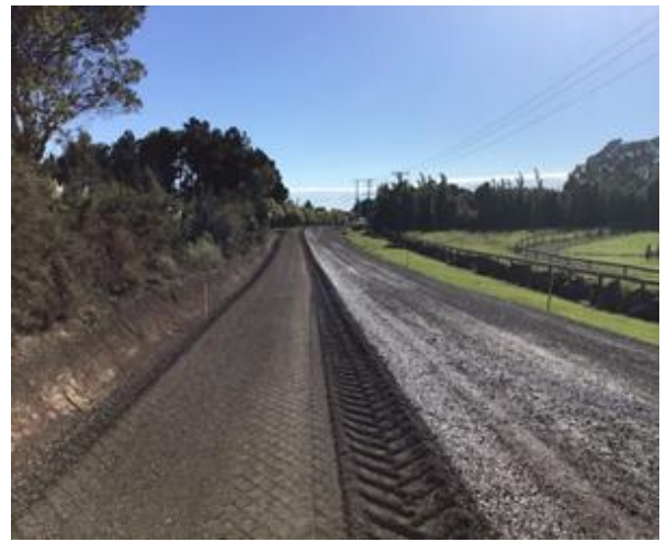
Pungaere Seal Ext. Stabilisation of first 1.4km
