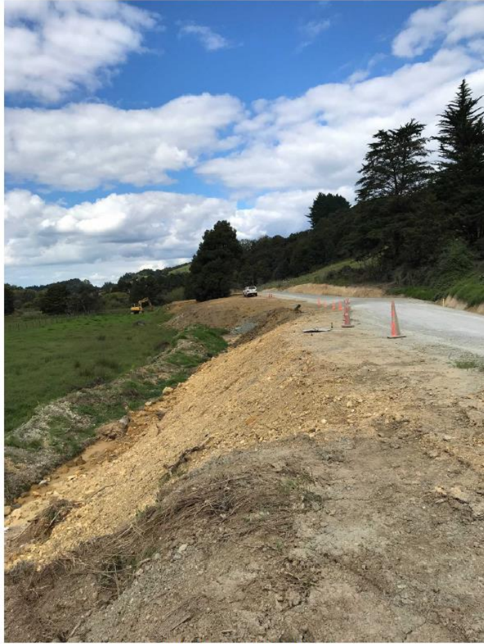
Figure 17: Section Five Tip site in progress
