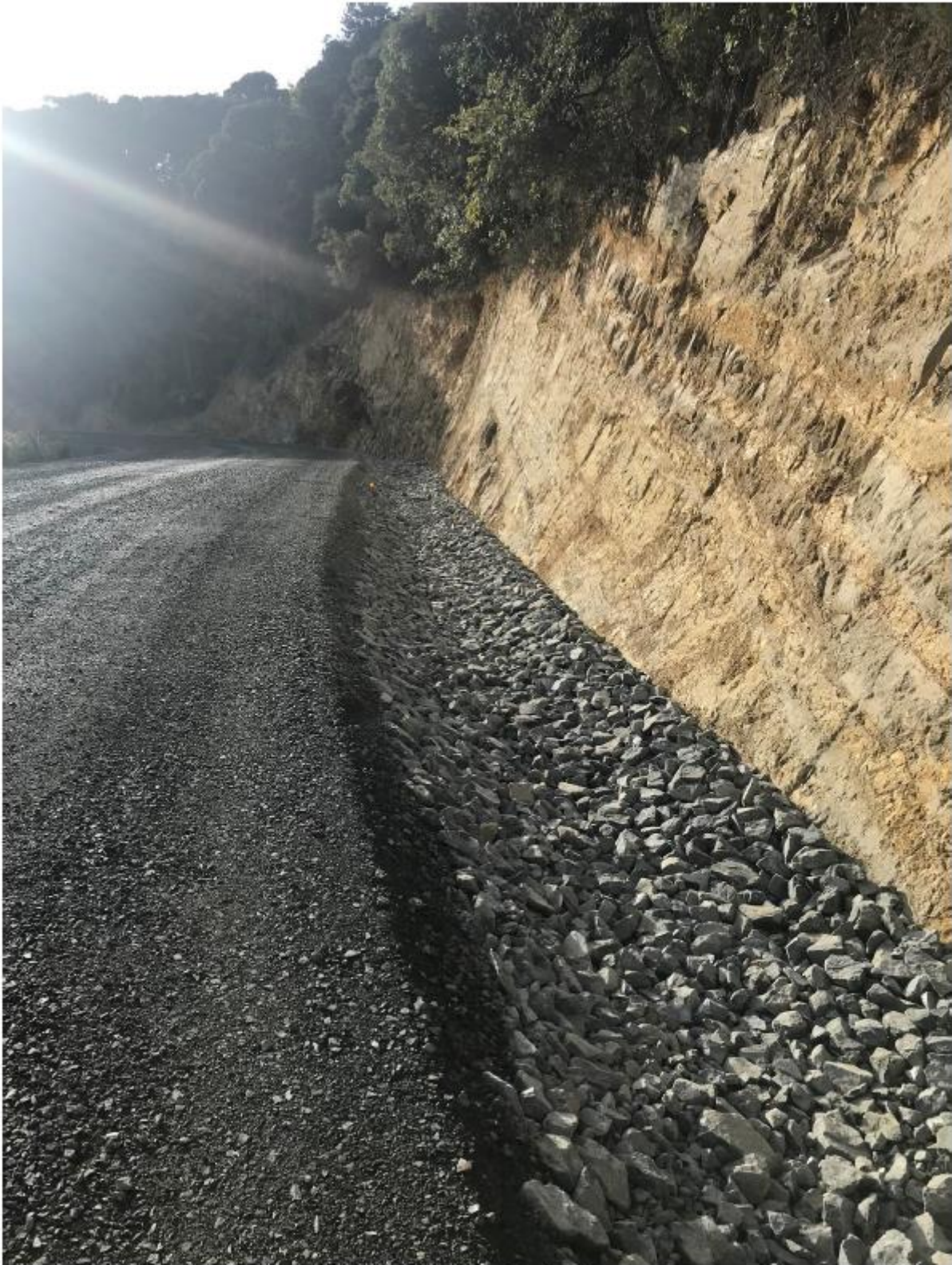
Figure 23: Section Four Scour Protection
