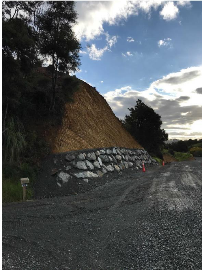
Figure 21: Section Four Rock wall construction
