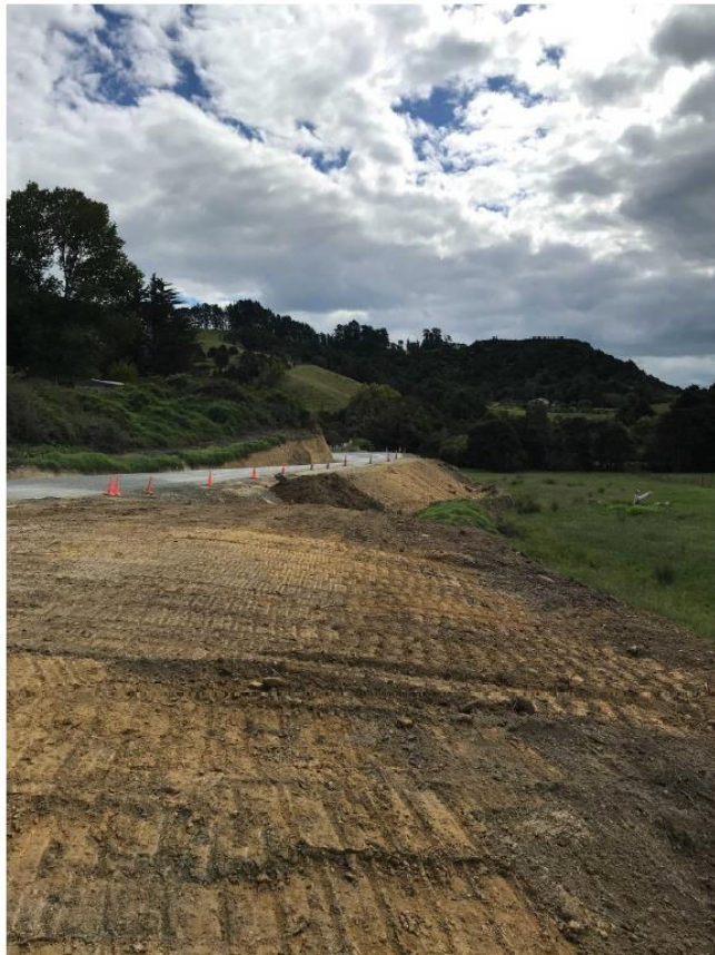
Figure 16: Section Five Tip site seal in progress
