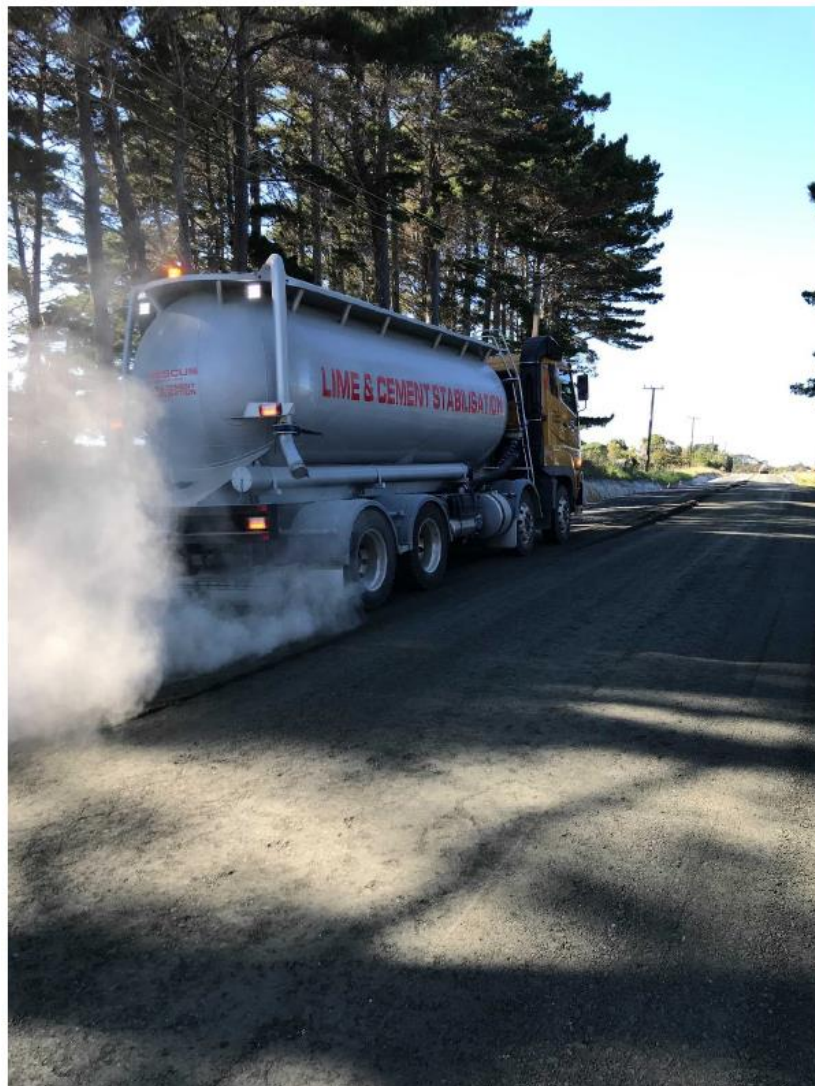
Figure 8: Section Two Stabilising in Progress
