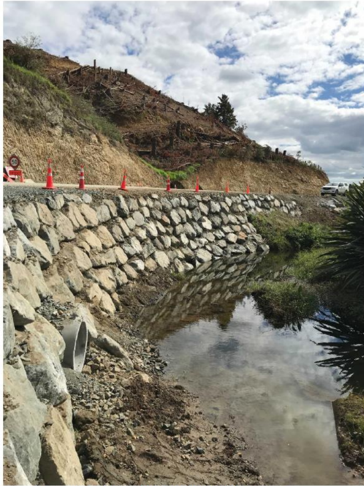
Figure 19: Section Four rock wall construction in progress
