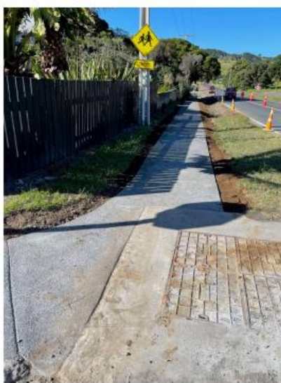
State Highway 12 (Omapere) – Footpath Replacement
