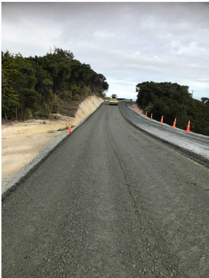
Figure 5: Section One Stabilising in progress
