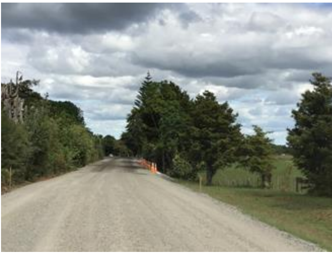
Koropewa Road/Seal Extension overlay complete pre-stabilisation
