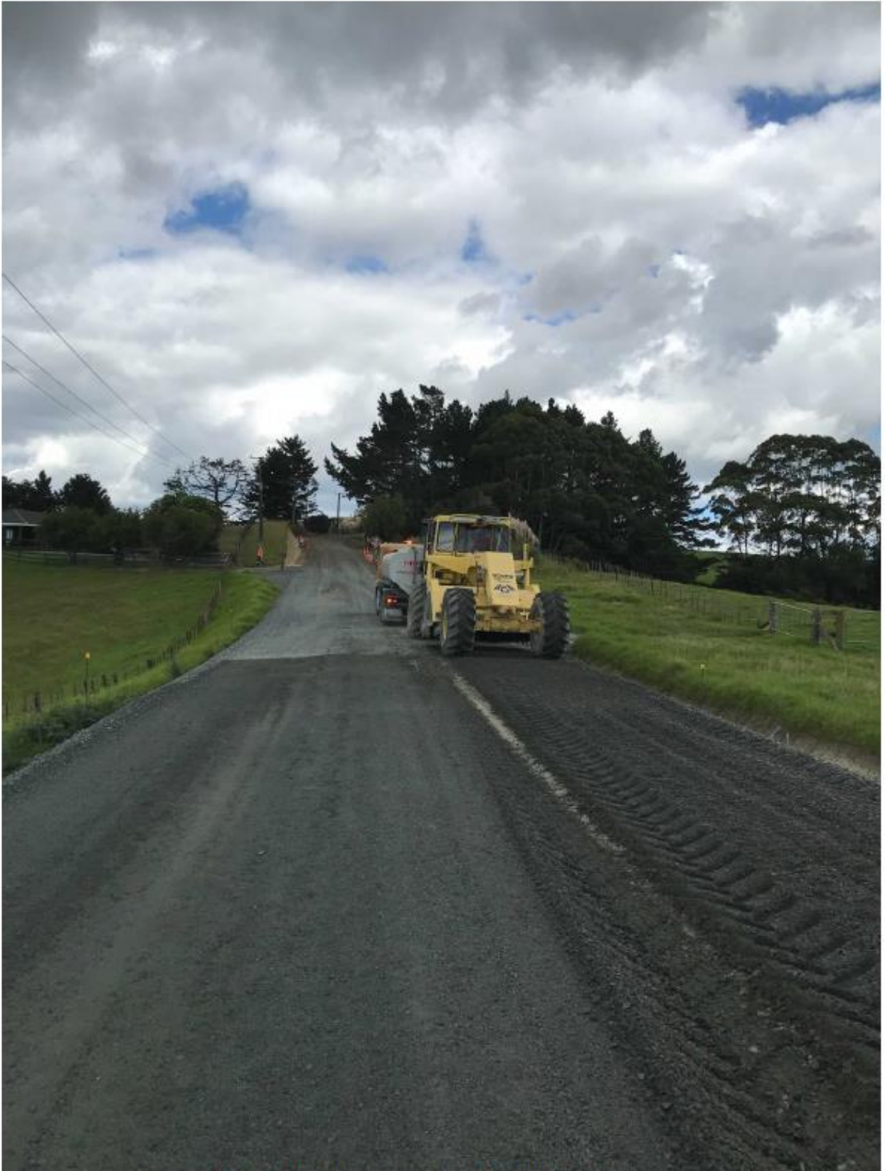
Figure 11: Section Two Stabilising in Progress
