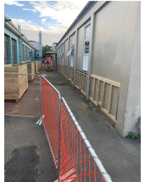
Planter boxes on the left and framing for historic photo boards in Dalmatian alleyway
