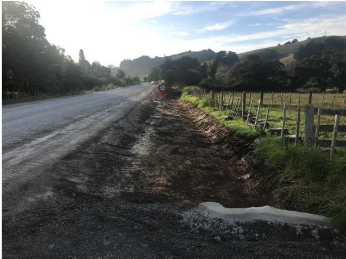
Figure 26: Section Five clearing in progress
