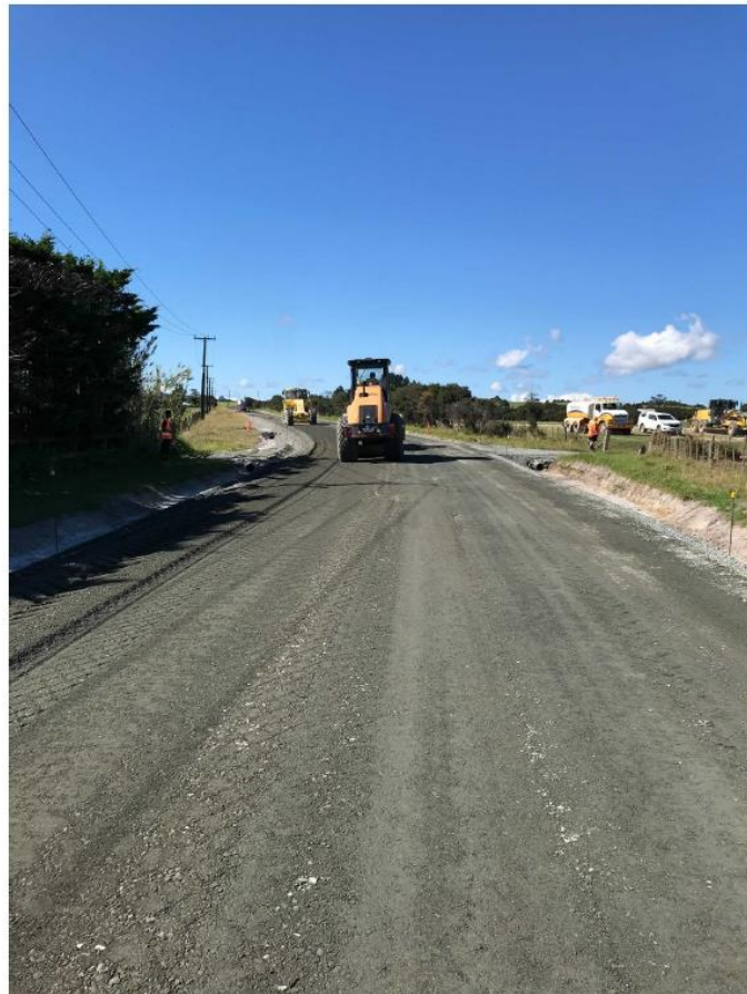
Figure 10: Section Two Stabilising in Progress
