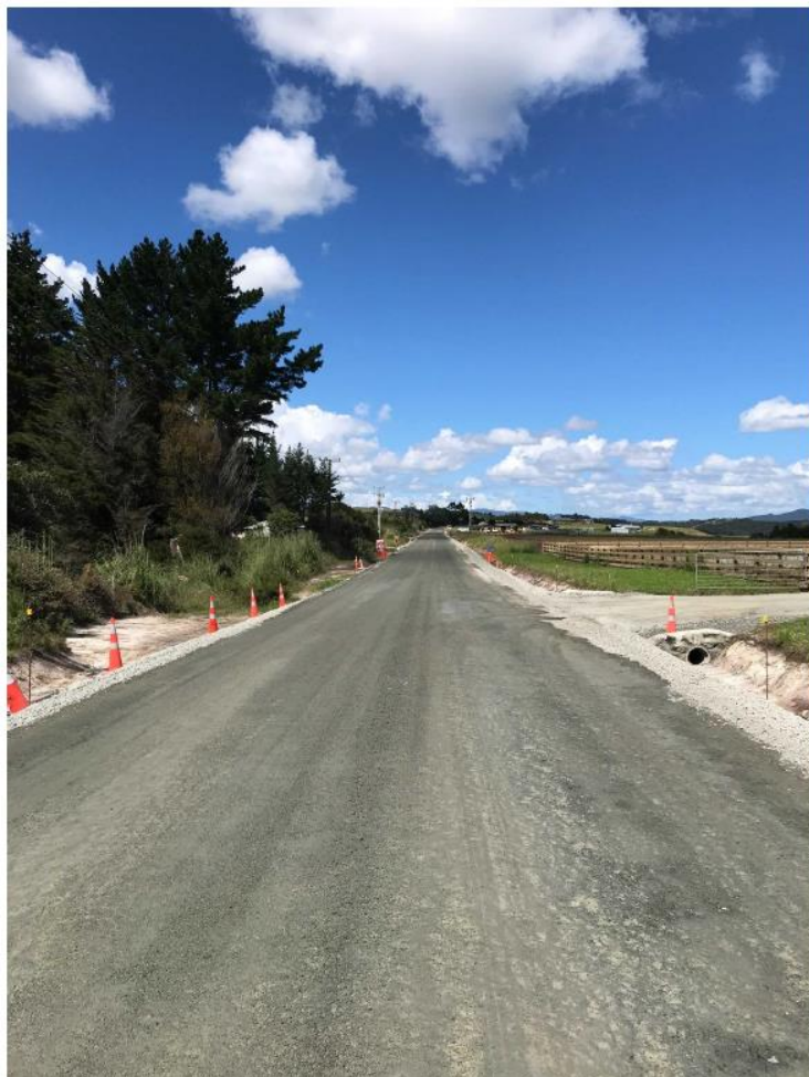
Figure 7: Section One Prepping for seal
