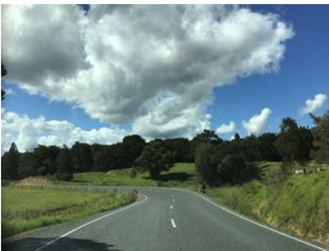
Pawarenga Site 1/ Rehab Sealed and Marked
