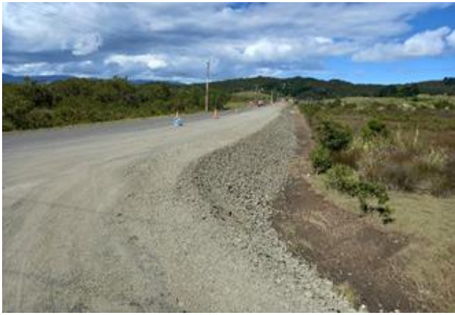
Panguru Road Flood Mitigation/Shoulder Widening
