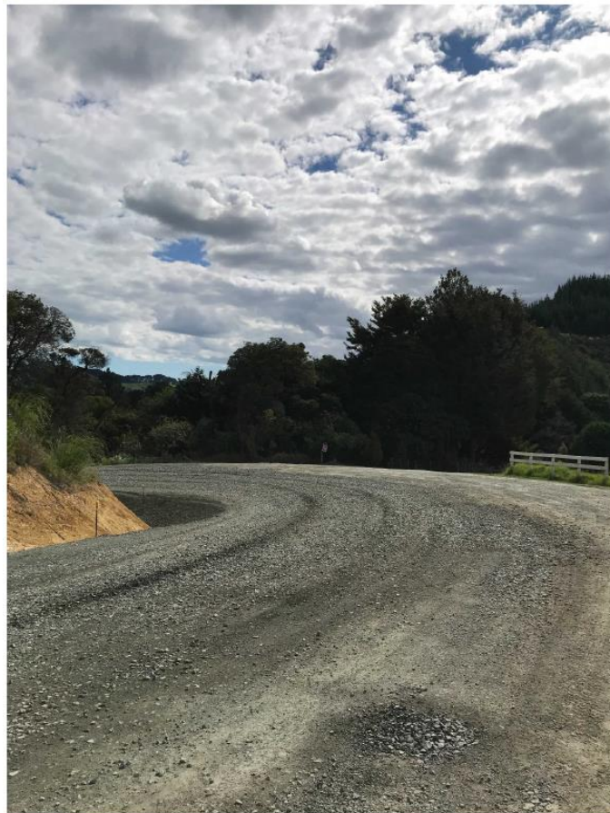
Figure 20: Section Four Overlay in Progress
