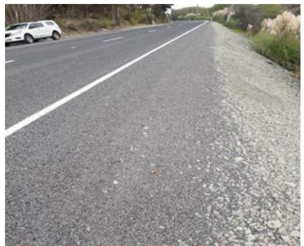
Mangamuka Road/Slip repair
