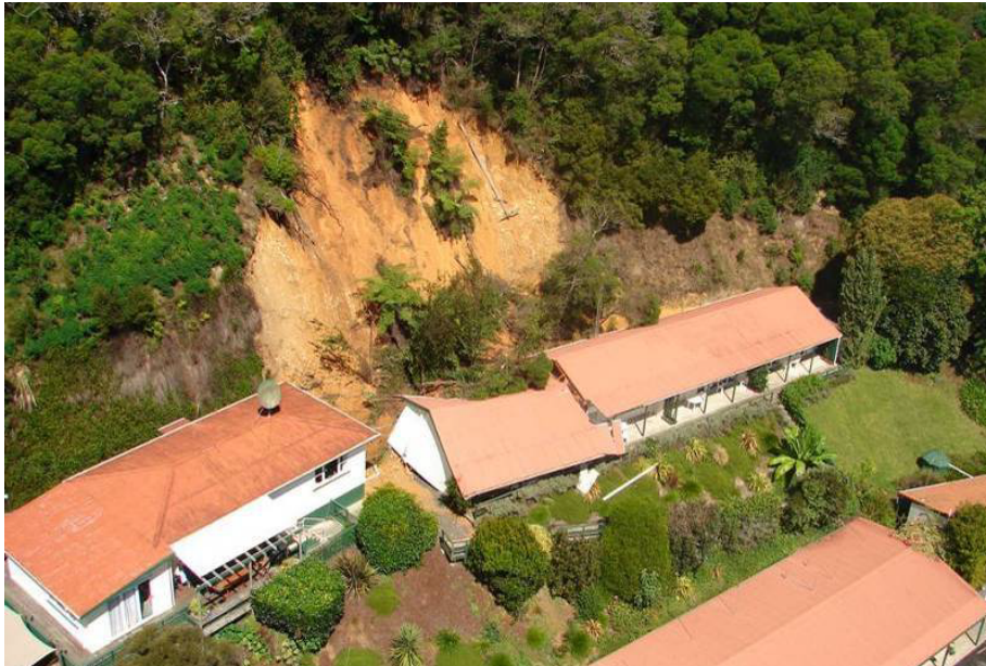
Figure 1: Landslide damage to the back of Haruru Falls Resort - 2007 (Photo FNDC)
