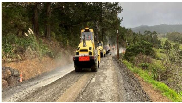
Pawarenga Road Unsubsidised Seal Extension - Stabilising
