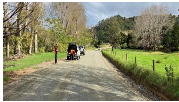
Pawarenga Road Unsubsidised Seal Extension - Pavement testing
