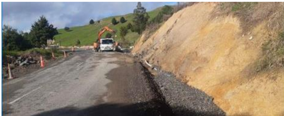
Ngapipito Road Rehabilitation - Enabling works
