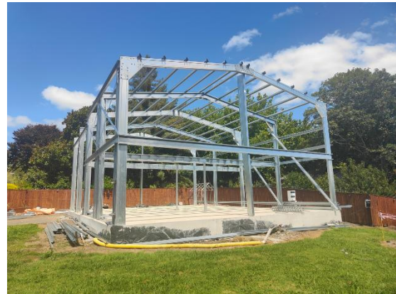
Figure 8 – Shed foundations built up 750mm
