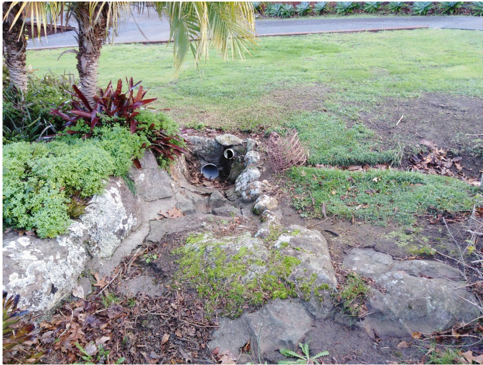
Figure 1, showing discharge pipe at base of existing rock lined basin
