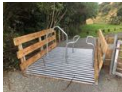
Example of a wheelchair-accessible barrier (for some wheelchairs), Belmont Regional Park (photo: Greater Wellington Regional Council)
