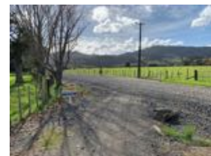
At grade crossing (low volume rural gravel road), Far North District
