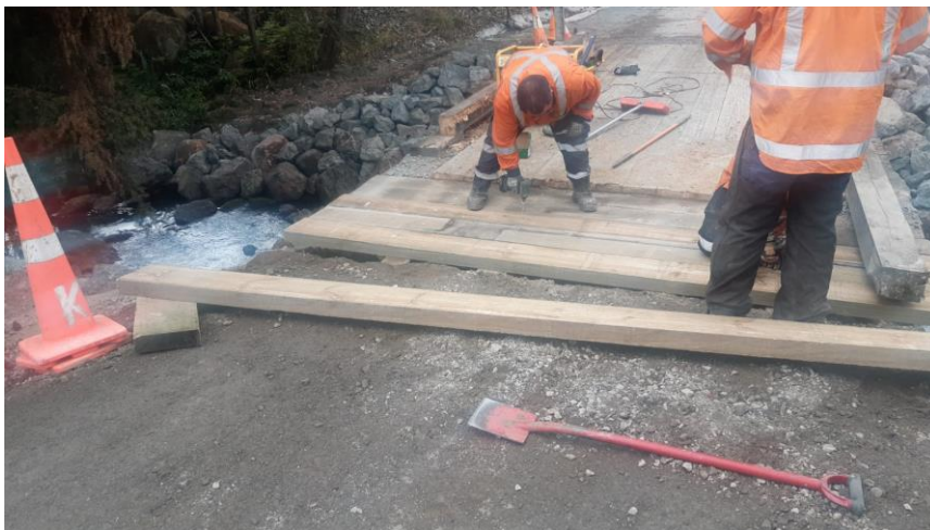
Cumber Road Bridge Repair
